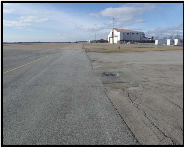
Photo 75 Building 700 (note the drains).
