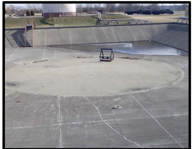
Photo 60 Tank B Dike, spray testing area.
