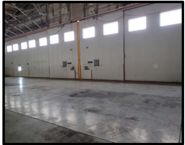
Photo 46 Interior of the hangar doors.
