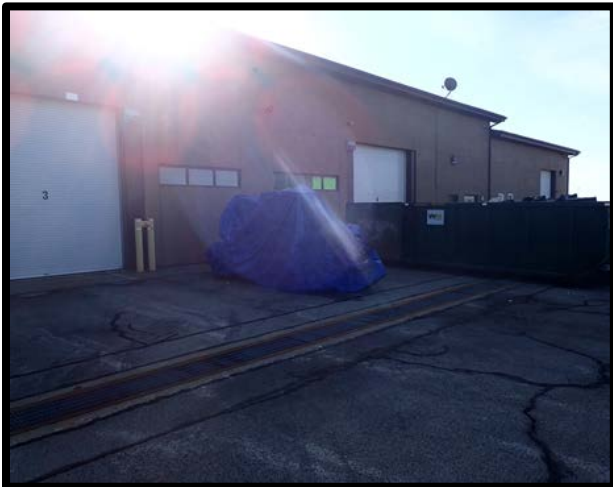
Photo 81 Building 700 (old fire station), drains not on the flight side.
