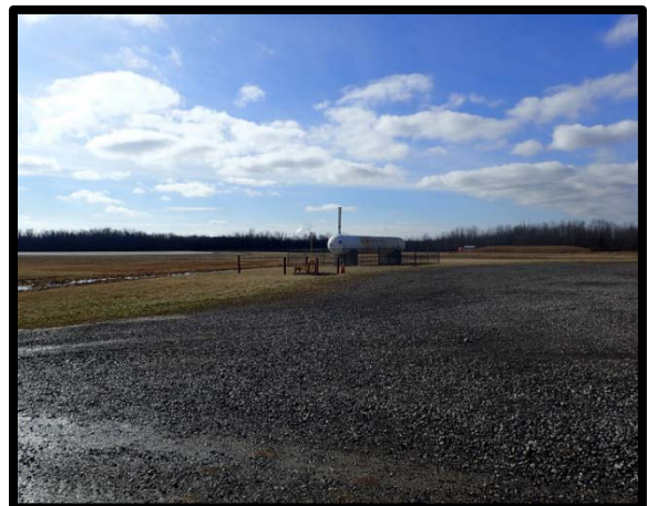
Photo 66 Propane storage for the current FTA.
