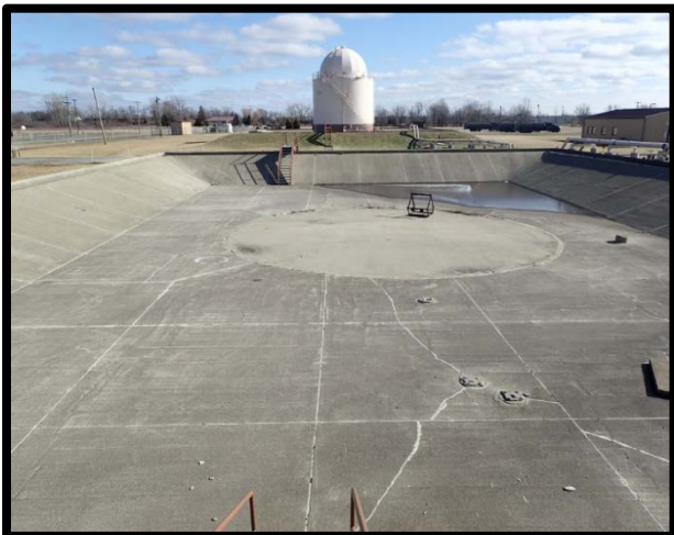
Photo 59 Tank B Dike, spray testing area.
