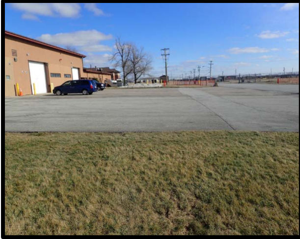
Photo 73 Building 700 (old fire station).
