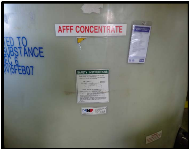
Photo 35 Building 850 AFFF tank labels.
