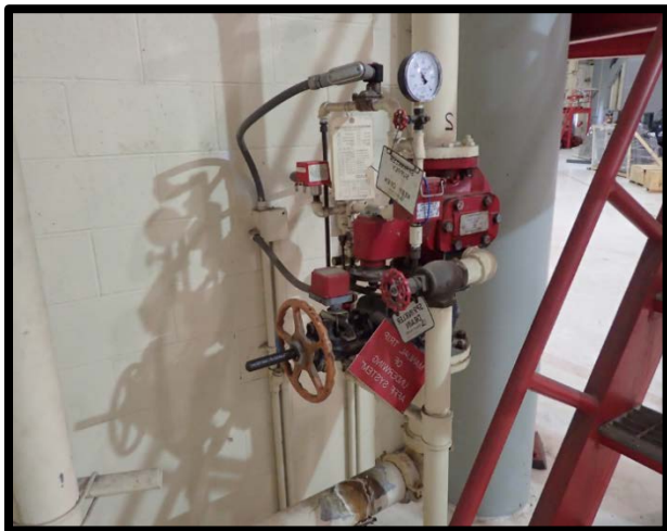
Photo 21 Underwing cannon control valve #1
