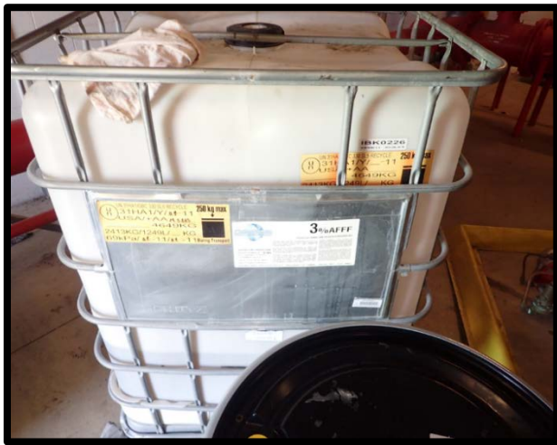
Photo 51 3 percent AFFF cubitainer at Building 707.
