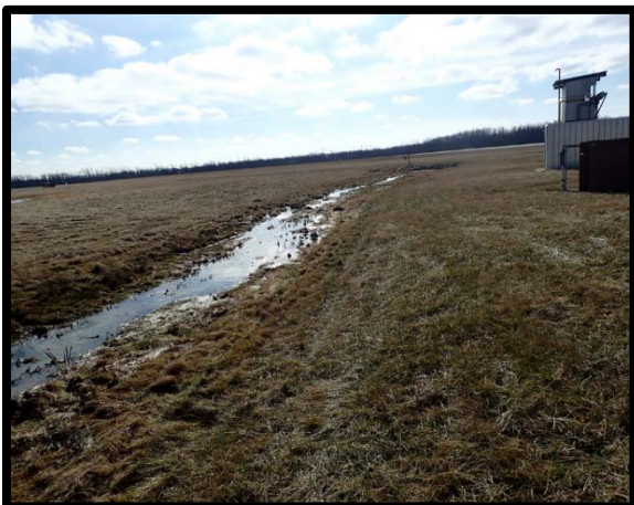
Photo 65 Northwest side of FPTA 03.
