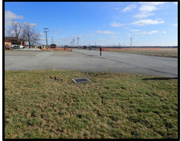
Photo 74 Building 700 (note the drains).
