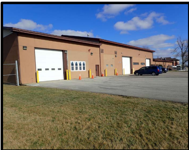
Photo 77 Building 700 (old fire station).
