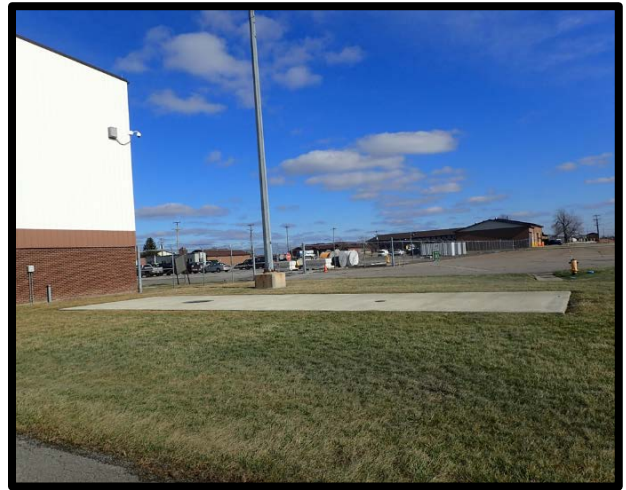
Photo 76 Building 707 holding tank.
