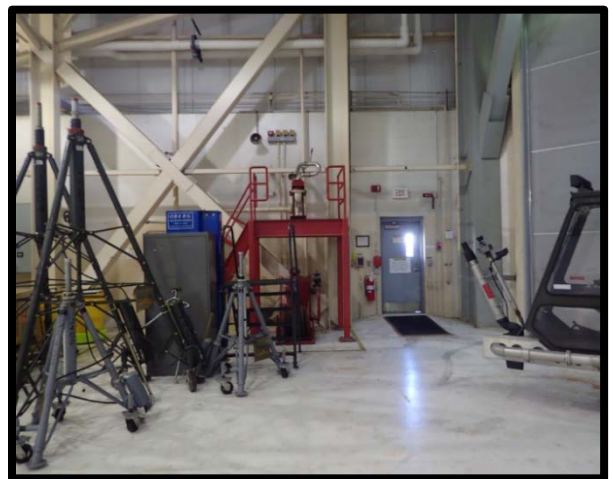
Photo 24 Building 907 underwing cannon #2.
