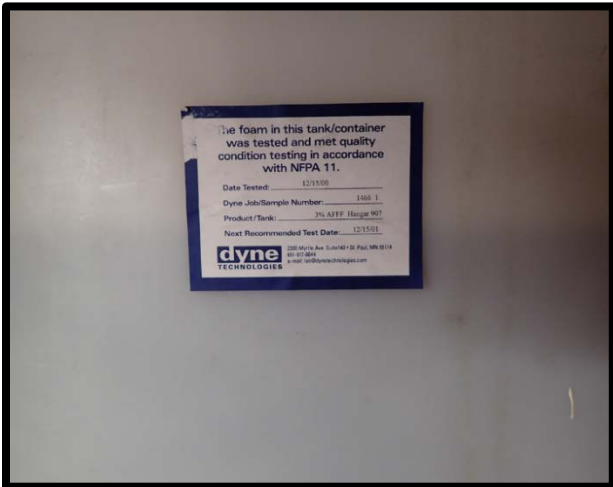
Photo 15 Building 907 AFFF tank label.
