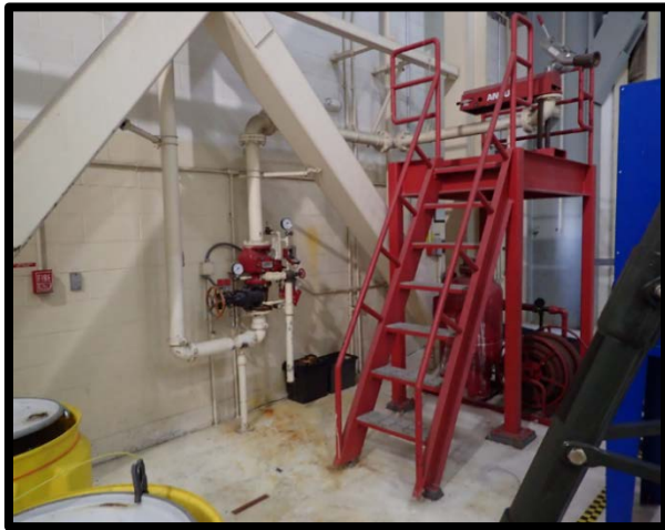
Photo 27 Building 907 underwing cannon #2.
