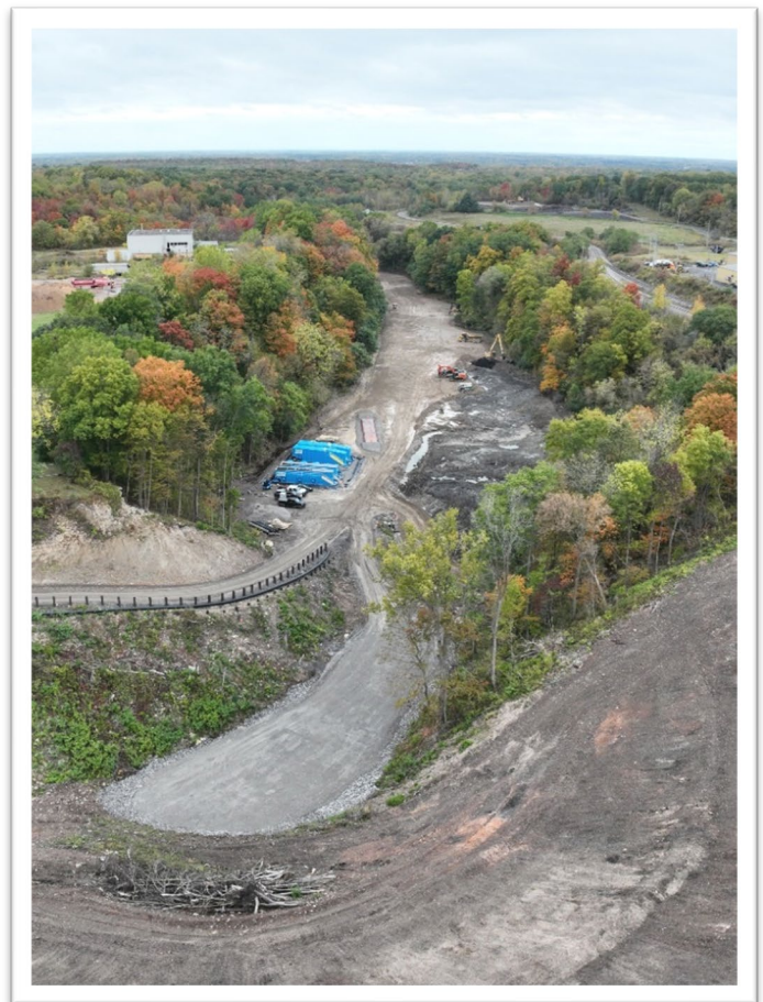
Drone imagery of the progress former dump site excavation (foreground) and Gulf Creek sediment excavation and backfilling, October 2023.
