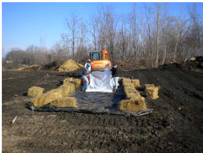
Construction of decon pad
