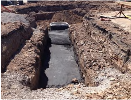
5/16/2013: MH-8 and connection to existing 42-inch diameter concrete storm line looking west
