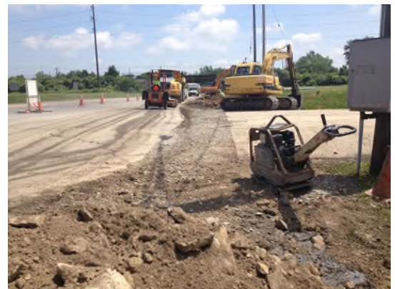
6/26/2013: Stone subbase installed in roadway cut at Road 1 looking south
