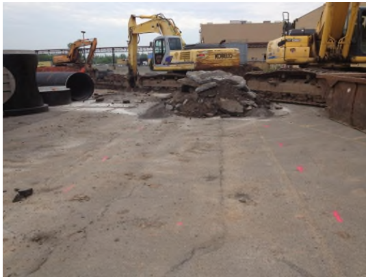
5/22/2013: Excavation markout for storm line from MH-6 to MH-5 looking south
