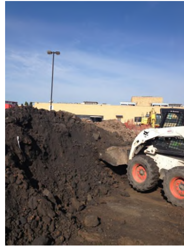
5/14/2013: Fine grain soil pile for backfill from excavation between MH-8 and MH-9 looking west
