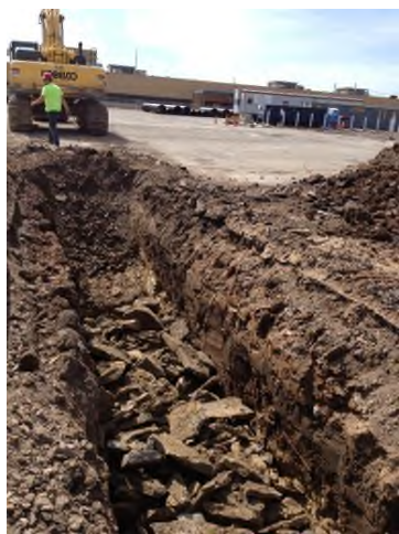
5/7/2013: Broken bedrock in excavation from MH-9 to MH-8 looking west
