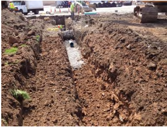
5/29/2013: Force main excavation northwest of MW-10 crossing under electrical conduit to pump station looking east
