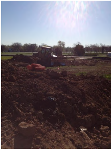
5/2/2013: Backfilling to grade near MH-13
