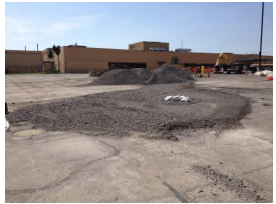
5/29/2013: Backfill around MH-7 looking northwest
