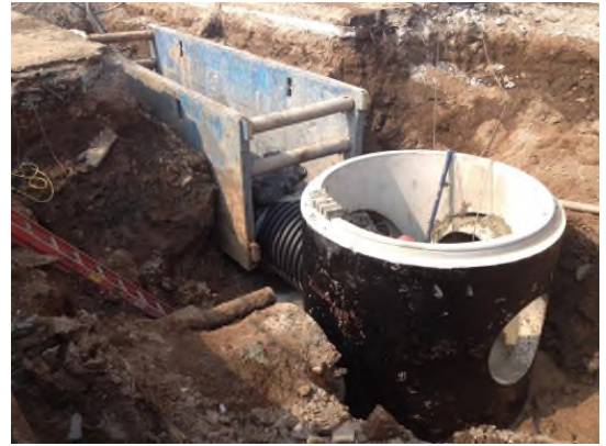
7/17/2013: Installation of MH-5 on the 48-inch GMCH storm sewer looking southwest
