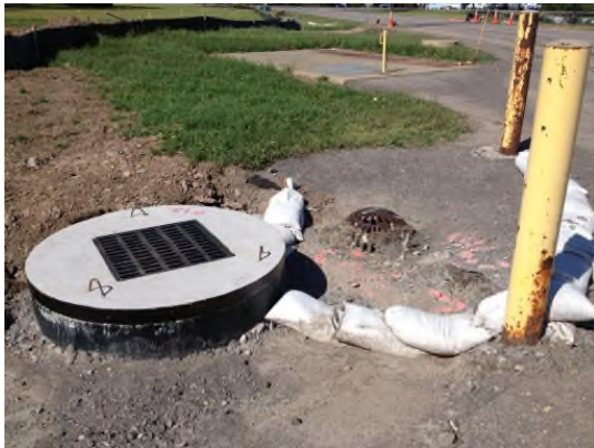
5/16/2013: New grated top for MH-12-15 looking northeast
