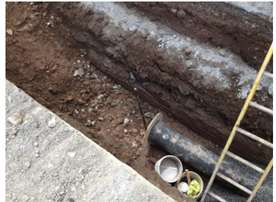
8/8/2013: Fire suppression line pipe end east of Bldg 8 looking west
