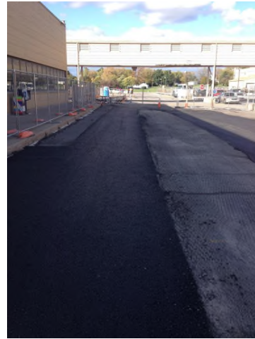
10/22/2013: Asphalt subbase placed east of Bldg 8 looking north
