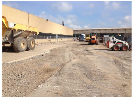
7/23/2013: New GMCH 48-inch storm sewer excavation backfilled between MH-4 and MH-5 looking north
