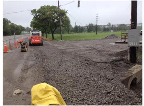
6/7/2013: Backfill of force main excavation at Road 3 and Upper Mountain Road looking south
