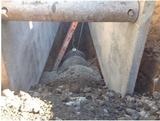
7/26/2013: 48-inch storm sewer line looking south in excavation
