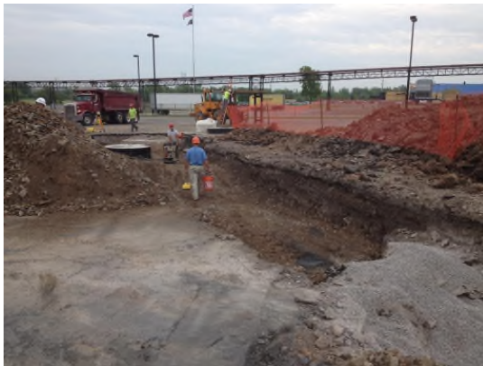
5/22/2013: Compacting backfill in vicinity of MH-7 looking southeast
