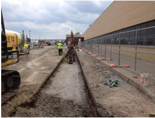
8/8/2013: Compacting backfill over fire suppression line east of Bldg 8 looking south
