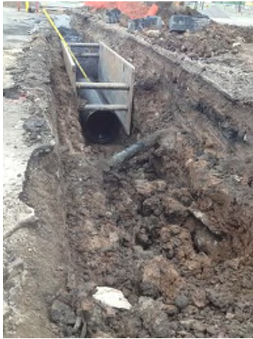
5/22/2013: 48-inch storm line and fire suppression line within excavation between MH- and MH-7 looking SE
