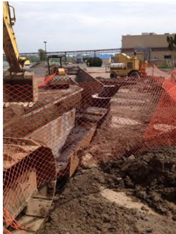
5/29/2013: Barricaded storm sewer excavation north of MH-6 looking south
