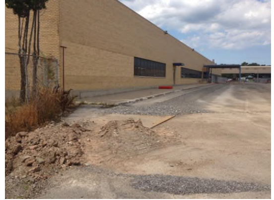
8/15/2013: Backfilled fire suppression line excavation east of Bldg 8 looking north
