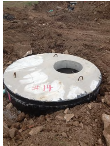
4/29/2013: Backfill around MH-14
