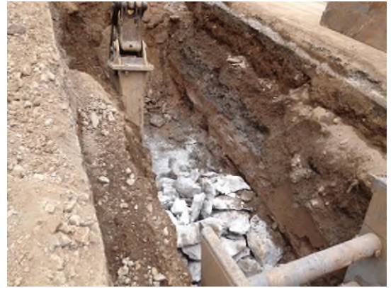
7/12/2013: Breaking bedrock for GMCH 48-inch storm sewer line looking north
