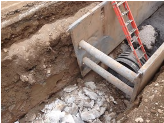
7/12/2013: Flowable fill and broken bedrock in excavation for GMCH 48-inch storm sewer line looking southeast
