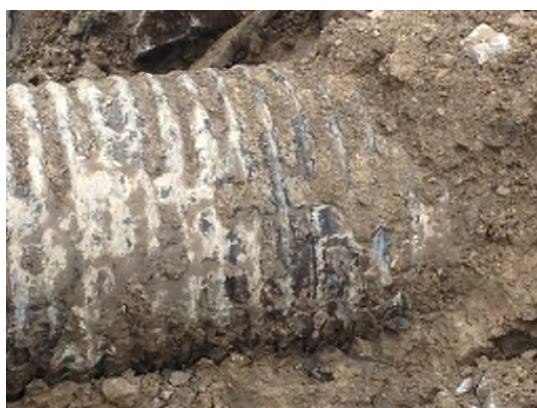
7/1/2013: Sand, gravel & fractured bedrock backfill around GMCH sanitary sewer line
