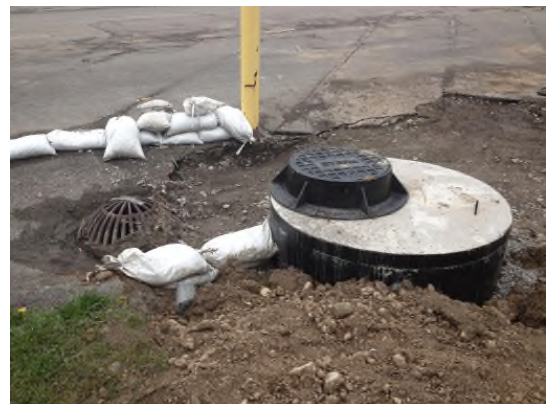
4/29/2013: Elevation difference from MH-12-15 and existing to be abandoned
