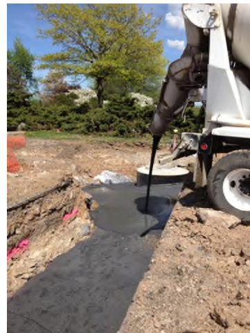
5/7/2013: Flowable fill placement around MH-9 looking east
