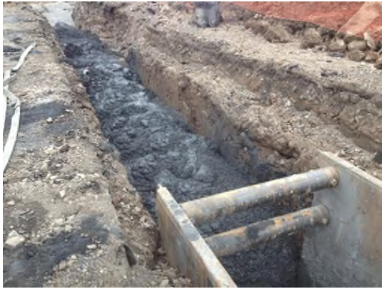
5/22/2013: Flowable fill backfill between MH-6 and MH-7 looking south
