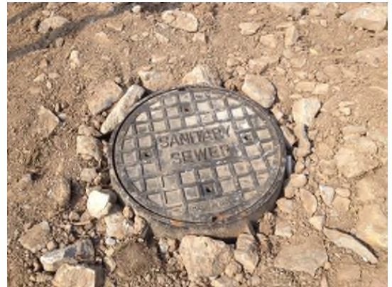
7/17/2013: Sanitary sewer cover placed on MH-1 on force main
