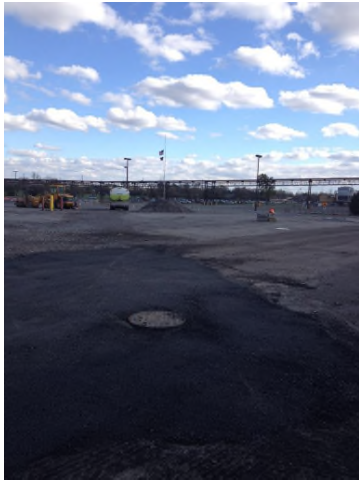
10/22/2013: Asphalt subbase around new GMCH MH-6 looking east
