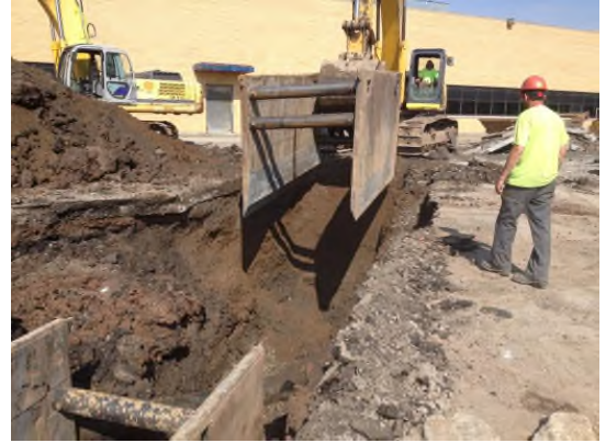
5/22/2013: Placement of trench box in excavation in vicinity of MH-6 looking northwest
