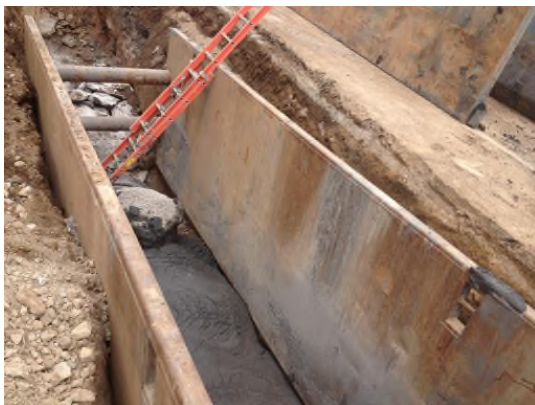
7/12/2013: Trench box and flowable fill in GMCH 48-inch storm sewer excavation looking north
