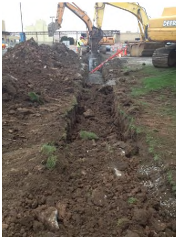
4/29/2013: MH-12-15 to CB-12 looking west – backfill and stone placement
