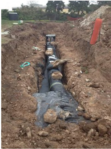
4/29/2013: Flowable fill around pipe from MH-14 to MH-13 looking northeast
