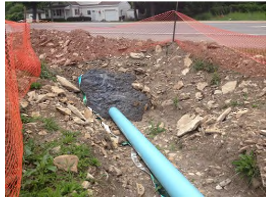
7/12/2013: Flowable fill around force main at Upper Mountain Road near on-site stream crossing looking east
