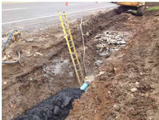
7/1/2013: Force main installation south of Road 1 looking southeast
