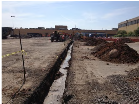
5/29/2013: Electrical conduit trench from pole to new substation south of Bldg 6 looking west
