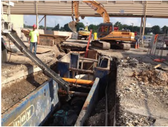
7/23/2013: Flowable fill placement south of MH-4 looking north
