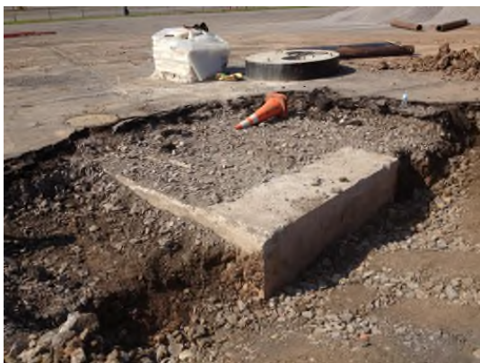
5/22/2013: Existing storm structure MH-A that was tied into with 48-inch storm line looking southwest
