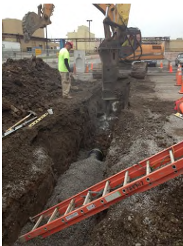
4/29/2013: Breaking bedrock near CB-12 looking west
