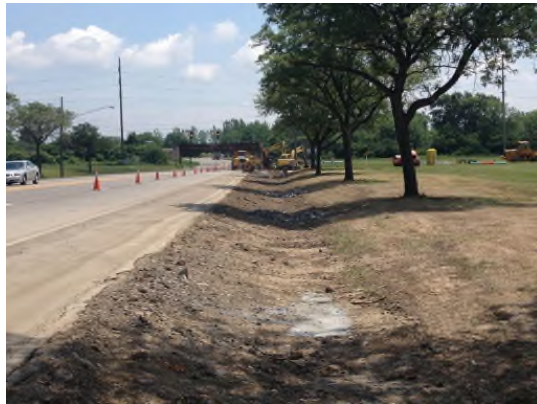
6/26/2013: Force main backfill and swale south of Road 1 looking south
