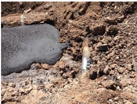
5/16/2013: Fire suppression line encountered and repaired during work near MH-8 looking west
