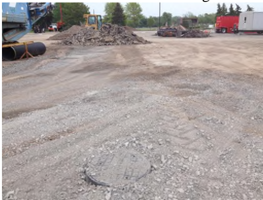
5/22/2013: Backfill around MH-8 looking east
