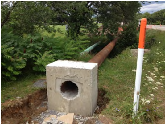
7/29/2013: Concrete form and steel pipe for creek crossing along Upper Mountain Rd. looking north
