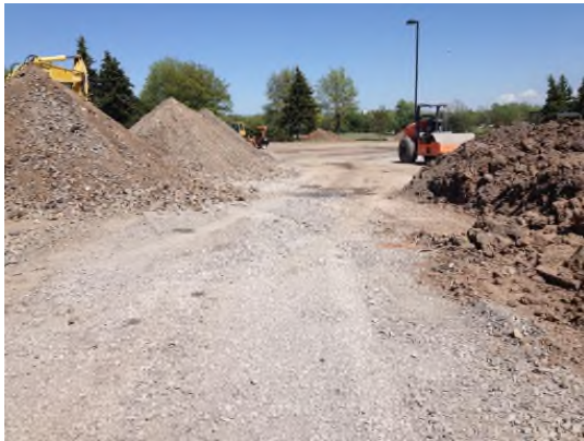
5/16/2013: Crushed concrete and backfilled storm line from MH-8 towards MH-9 looking east
