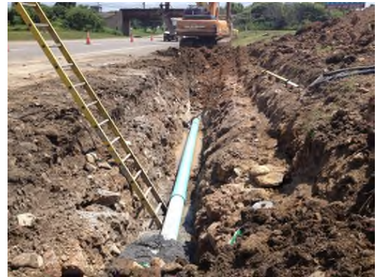
6/26/2013: Force main installation, flowable fill and soil removal in excavation at Upper Mountain Rd. south of Road 1 looking south
