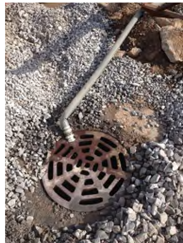
5/14/2013: Water divert form MH-B during tie-in
