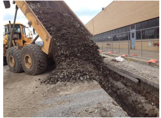
8/8/2013: Placing crushed concrete and bedrock in fire suppression excavation east of Bldg 8 looking south
