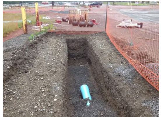
6/7/2013: Force main pipe to be tied into lift station looking south
