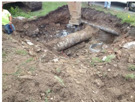
7/1/2013: GMCH sanitary sewer line and gas line exposed along Upper Mountain Rd. looking east
