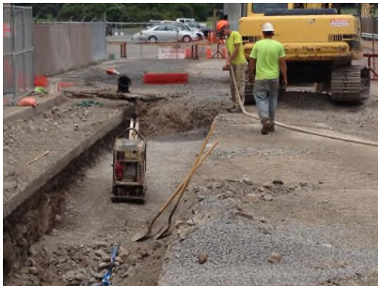
8/8/2013: Placing water on stone backfill over fire suppression line excavation to help with compaction requirements looking north
