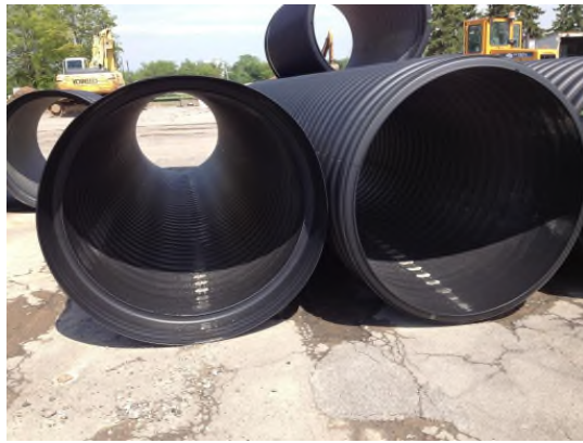
5/29/2013: 48-inch storm piping in storage area
