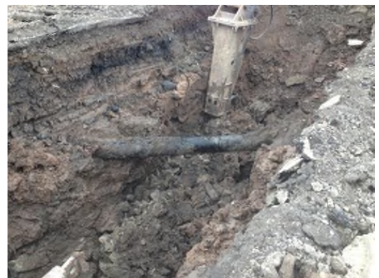
5/22/2013: Fire suppression line encountered in excavation between MH-7 and MH-6 looking west
