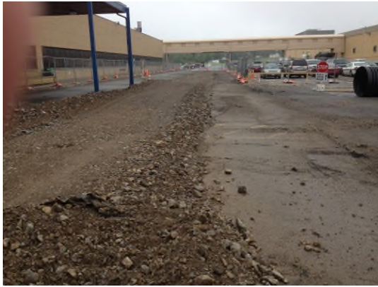
6/7/2013: Asphalt and concrete removed and replaced with crushed bedrock to prevent ponding looking north
