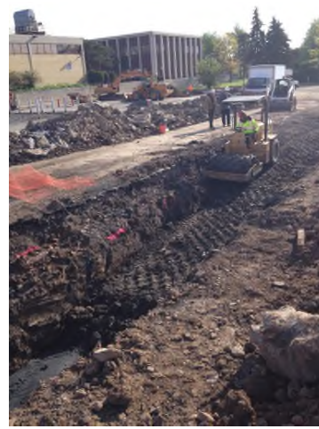
5/14/2013: Compacting fine grained soil east of MH-8 looking northeast
