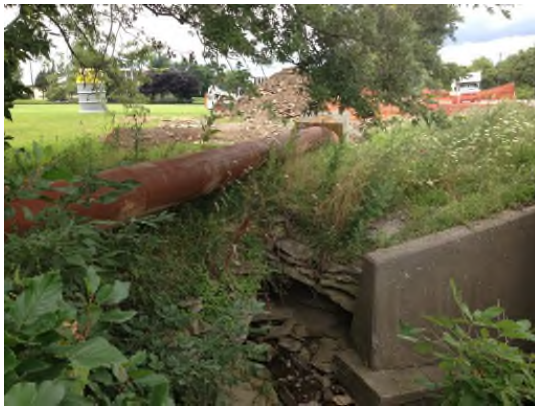
7/29/2013: Steel pipe for force main crossing of creek in place looking north
