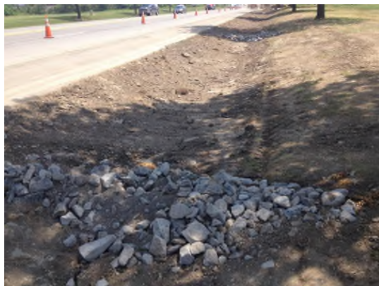
6/26/2013: Sediment traps installed in swale along Upper Mountain Rd. south of Road 1 looking south
