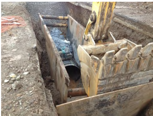
6/7/2013: New GMCH 48-inch pipe between MH-5 and MH-6 looking south
