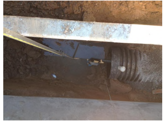
7/26/2013: 48-inch storm line within excavation
