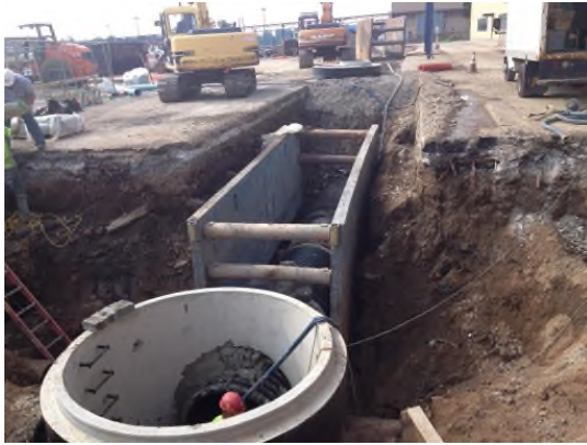
7/17/2013: 48-inch pipe, backfill and trench box south of MH-5 looking south
