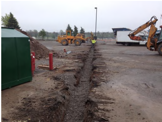
6/7/2013: Backfilling electrical conduit for light pole looking south
