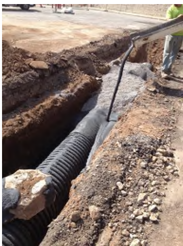
5/7/2013: Flowable fill placement north of MH-10 looking northwest
