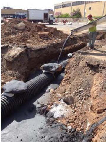
5/7/2013: Flowable fill placement north of MH-10
