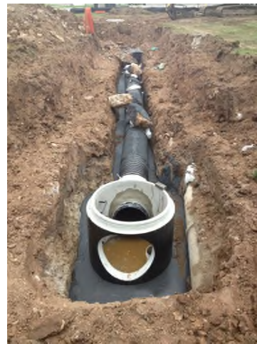
4/29/2013: MH-13 and pipe to MH-14 with flowable fill around pipe looking southeast
