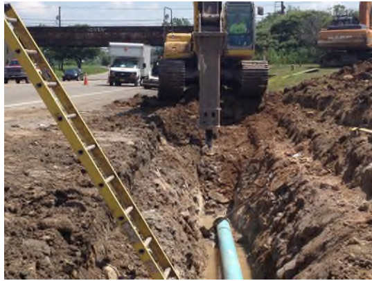
6/26/2013: Breaking bedrock south of Road 1
