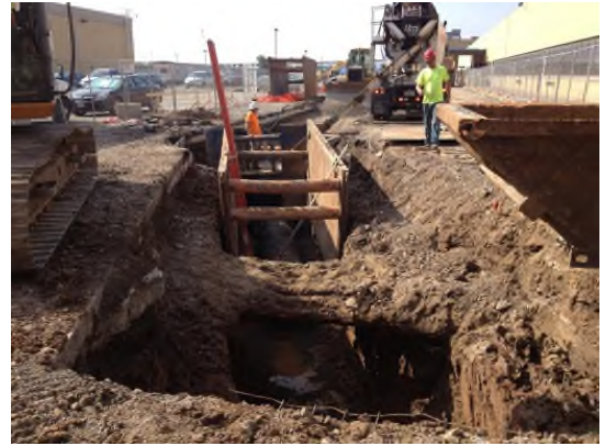
7/23/2013: GMCH 48-inch storm sewer installation north of MH-4 looking south
