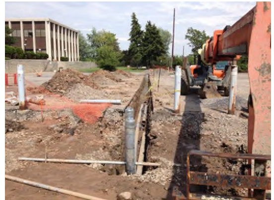
5/29/2013: Electrical conduit trench to new substation form power pole south of Bldg 6 looking east
