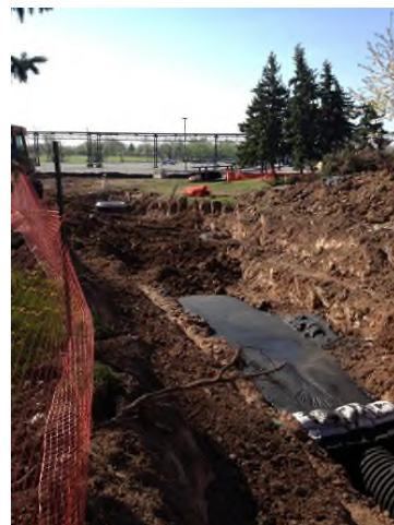
5/2/2013: Backfill around pipe from MH-13 to MH-9
