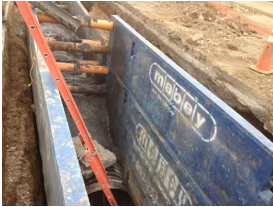
7/9/2013: Flowable fill placement around GMCH new 48-inch storm sewer line looking south
