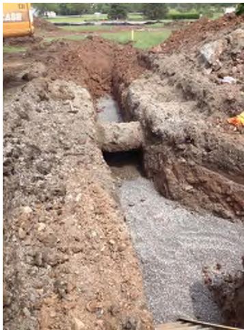
5/29/2013: Force main excavation northwest of MW-10 crossing under electrical conduit to pump station looking east
