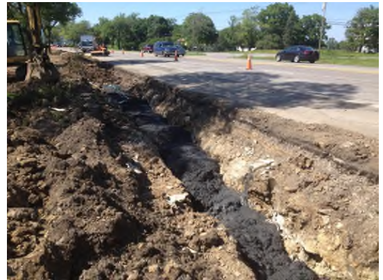
6/18/2013: Flowable fill backfill in excavation along Upper Mountain Road between Roads 2 & 3 looking north
