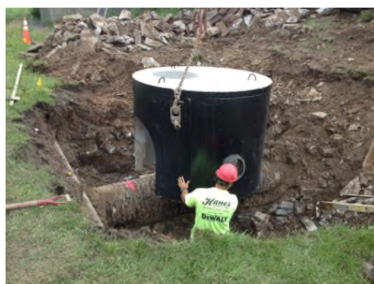
7/1/2013: Placing sanitary MH-1 over GMCH sanitary line south of Road 1 looking south
