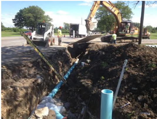
6/18/2013: Covering force main excavation with plates, end of work day, looking south near Road 2
