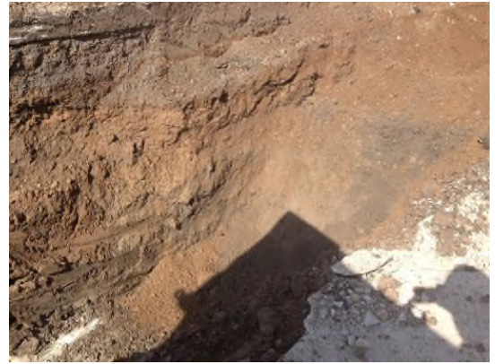
5/22/2013: Gravel layer encountered near location of MH-6 looking west
