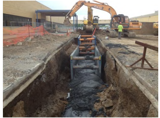
7/9/2013: New GMCH 48-inch storm sewer line excavation looking north
