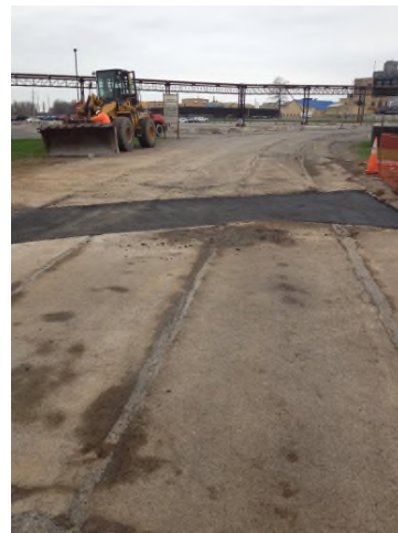
4/24/2013: Road 3 Cut Asphalt Repair
