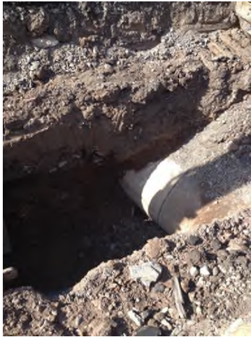
5/14/2013: Existing 48" concrete storm sewer in vicinity of MH-8 looking SW
