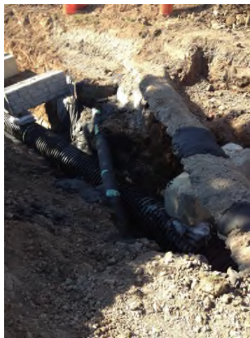
5/2/2013: Utility lines encountered south of MH-9
