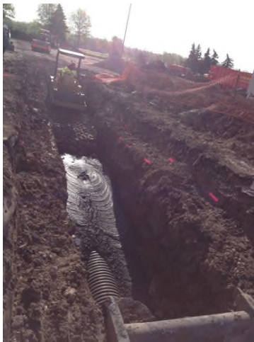
5/14/2013: Compacting fine grained soil east of MH-8 looking east
