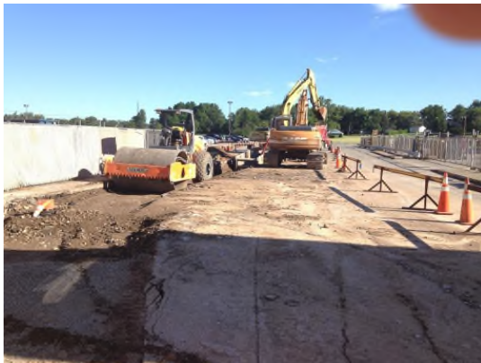
7/26/2013: Storm sewer excavation backfilled north of MH-3 and 4 looking north
