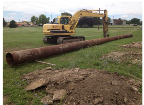
7/12/2013: Welded steel pipe to be used for on-site stream crossing for force main pipe looking north
