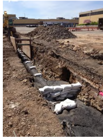
5/7/2013: Excavation, backfill and pipe from MH-9 to MH-8 looking west
