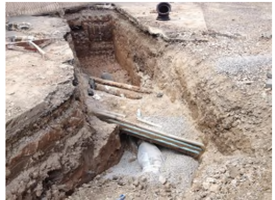
8/8/2013: Start of fire suppression line excavation near pedestrian bridge east of Bldg 8 looking northwest
