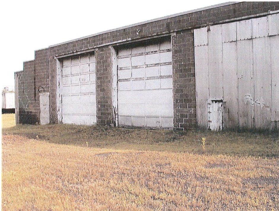
Photograph No. 4 West side of Building, facing north
