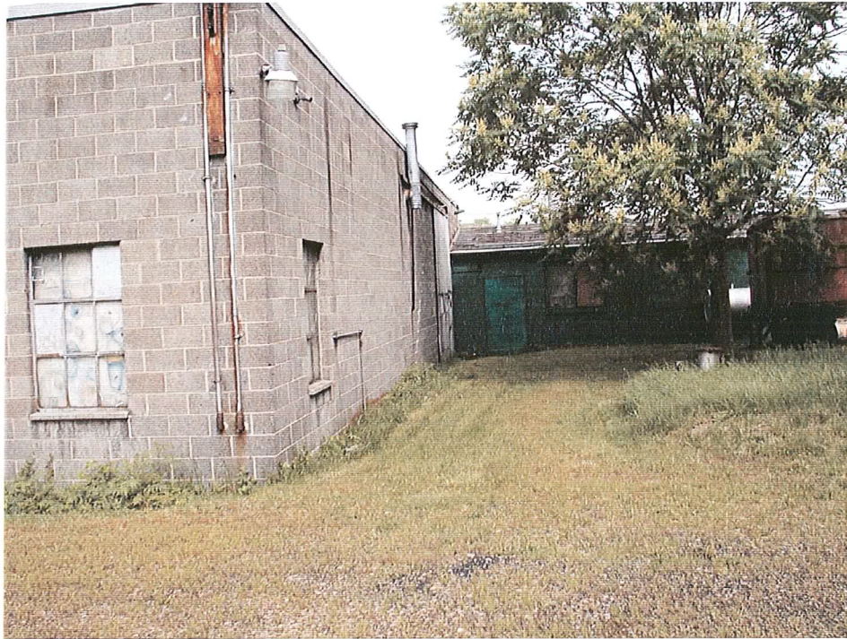
Photograph No. 5 South side of Building, facing northwest
