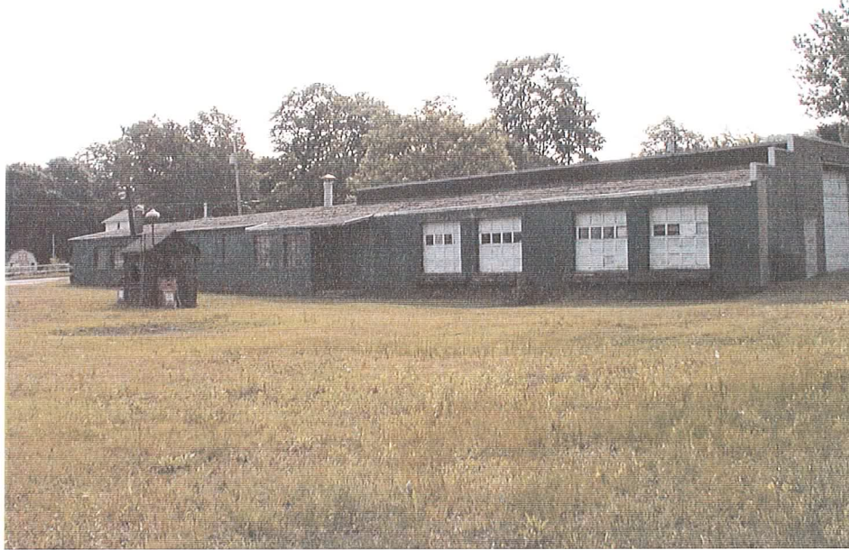
Photograph No. 3 North side of Building, facing east
