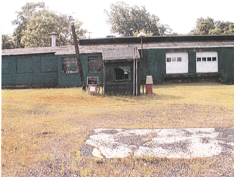
Photograph No. 2 North side of Building, facing southeast, note concrete pad, pump house and fuel dispensers
