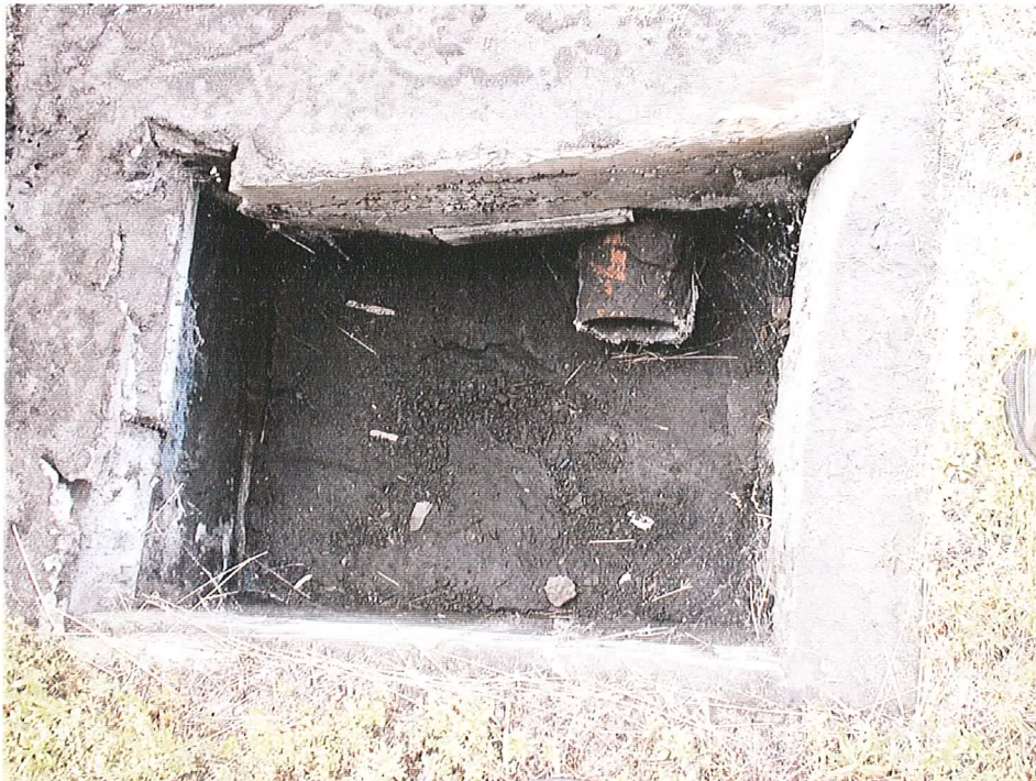
Photograph No. 8 Sediment trap, located along the west side of the building
