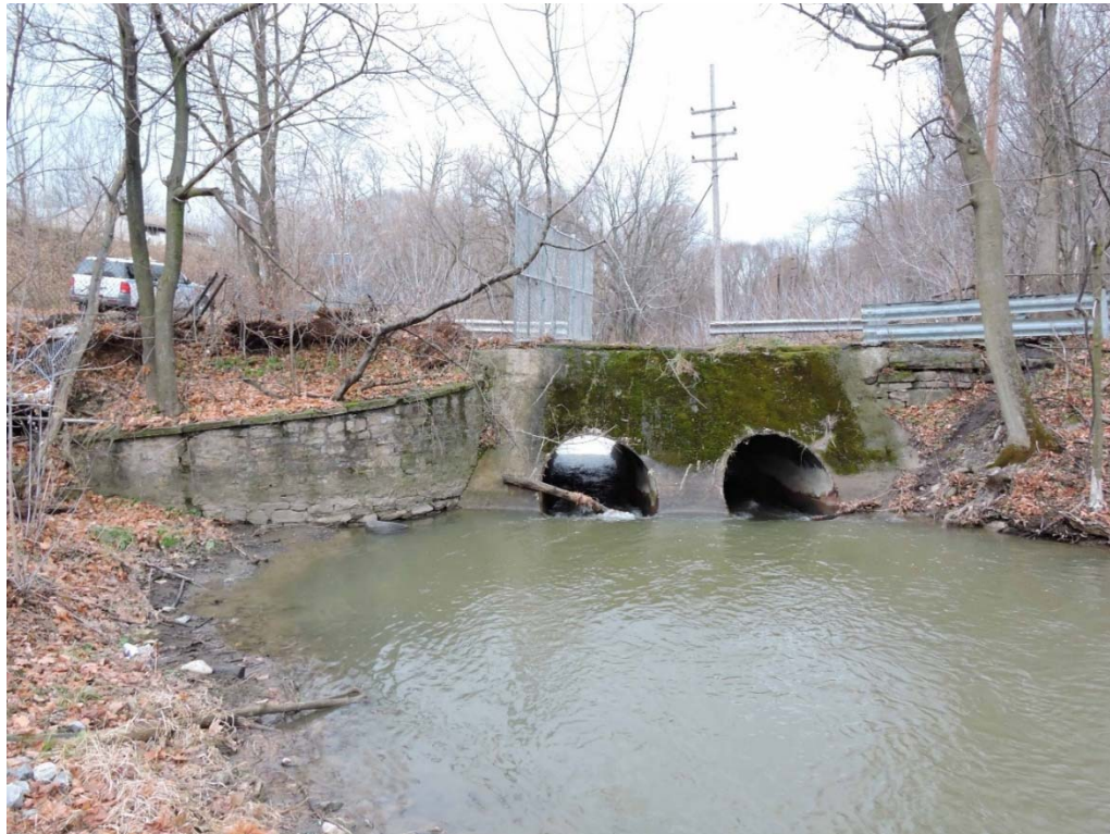
Photo 2. View facing northwest of the double culvert and associated wingwalls beneath William Street at the north end of the OU1 APE. The eastern wingwall composed of dry-laid stone is likely a remnant of an earlier bridge/dam. The double culvert is just outside of the OU1 APE to the north.
