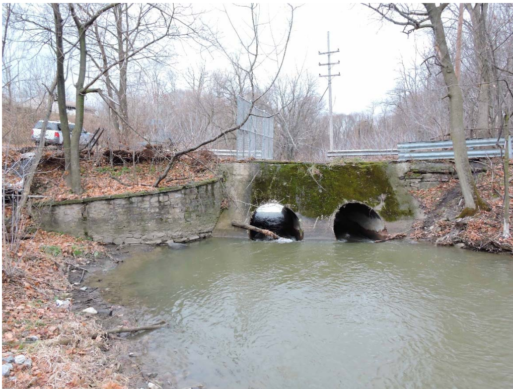
Photograph 25. Structure 16, looking north toward a double culvert with associated stone retaining walls. This structure was likely initially constructed around 1892 when the Lockport Paper company first began
