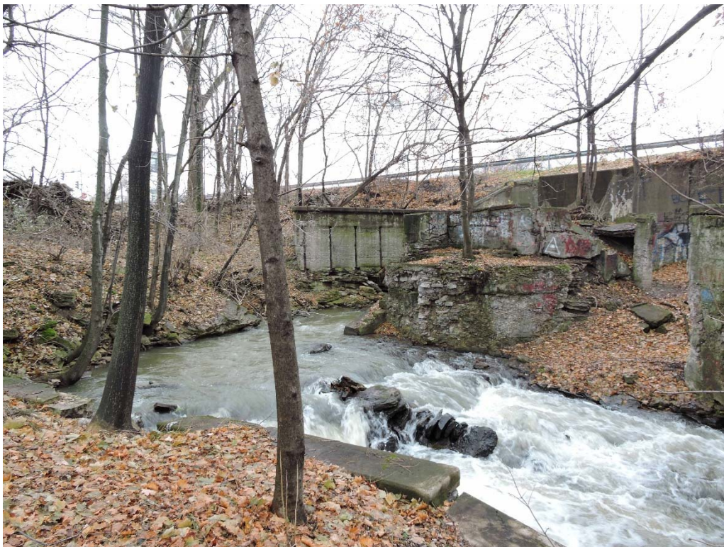
Photograph 35. A view to the southeast of the White Transportation Archeological Site, the concrete tailrace utilized by the Niagara Mills is seen in the foreground. The tailrace for the Leatherboard Mill is further to the west, but its foundation walls can be seen on the other side of the creek.
