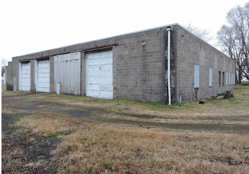
Photograph 19. Structure 12, 34 Mill Street, looking northeast. A one-story concrete block addition to the building, housing four vehicle bays. Sanborn maps indicate that this structure was built after 1948.
