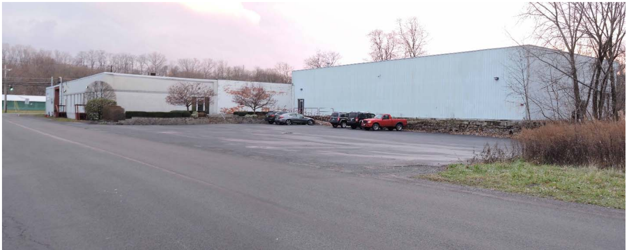
Photograph 23. Structure 14, 62 Mill Street looking southwest. Additions to the east side of the mill complex during the course of the 20 th century entirely obscure the 19 th -century portions of the building.
