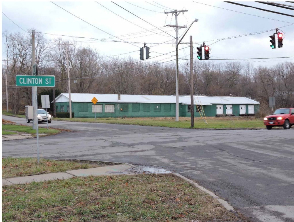
Photograph 18. Structure 12, 34 Mill Street, looking southwest. A one-story masonry building with low-slung gable roof, constructed between 1903 and 1909 for the New York Cotton Batting Co. Sanborn maps describe it as being constructed of "artificial stone"—a term sometimes applied to early concrete block.
