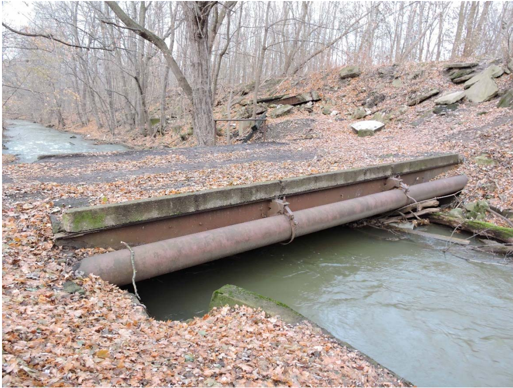
Photograph 24. Structure 15, looking northeast toward an iron and concrete single span bridge, carrying Olcott Street over Eighteen Mile Creek. It appears to date to the early 20 th century. Portions of a concrete wall for the tail race are also seen in the foreground.
