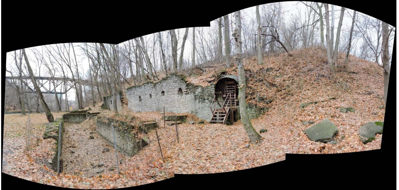
Photograph 37. The Upson Park Archeological Site consists of the former Lockport Pulp Mill that was in operation from about 1889 to 1941. Visible today is the tailrace to the left and steel-lined penstock that brought water from the hydraulic canal.
