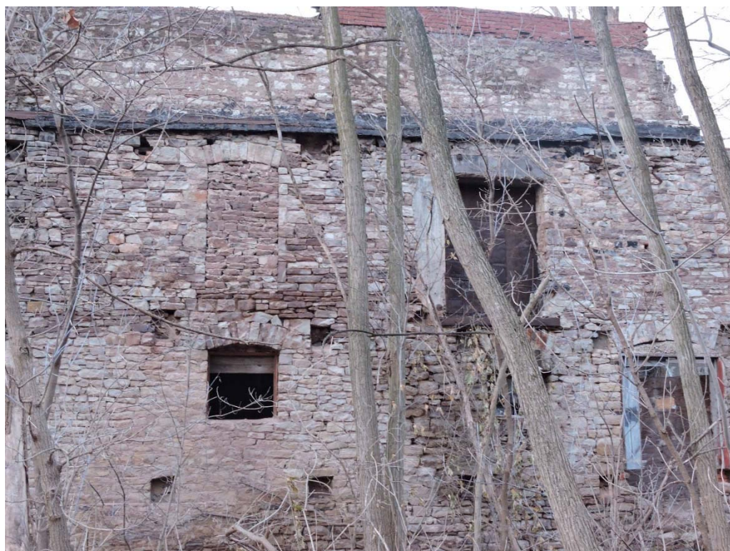
Photograph 26. A view to the north of the southern exterior wall of the former Flintkote mill complex (Structure 17) along William Street. The various building materials in the wall and their orientation suggest a complex structural evolution that likely started about 1850 and continued until the late 20 th century.
