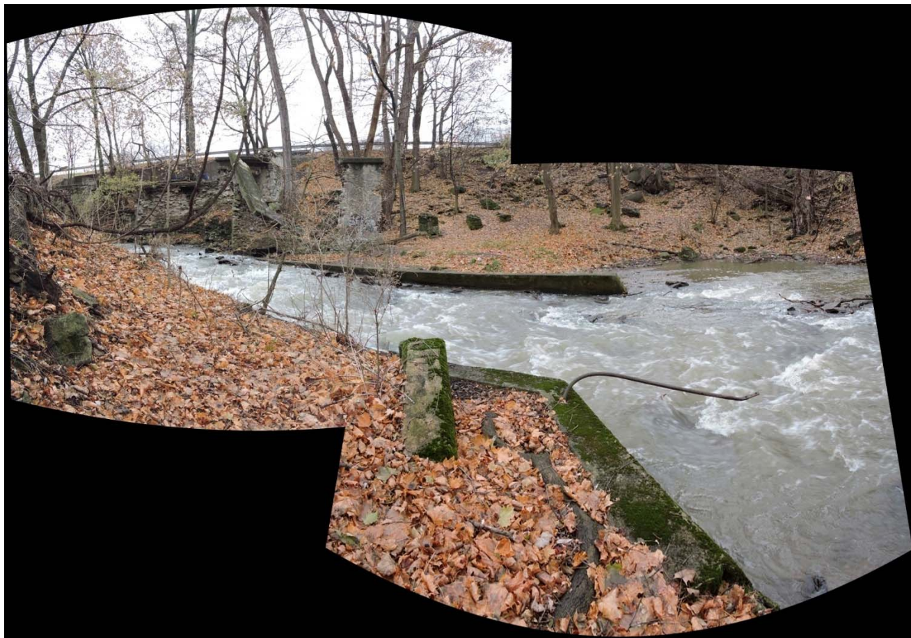
Photograph 36. Another view to the south of the concrete tailrace of the Niagara Mills, the foundation of the Leatherboard Mill is to the south, and its tailrace would have been to the far right of the frame.
