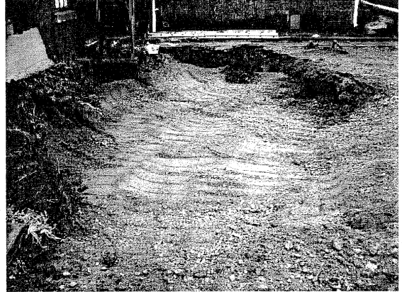
#2 crushed stone used to finish grade of UST excavation looking east
