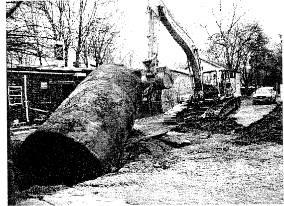
Removing UST from ground looking southeast
