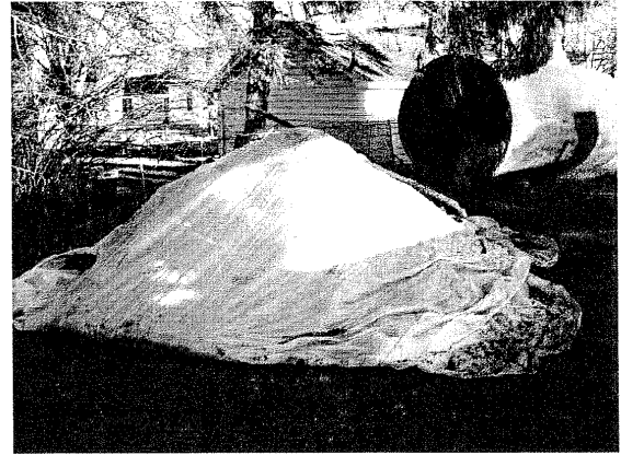
Sand and soil stockpiled to be disposed
