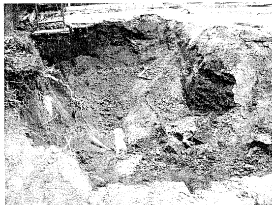
UST excavation looking southeast
