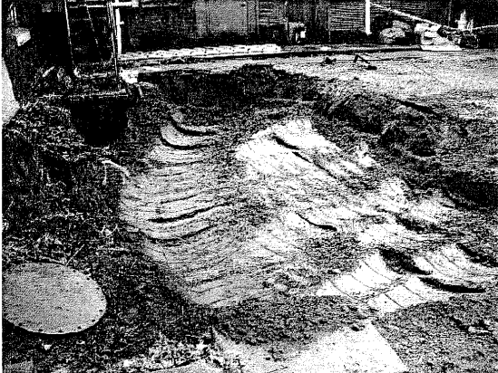
UST excavation backfilled looking east
