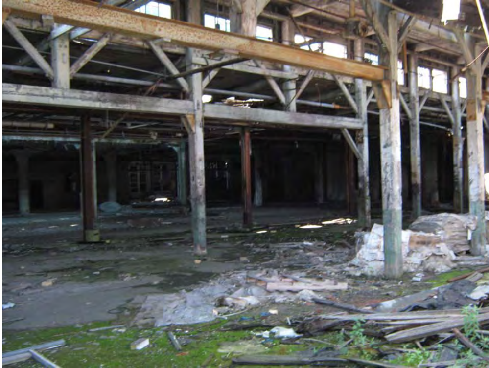
Photograph 1 – Looking south into the Tract I building from a missing window on the north side. The area of investigation was limited to the center building, which is depicted by the reinforced concrete columns in the background. The areas with the wooden timber columns on the north and south sides were not investigated.
