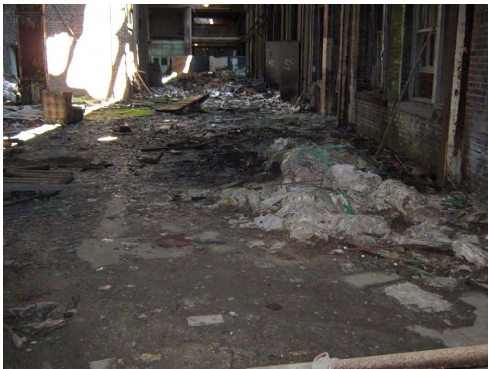
Photograph 8 – Pile of bagged PACM located in the south-central area of the structure. This material might have been illegally dumped.
