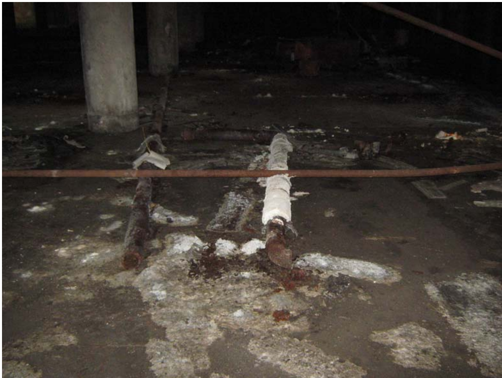
Photograph 6 – Pipe on the floor of the garage still covered with pipe insulation. Note the poor condition of the pipe insulation and the same material on the floor seen in the above photograph.
