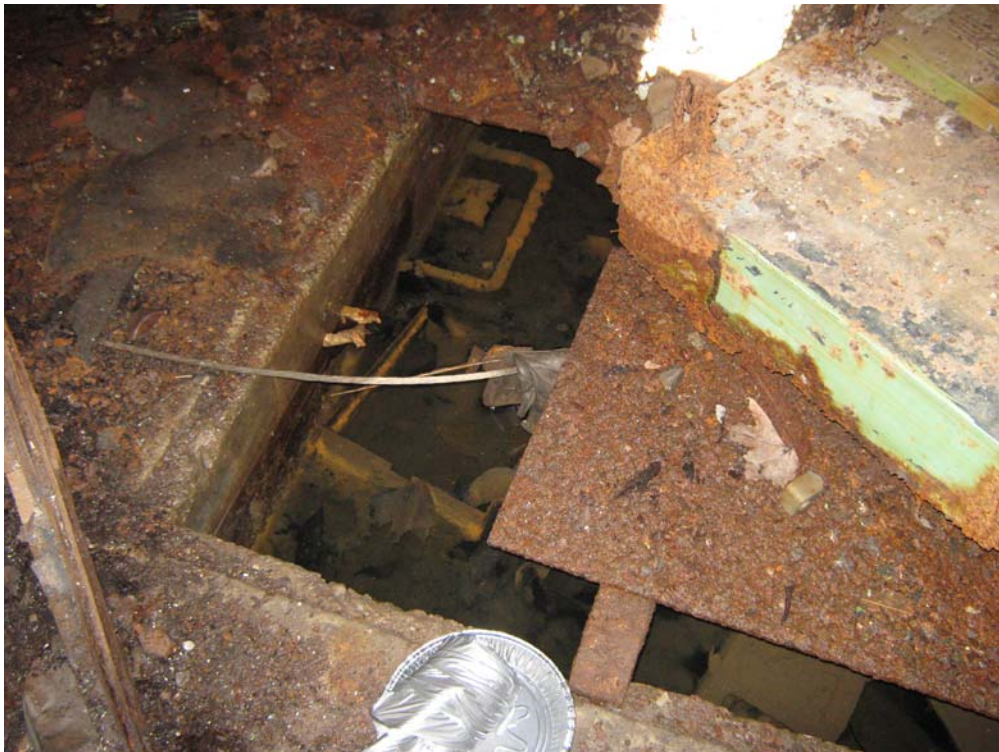
Photograph 12 – The sump in the former mechanical room. A sediment and wipe sample for PCBs analysis was collected from the sump.
