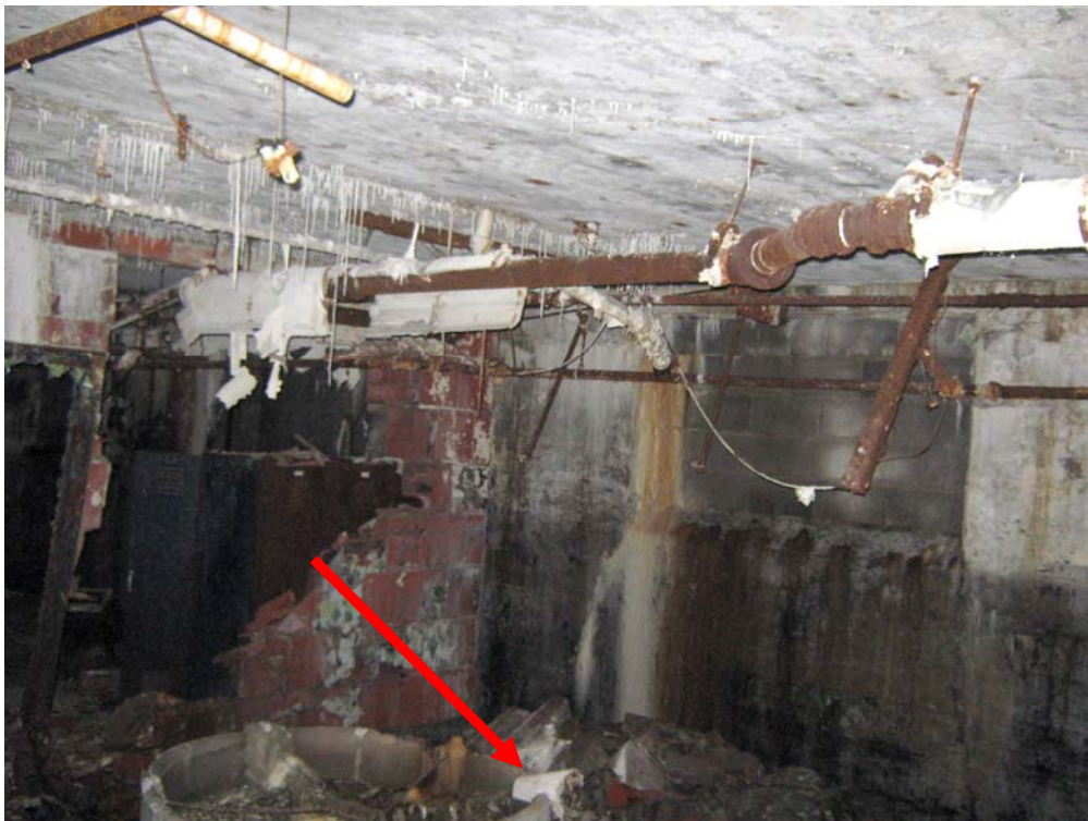
Photograph 10 – Different run of pipe along the ceiling showing the poor condition of pipe insulation. Part of the missing insulation can be seen on ground.
