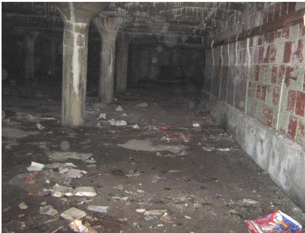
Photograph 2 – Entering the underground garage. The floor is littered with garbage and debris. Note the concrete efflorescence resulting in concrete stalactites.
