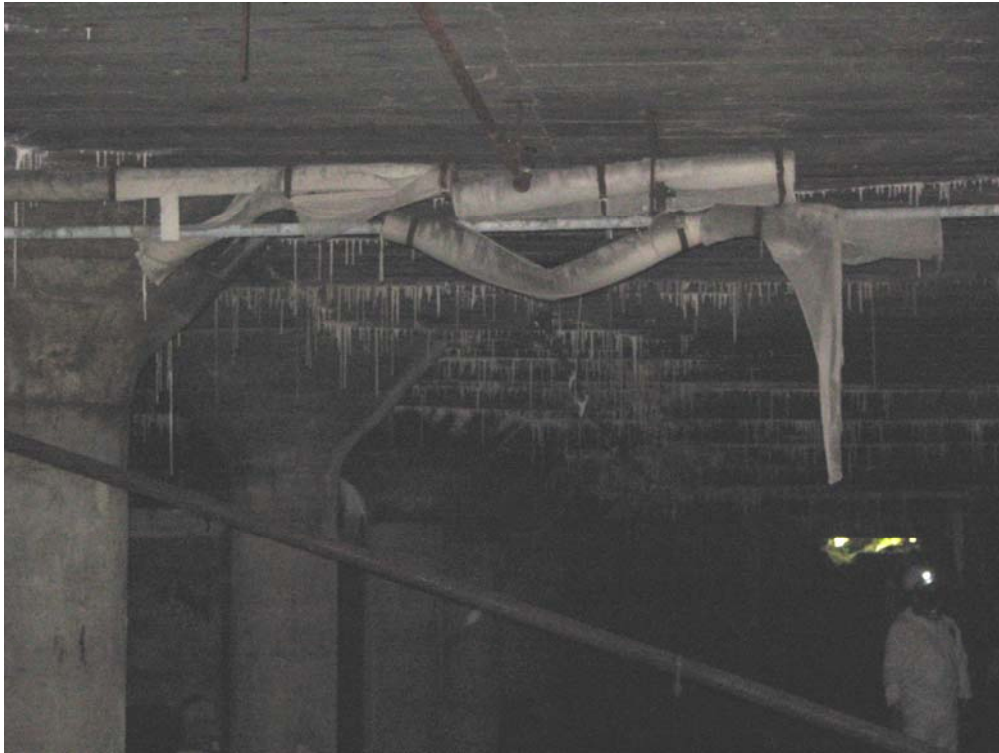
Photograph 7 – Typical condition of pipe insulation hanging loosely from overhead pipe in the underground garage.
