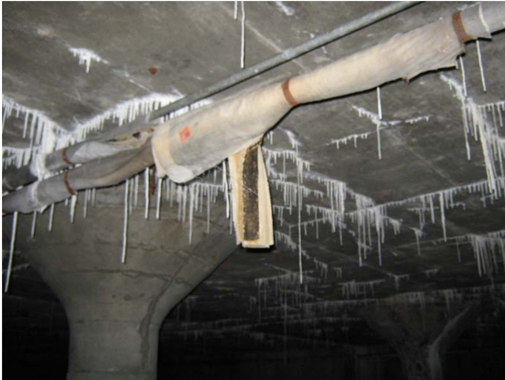
Photograph 3 – Presumed asbestos containing material (pipe wrap) hanging from overhead pipe in the underground garage.
