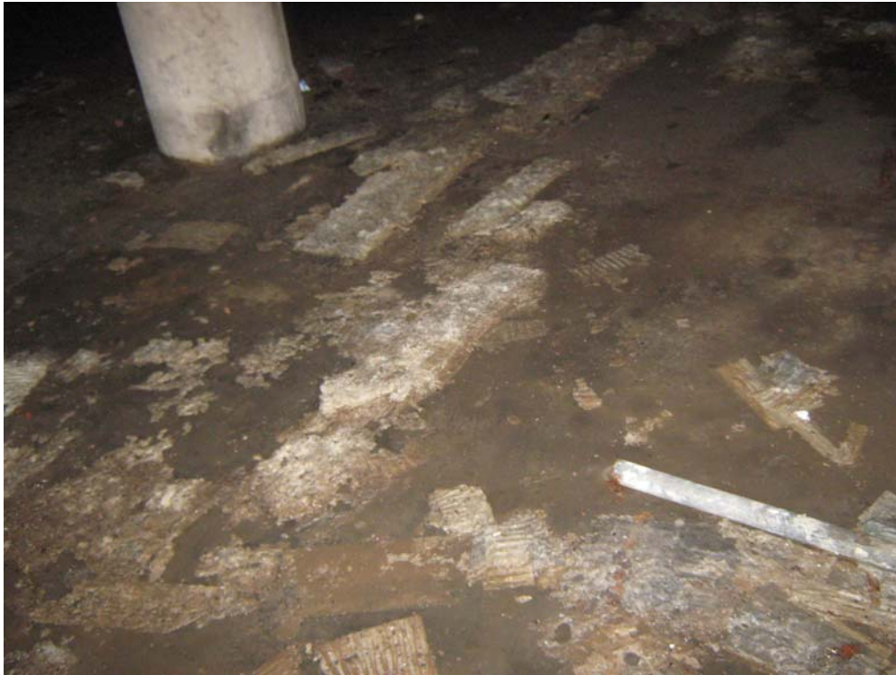
Photograph 5 – Deteriorated pipe insulation on the garage floor. This was found in several areas in the garage.
