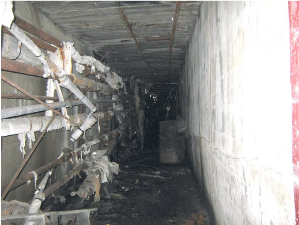
Photograph 11 – Corridor of piping, possibly an old utility run. Note the amount and condition of the pipe insulation.
