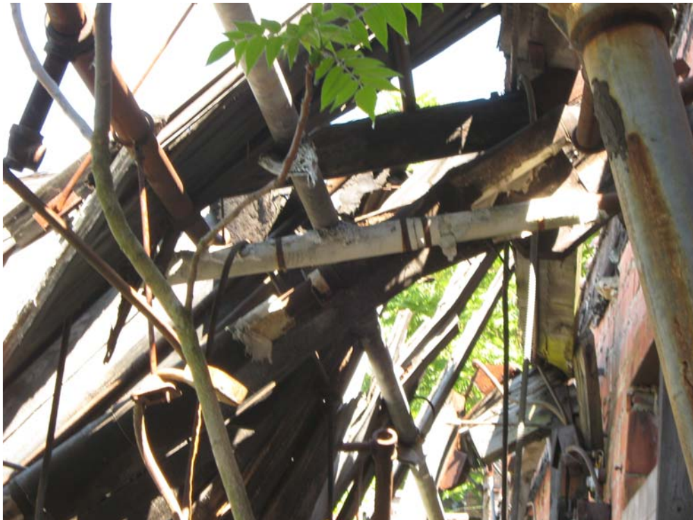
Photograph 16 – PACM in the shed area where the roof has collapsed. The material is in poor condition and is now exposed to the outside air.
