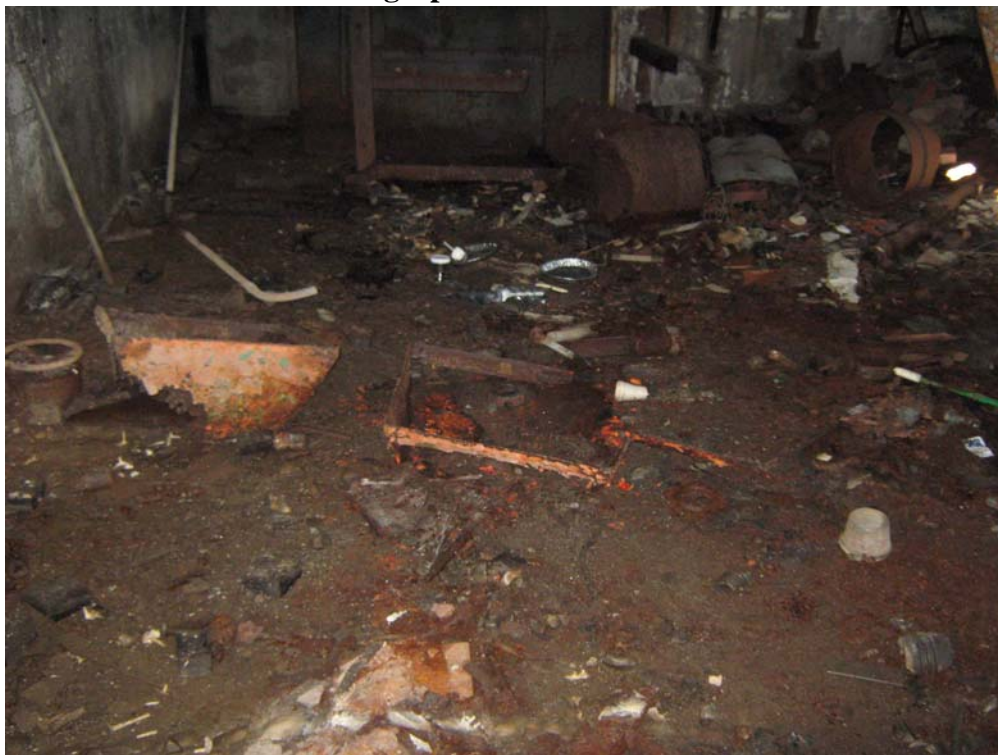
Photograph 13 – Debris on the floor of the mechanical room. Sample Nos. PC2-B-P-01 and PC2-B-P-02 were collected from floor debris and submitted for PCBs analysis.
