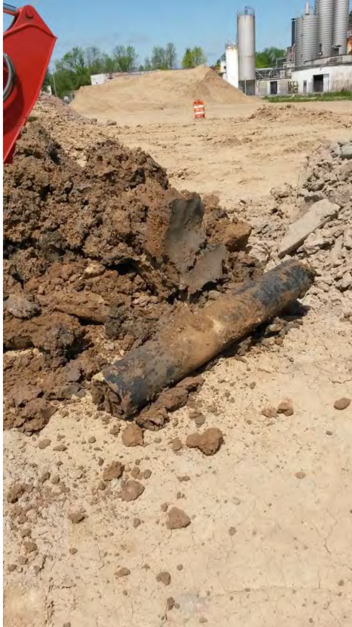
View of a piece of the pipe that was removed from the subsurface at test pit LNAPL-20 on May 19, 2015.
