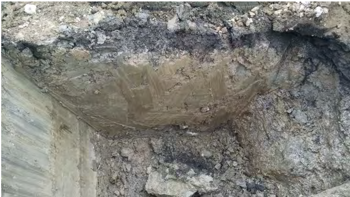
View of test pit LNAPL-17 upon completion on April 23, 2015.
