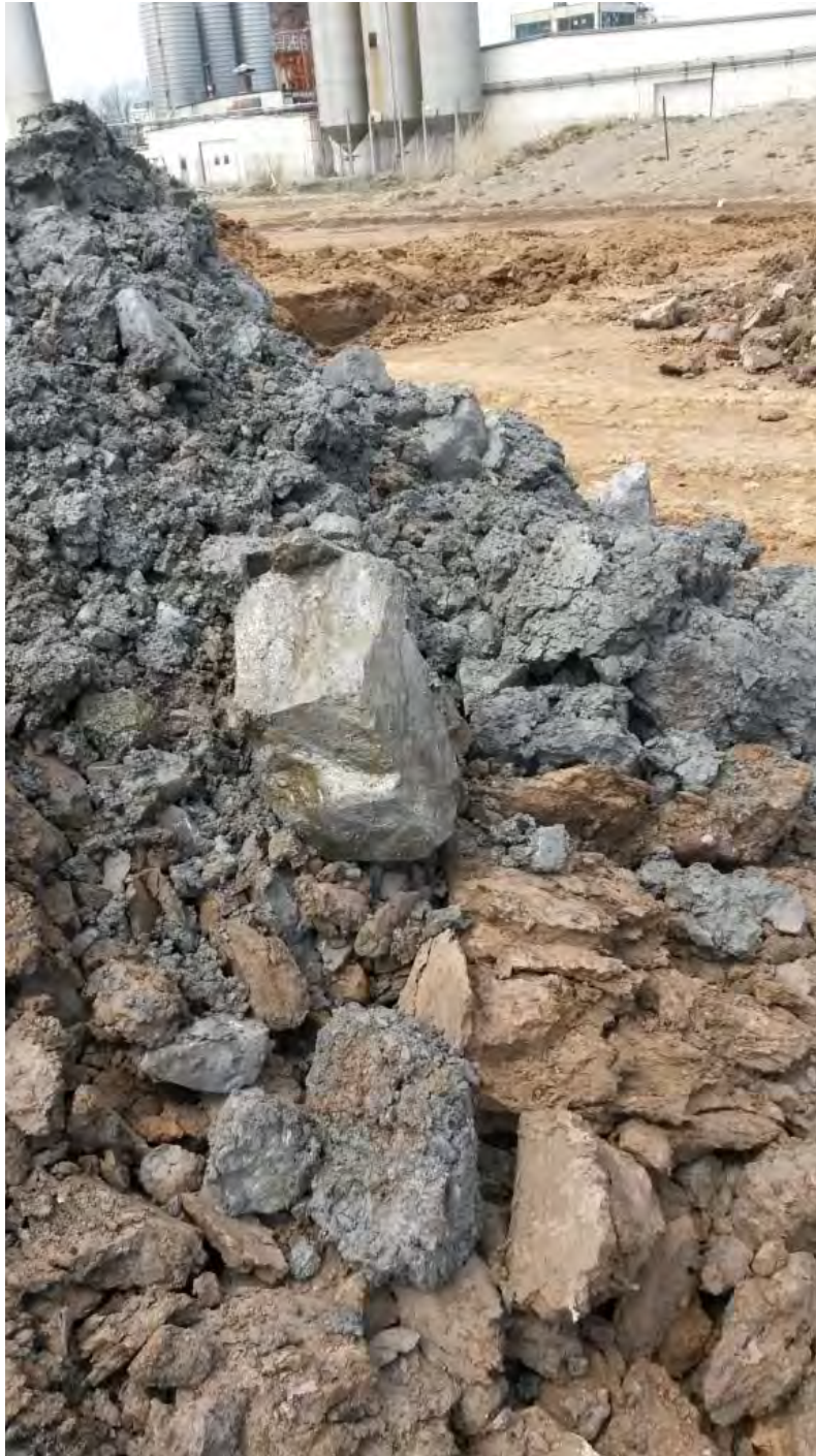
View of soil excavated from test pit LNPAL-20, showing NAPL impacts. This was segregated and transported for landfill disposal.
