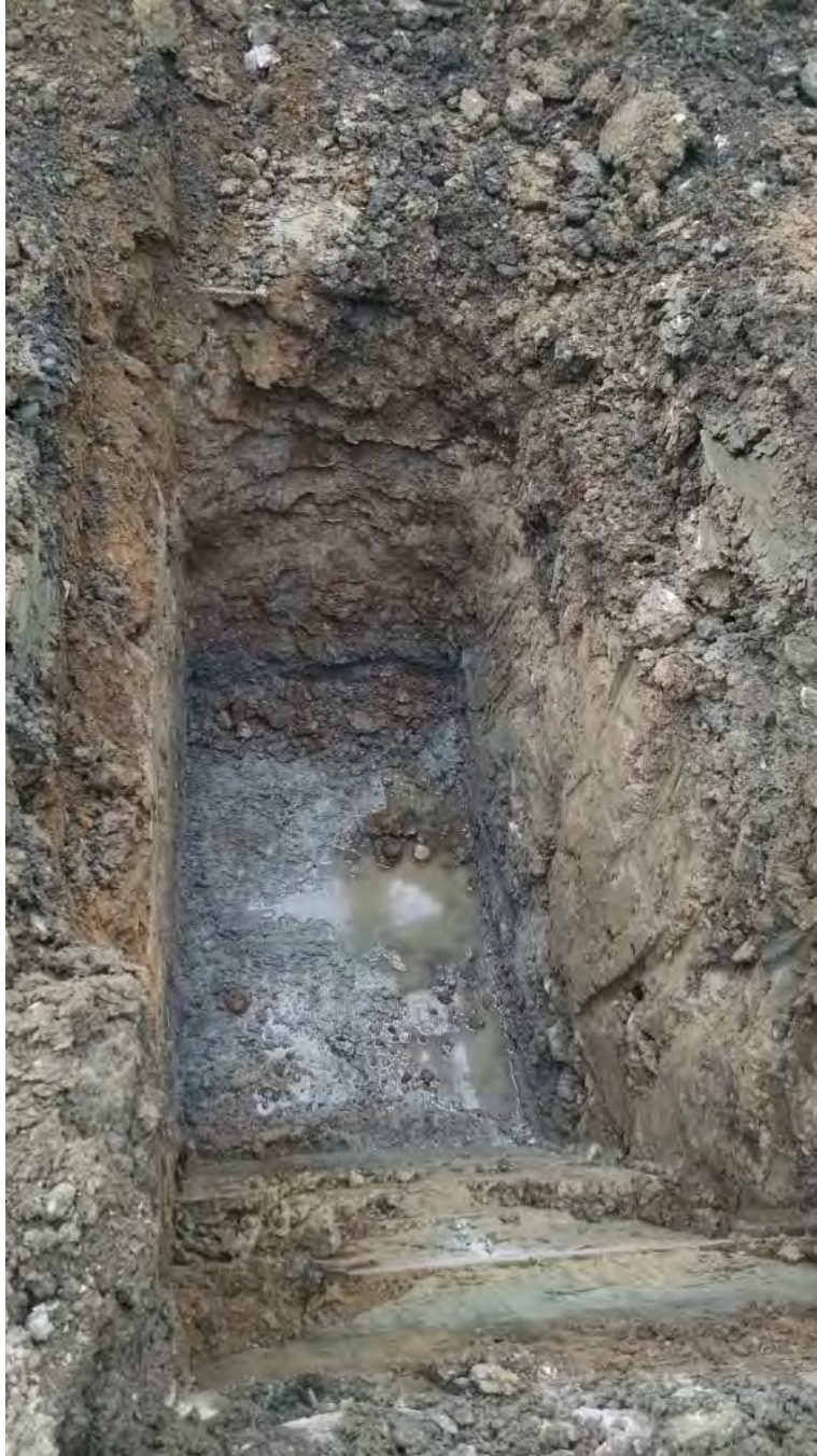
View of test pit LNAPL-13 upon completion on April 23, 2015.
