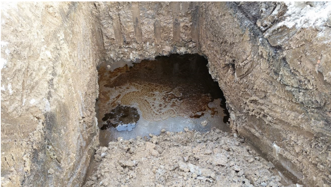
Photo 5: Petroleum product observed in Test Pit and subsequently remediated
