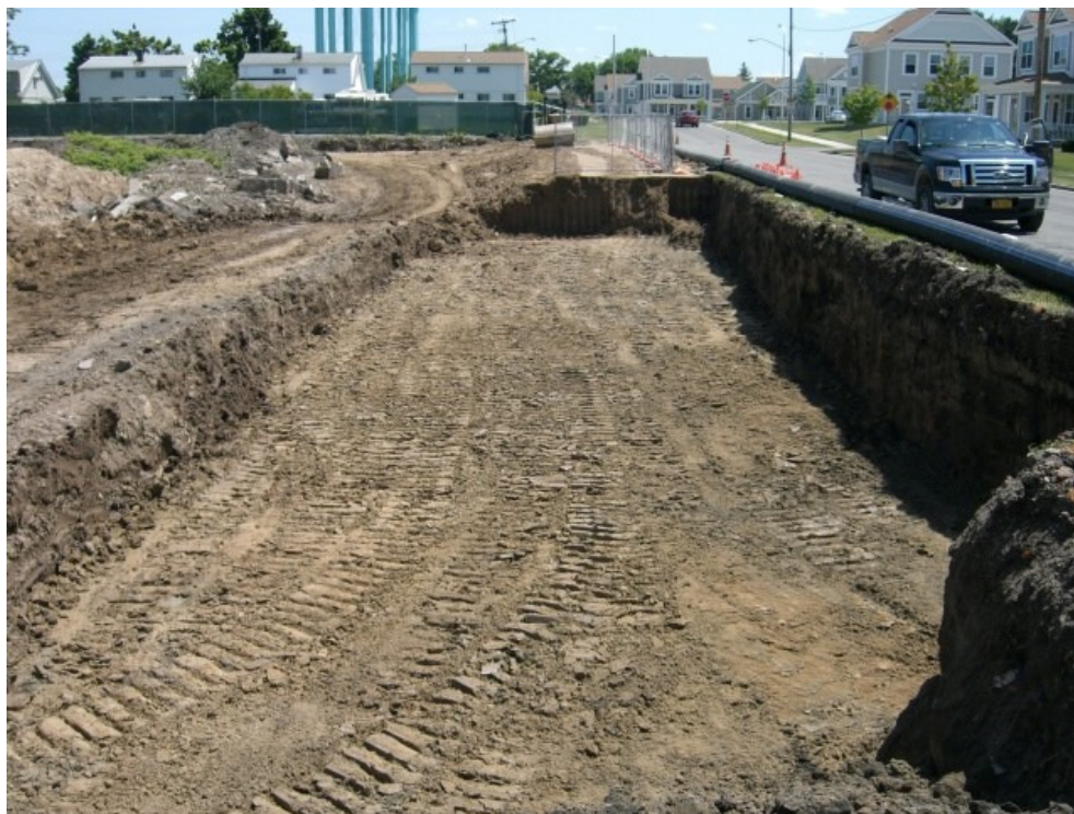
Photo 9: Remediation along Beech Street
