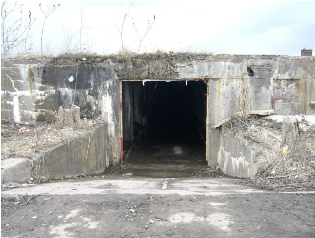
Photo 4: “Underground Structure” in Park Area prior to removal.
