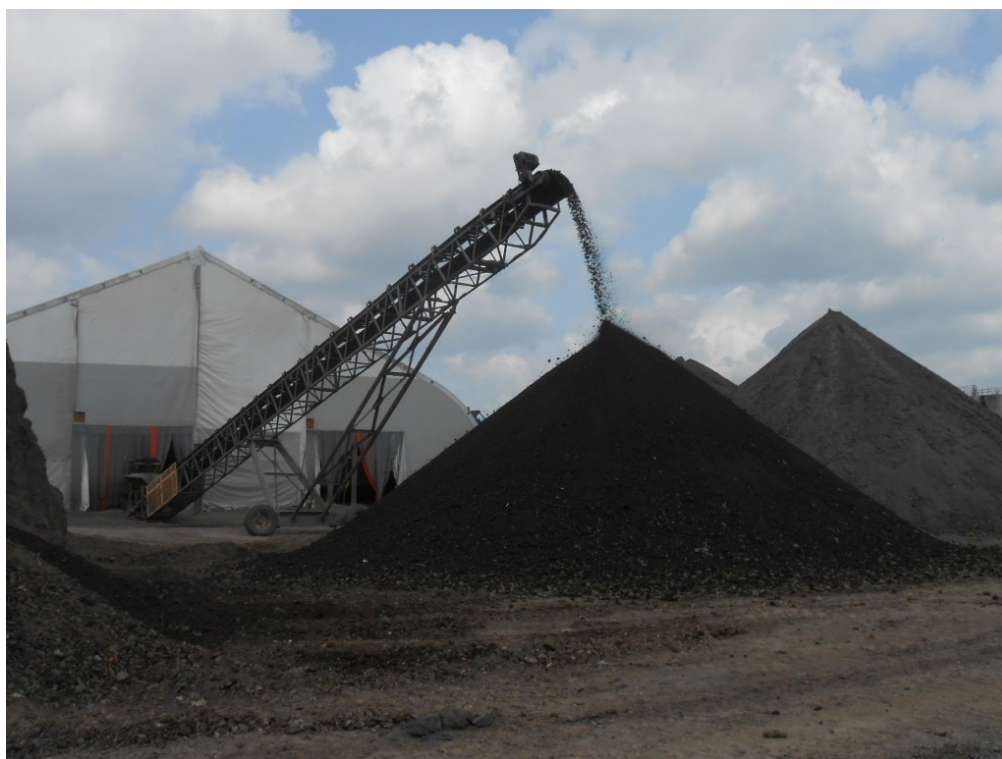
Photo 1: Pugmill in operation (inside tent structure) conveying stabilized lead impacted soils
