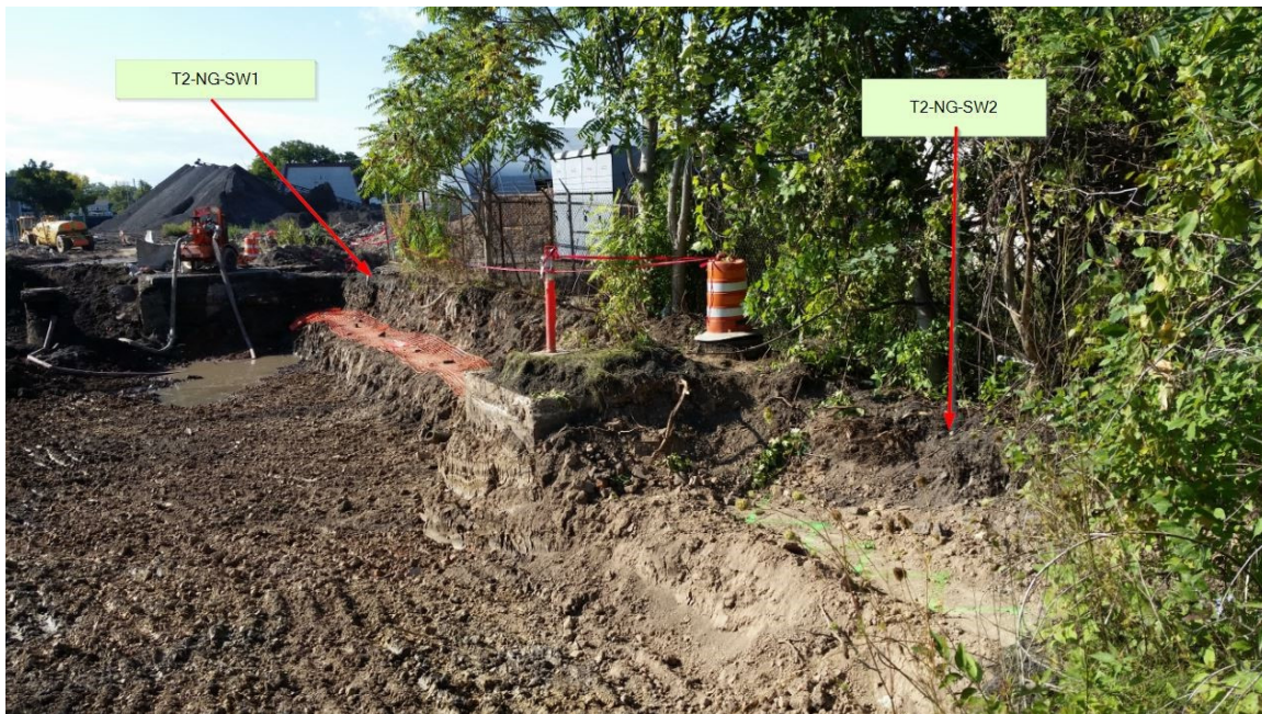
Photo 6: West edge of 15 th St ROW prior to further excavation westward onto Tulip property
