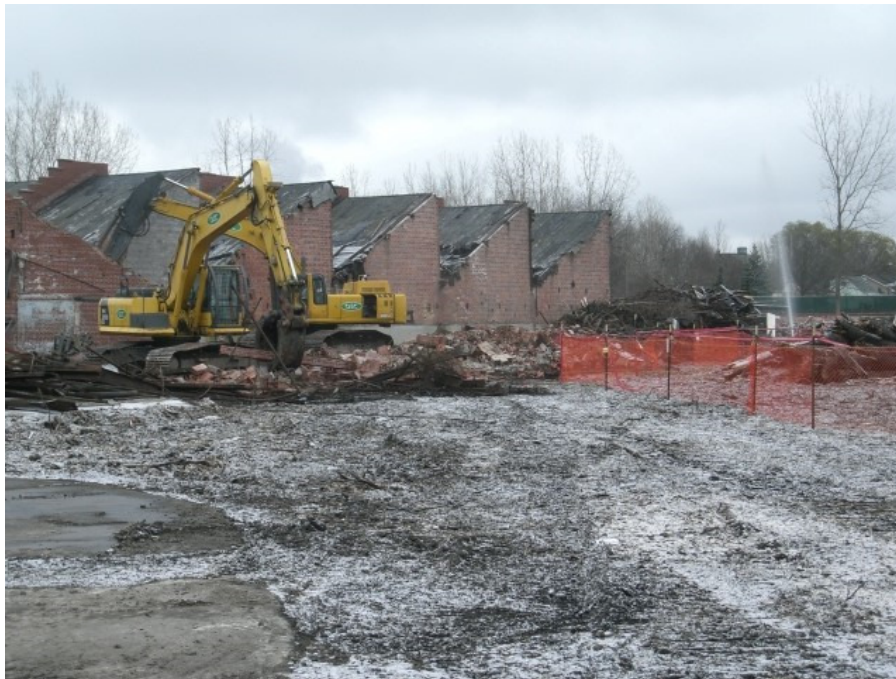
Photo 7: 17 th St Warehouse prior to demolition
