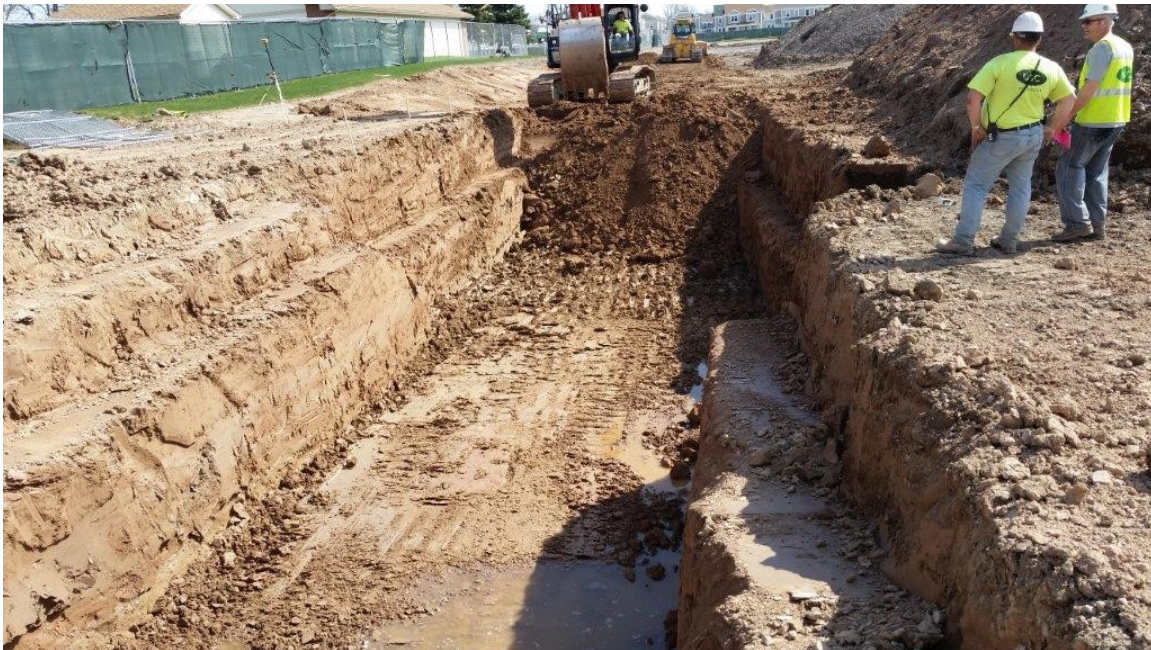
Photo 11: Excavating clay fill from borrow Pit (subsequently infilled with treated soils)
