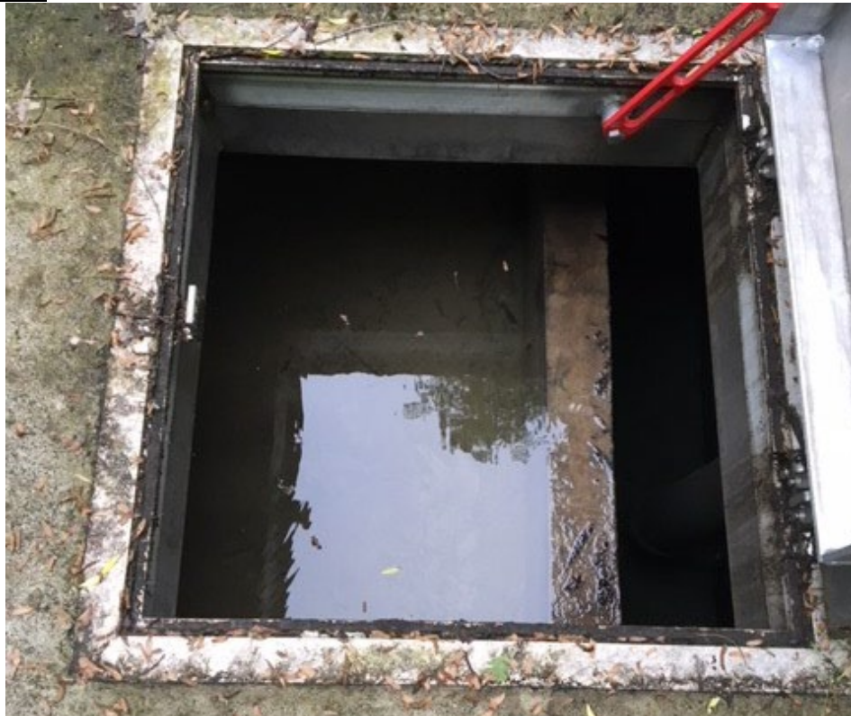
Photo 1: Interior of filter vault – top of sand filter bed (November 25, 2019).
