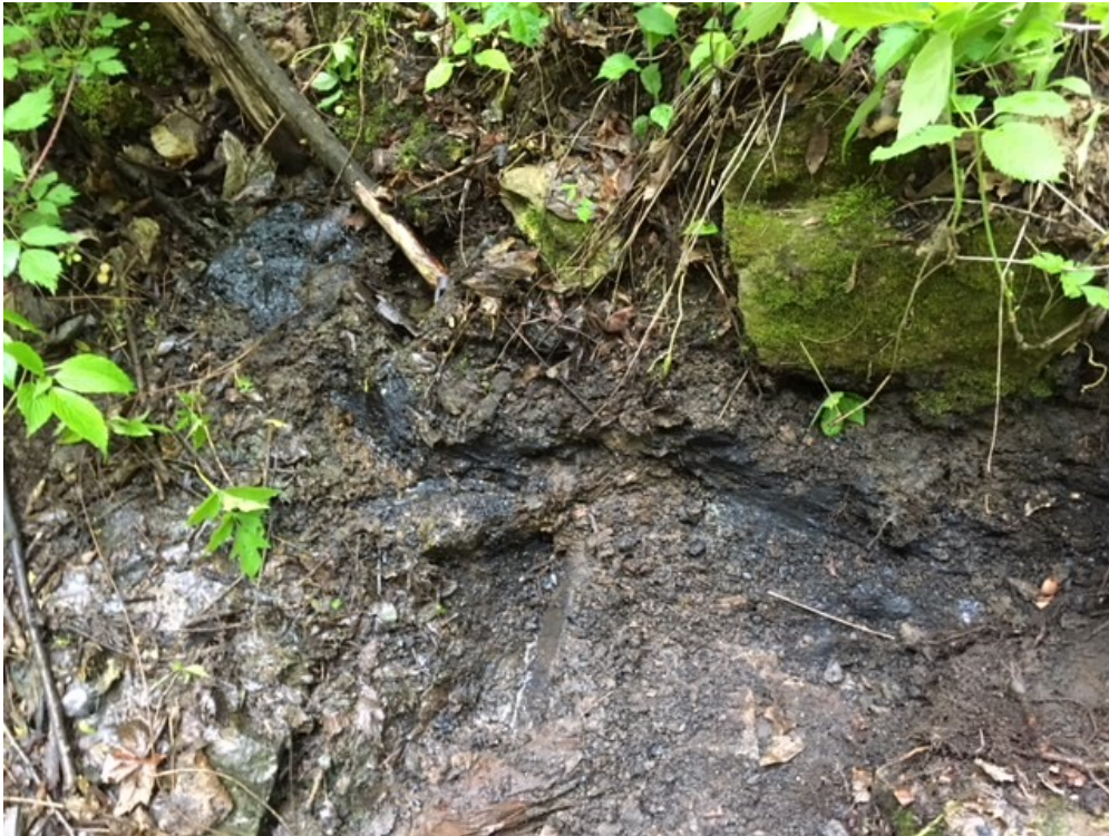
Photo 7: Residual tar removal area- south side of stone structure (May 29, 2019).
