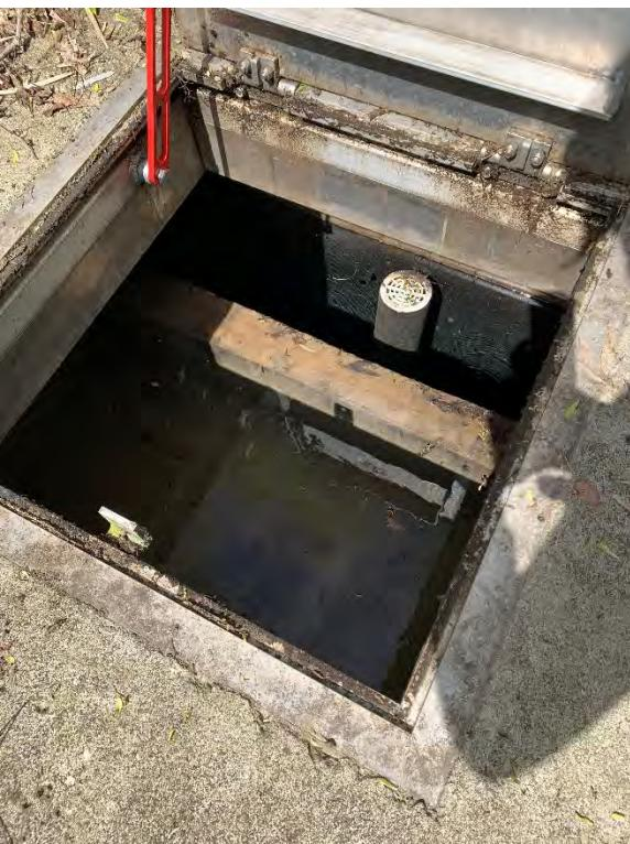
A photograph showing the interior of a concrete filter vault. The water level is high, covering most of the sand filter bed. A red metal ladder or tool is leaning against the left wall. A circular vent or access cover is visible in the center of the chamber floor. The concrete walls and floor show signs of age and wear. |
