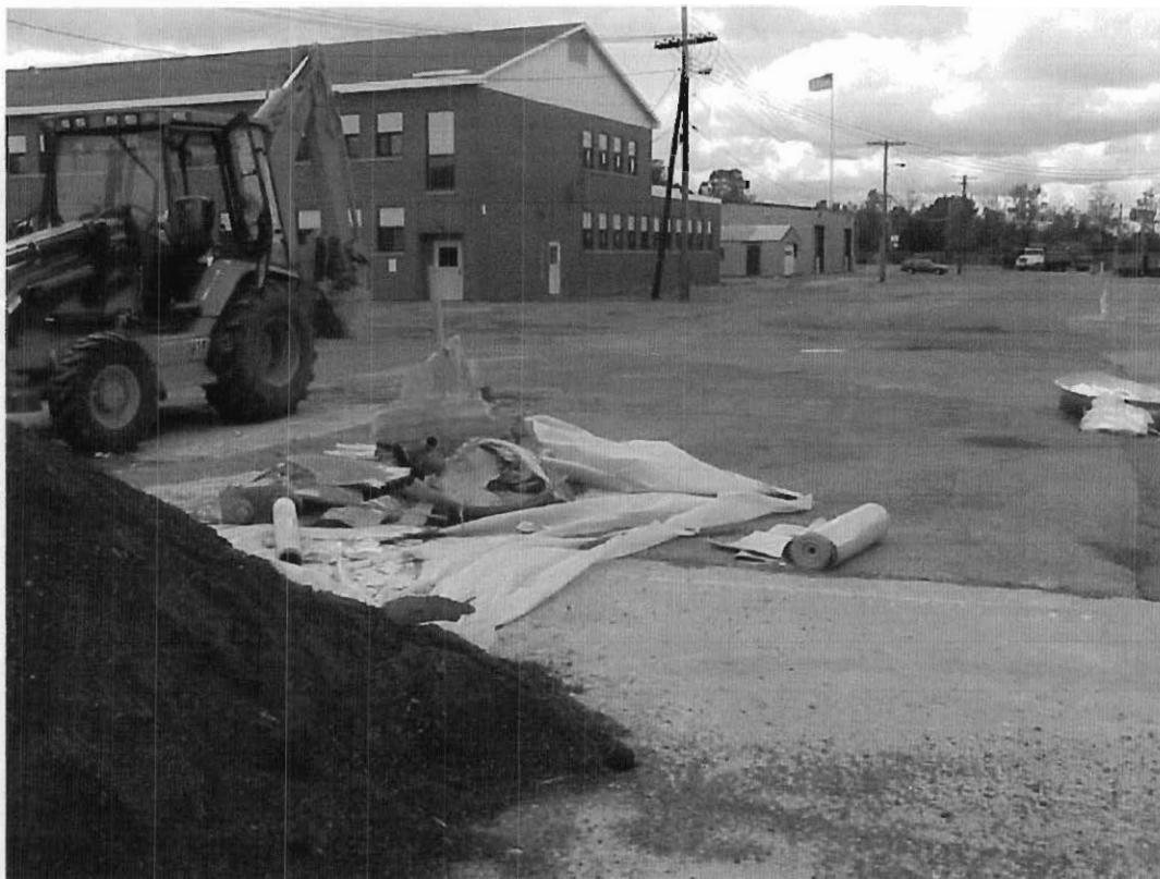
9/20/99 - Tank and piping removed and staged in pieces on plastic.
