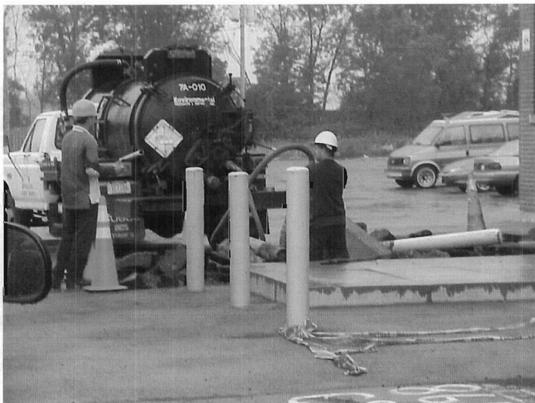
9/20/99 - Removing residual liquids from the UST, prior to tank removal.
