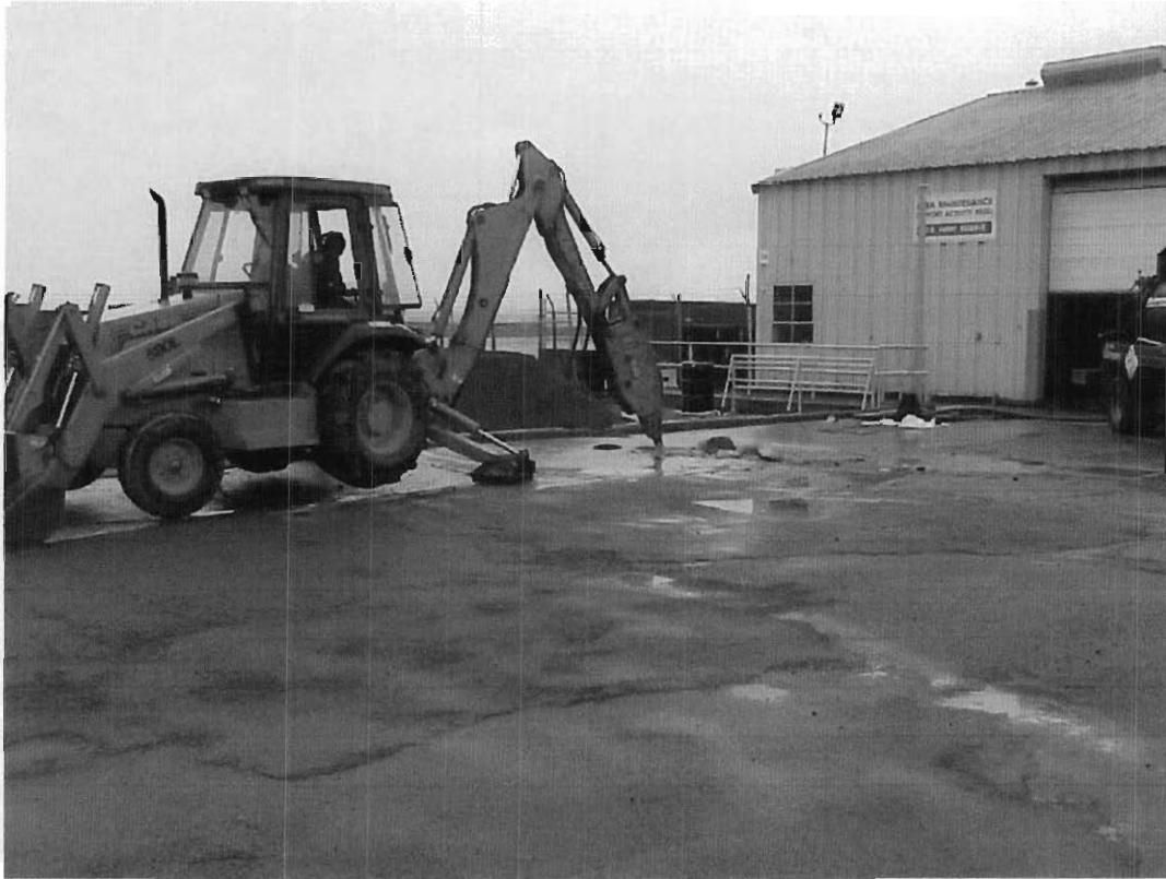
9/20/99 - Hydraulic concrete breaker demolishing concrete cover above UST.
