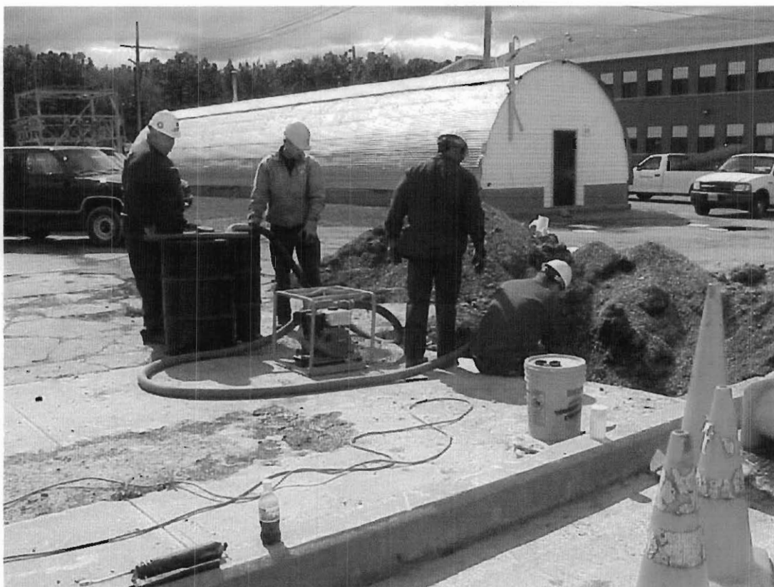
9/20/99 – Transfer of groundwater from the excavation into 55-gallon drums.
