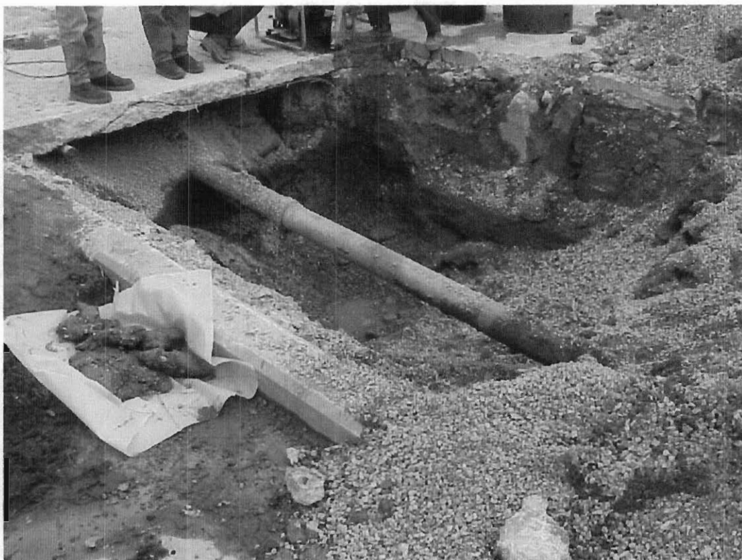
9/20/99 – Excavation pit following removal of the groundwater.
