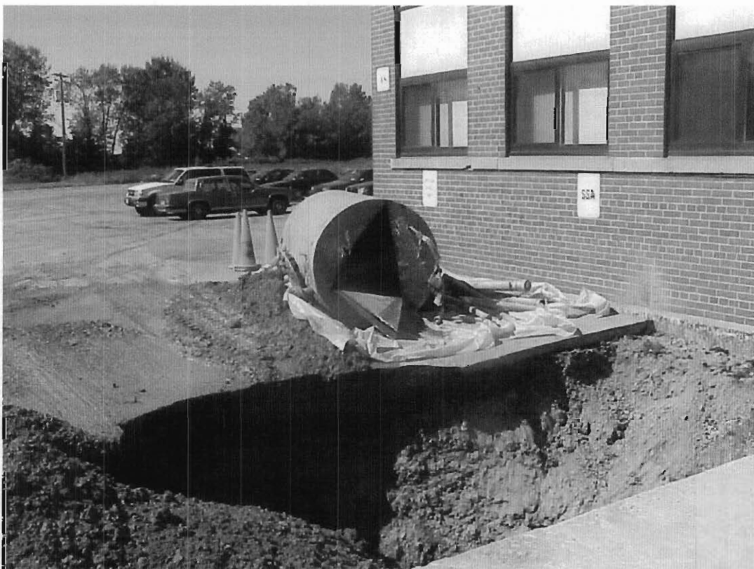
9/22/99 – UST rendered useless prior to transportation to scrap yard.
