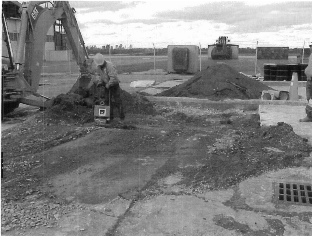
9/21/99 - Compaction of sub-base material prior to installation of concrete.
