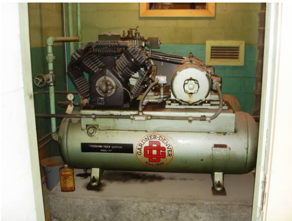
11. View north, Building 4S, first floor, unused air compressor. Note oil staining and oil container on floor/pad. Potential lead-based paint on wall.
