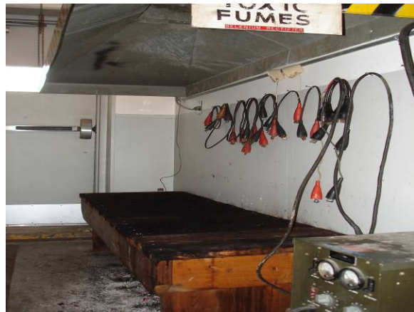
12. View west, Battery Room in Building 18, AMSA portion. Note charred wood bench and corrosion deposits on concrete floor.
