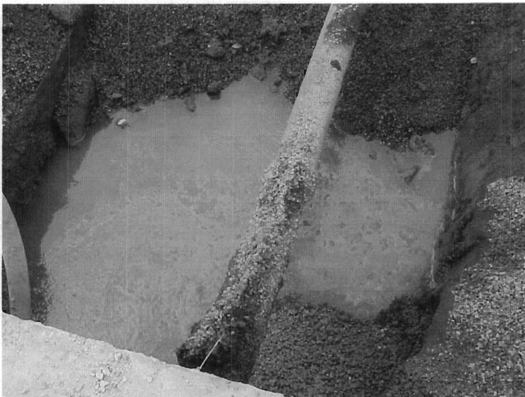
9/20/99 - Excavation pit following UST removal. Concrete footer and pooled groundwater are visible
