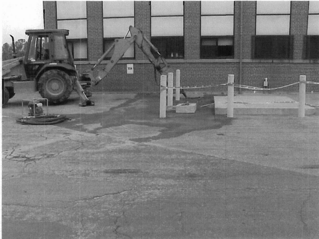
9/22/99 - Hydraulic breaker demolishing asphalt cover above the UST.
