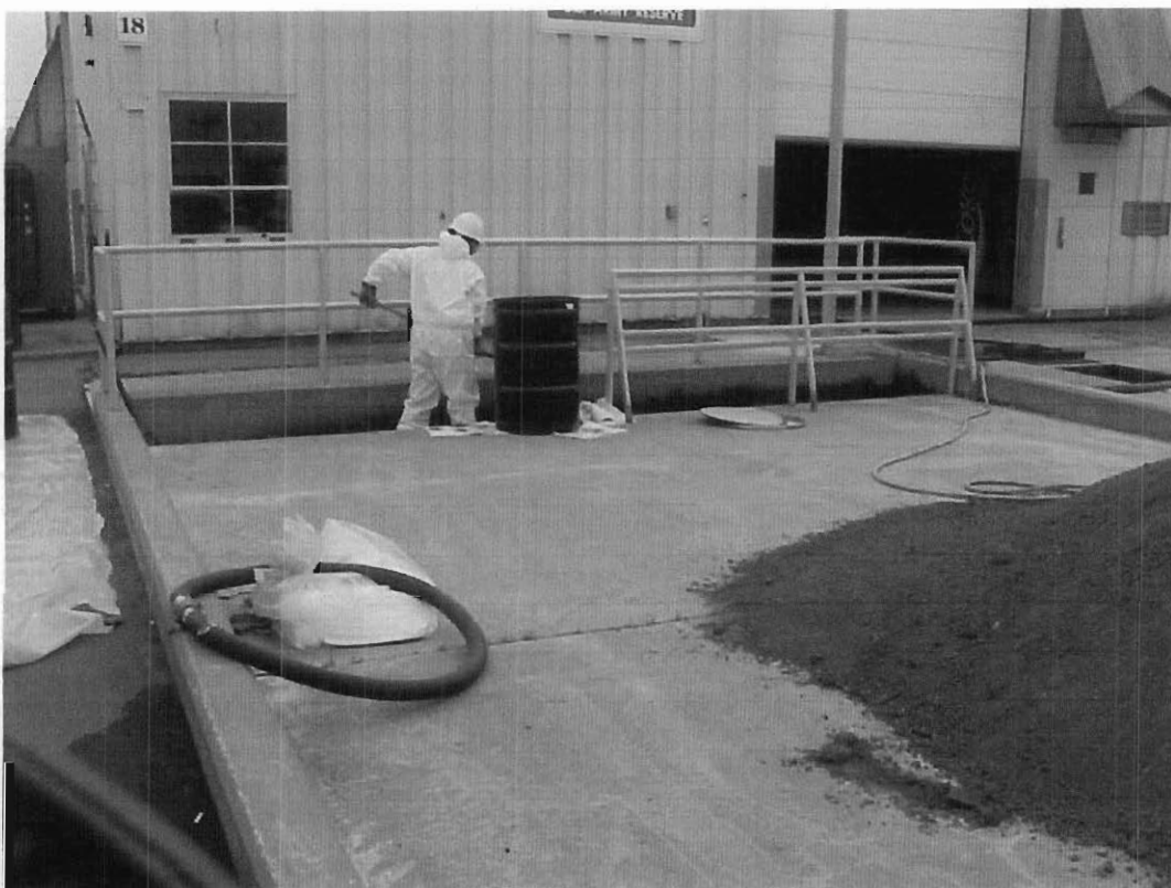
9/20/99 – Transfer of waste soil/debris material from trench drain and OWS into 55-gallon drums.
