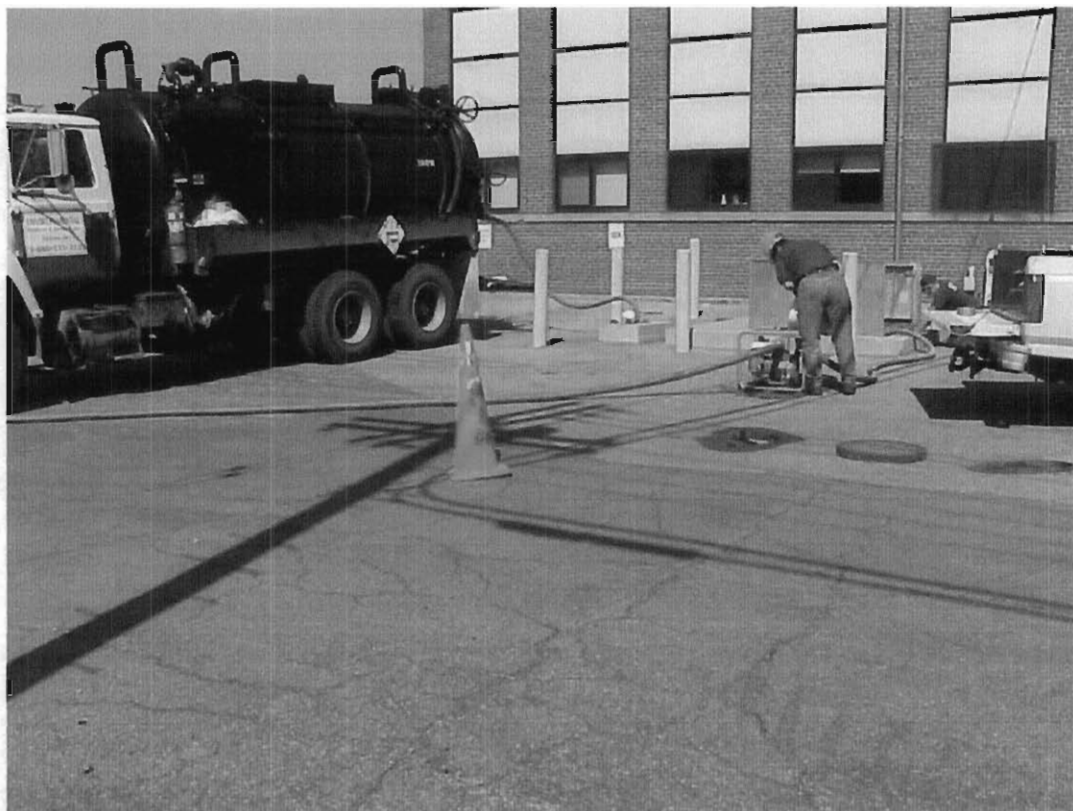
9/14/99 - Removing liquids from UST/OWS and concrete vault.
