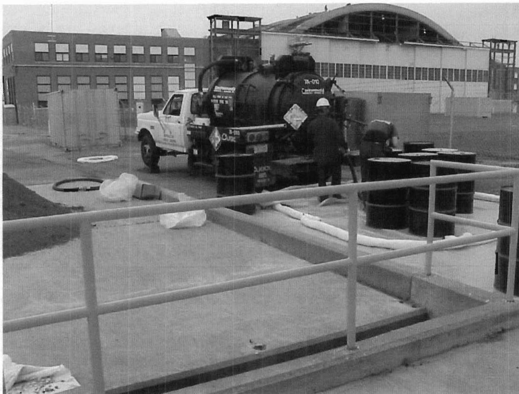
9/20/99 – Transfer of waste liquid from UST and OWS into 55-gallon drums, placed on staging pad.
