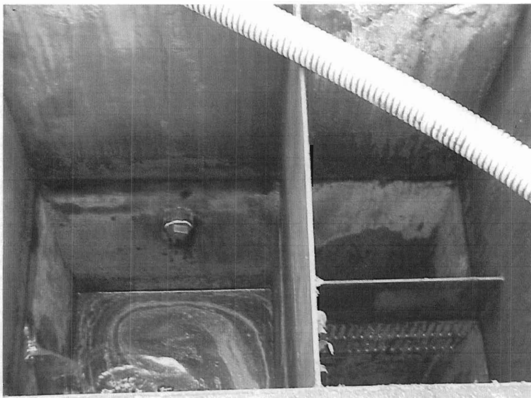
9/20/99 - Outlet from OWS to UST is plugged with a threaded, two-inch, galvanized steel plug.
