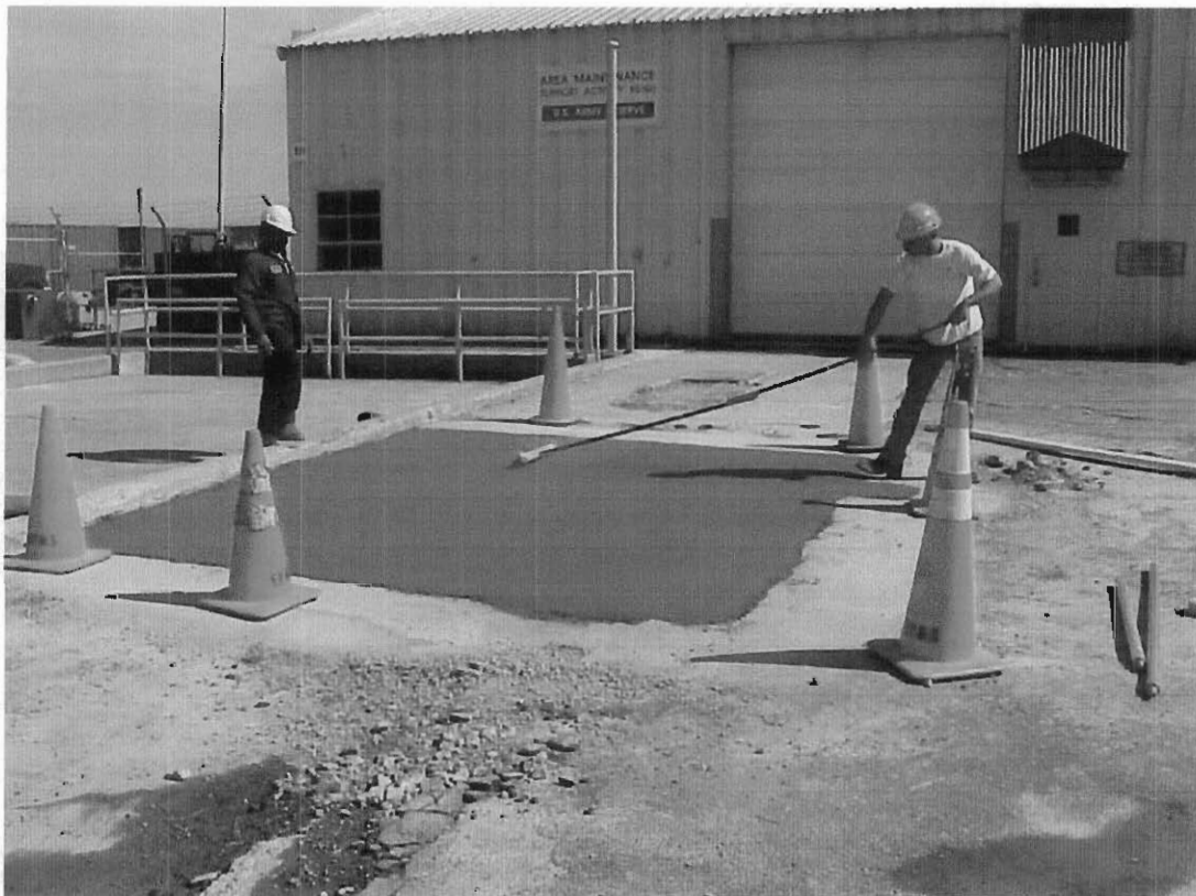
9/23/99 - Concrete restoration following UST removal activities.
