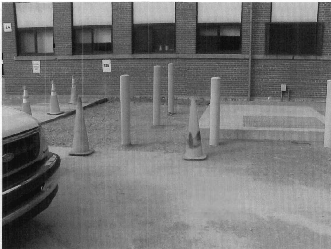
9/22/99 – Preparation for asphalt restoration. Compacted sub-base with bollards reset and repainted.
