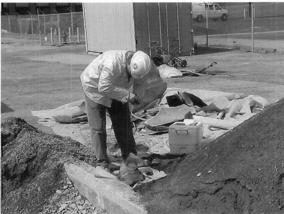
9/20/99 – Collecting samples of excavated soil.
