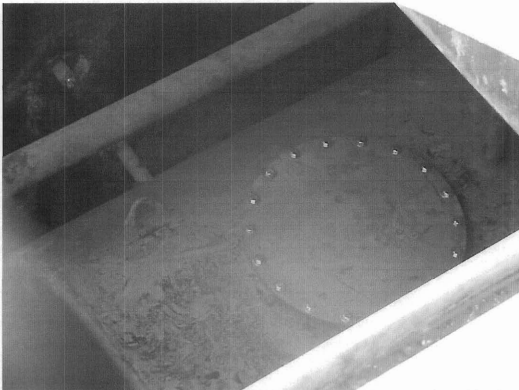
9/23/99 – New OWS manway gasket and bolts. Piping from OWS to UST is cut/capped inside vault.
