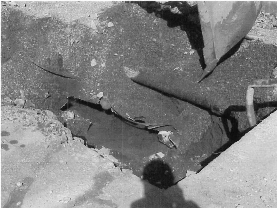
9/20/99 - UST ripped during excavation (groundwater entering). Sanitary line visible above the tank.
