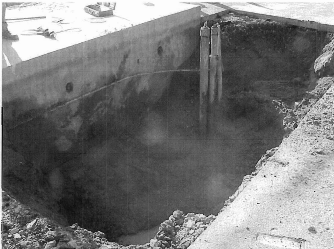
9/22/99 - Top of UST exposed during excavation. Oil feed line from OWS to the UST is visible.
