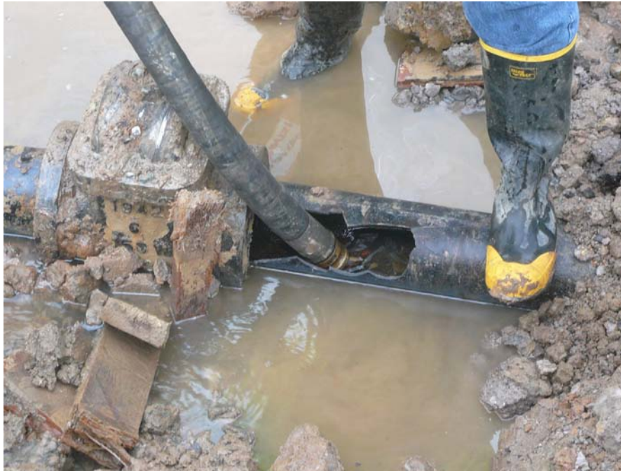
Photograph 3 – Pumping of Fire Protection Main prior to removal.
