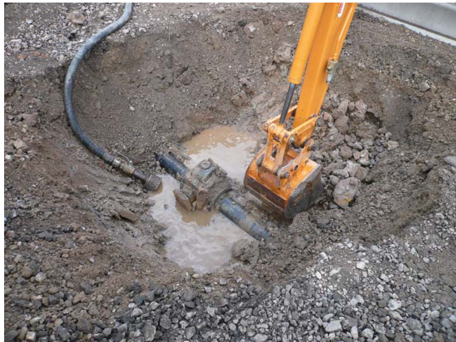
Photograph 2 – Excavation and 6" Fire Protection Main as viewed from the southeast.
