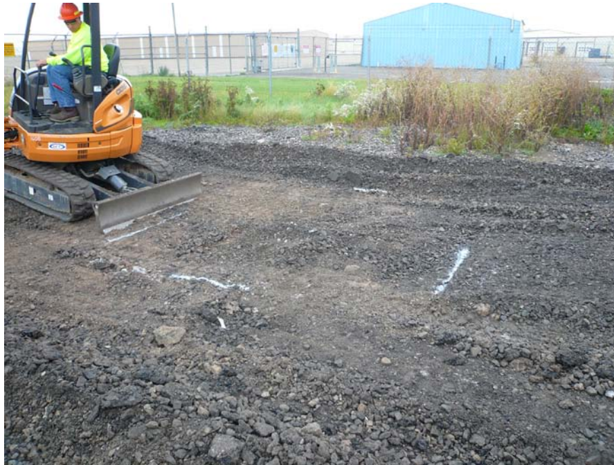
Photograph 1 – Area of IRA prior to excavation as viewed from the west.
