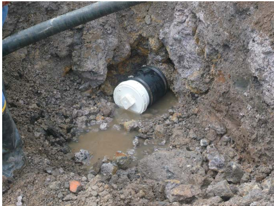
Photograph 4 – Capped end of the Fire Protection Main.
