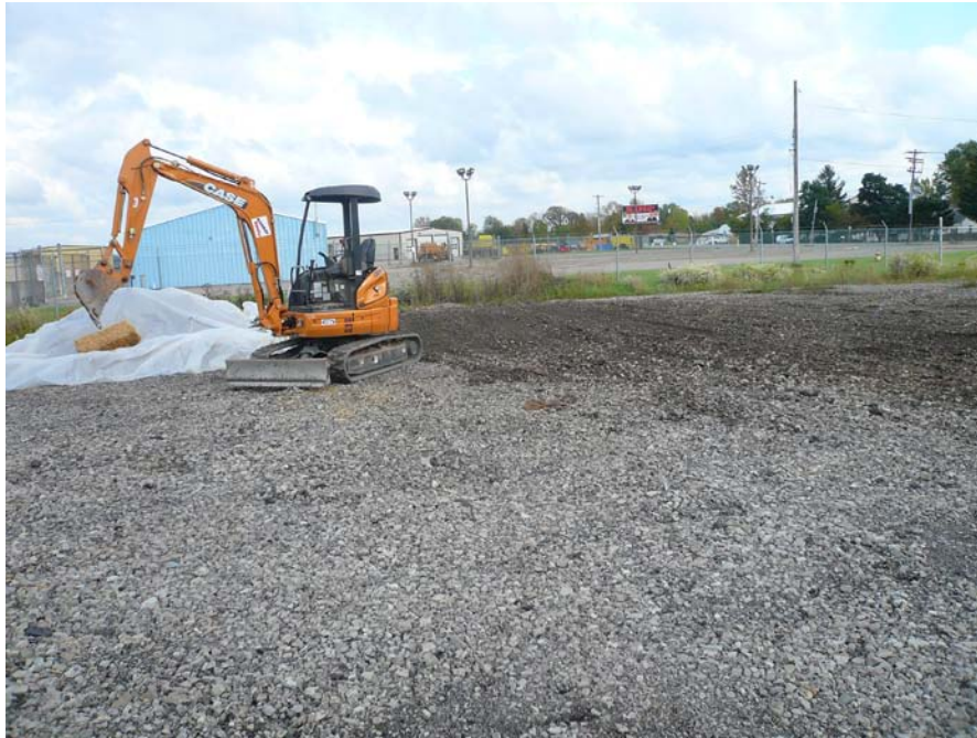
Photograph 5 – Backfilled excavation as viewed from the west.
