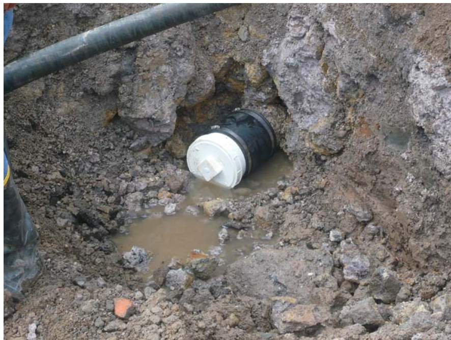
Photograph 4 – Capped end of the Fire Protection Main.
