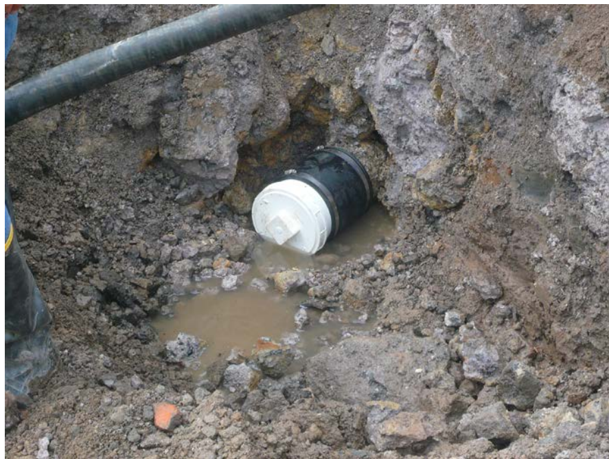
Photograph 4 – Capped end of the Fire Protection Main.
