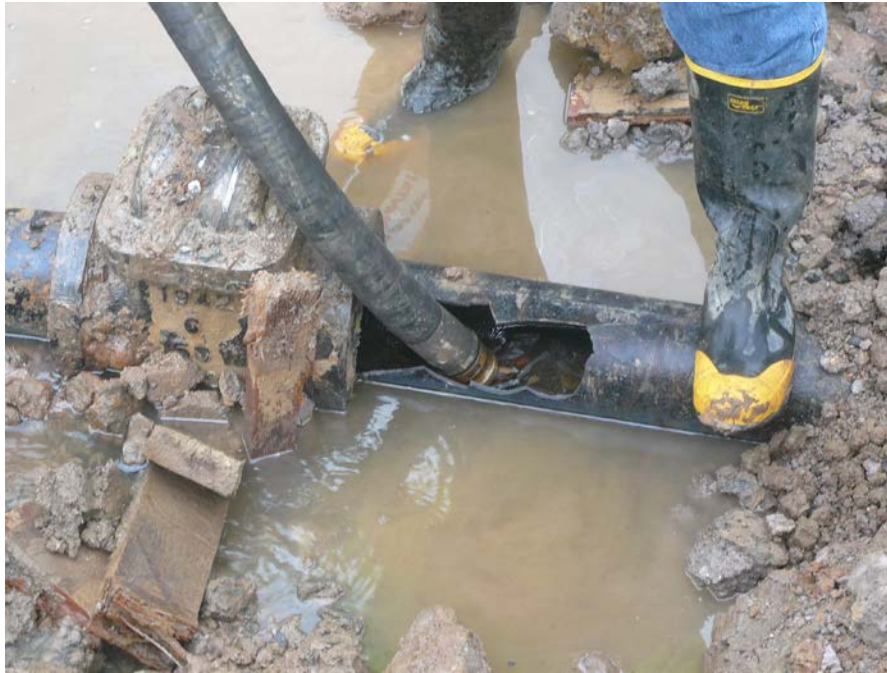
Photograph 3 – Pumping of Fire Protection Main prior to removal.
