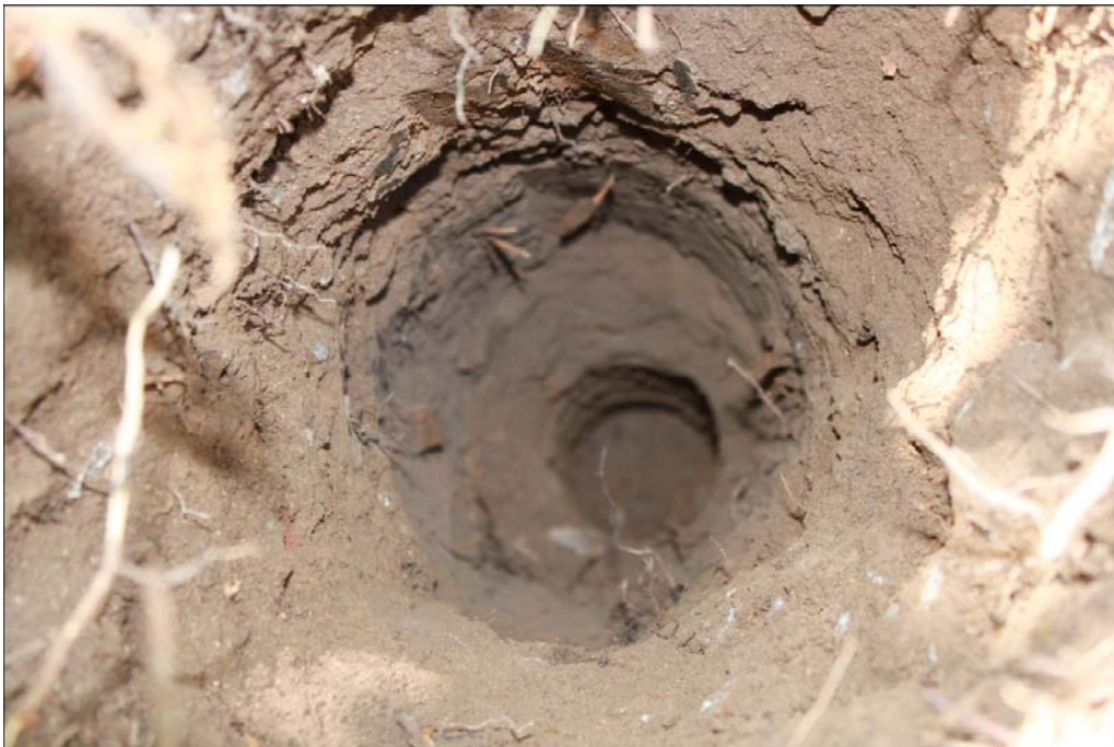
Photo 5 - Soil Boring 1 after soil was removed. Notice the rocks lined around the hole extending down approximately two feet. Rocks were encountered in every six-inch lift through the mound until reaching native soil.
