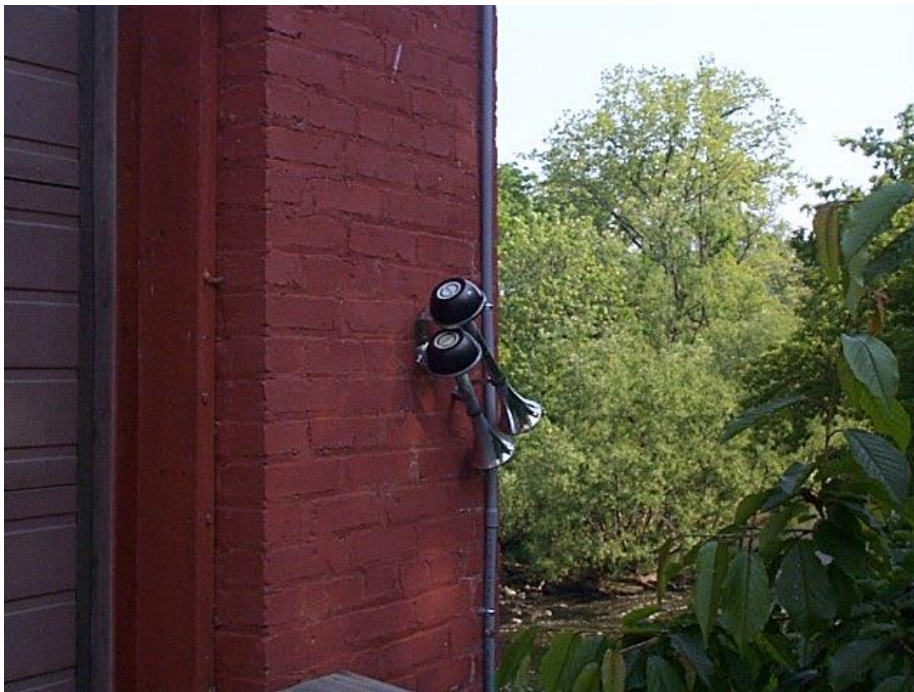
Photo No. 8 - Tailrace siren located on the end of east powerhouse wall.
