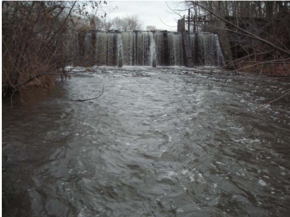
Photo: P75A Direction of view: S Description: View of Newfane Dam spillway from LDB of right channel.
