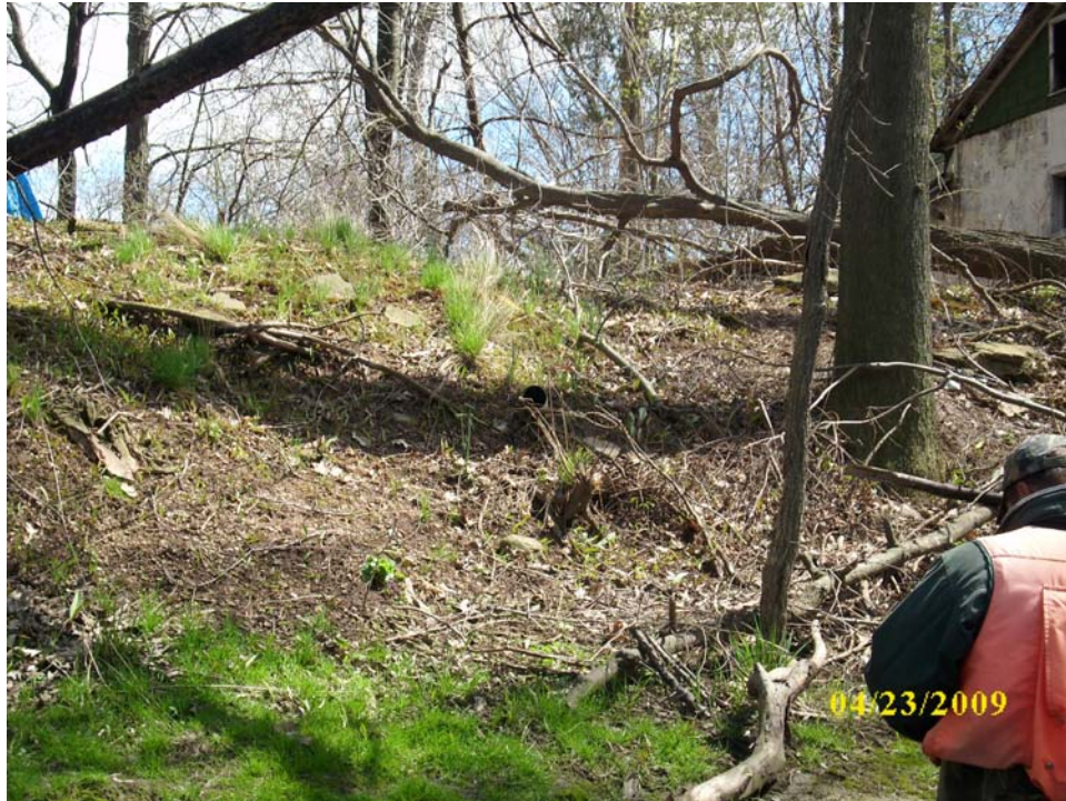
Photo: P43 Direction of view: SE Description: PVC pipe outfall along RDB (OUT-020).
