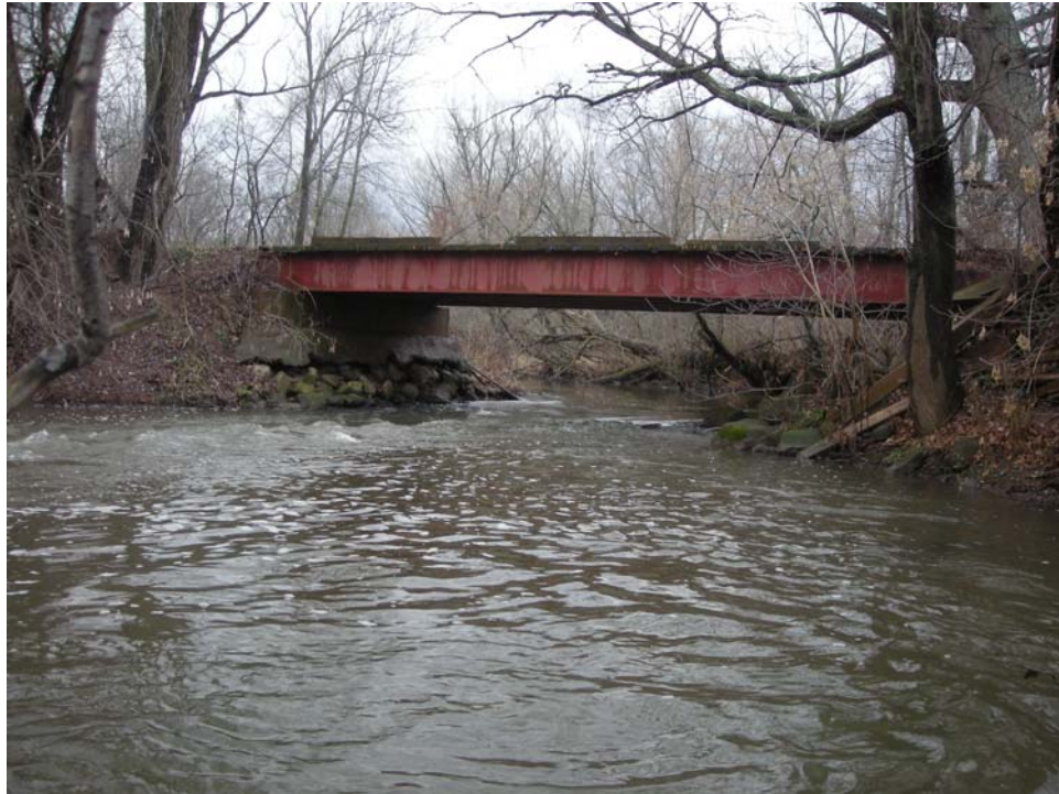
Photo: P27A Direction of view: S Description: Farm bridge #3 from mid-channel.
