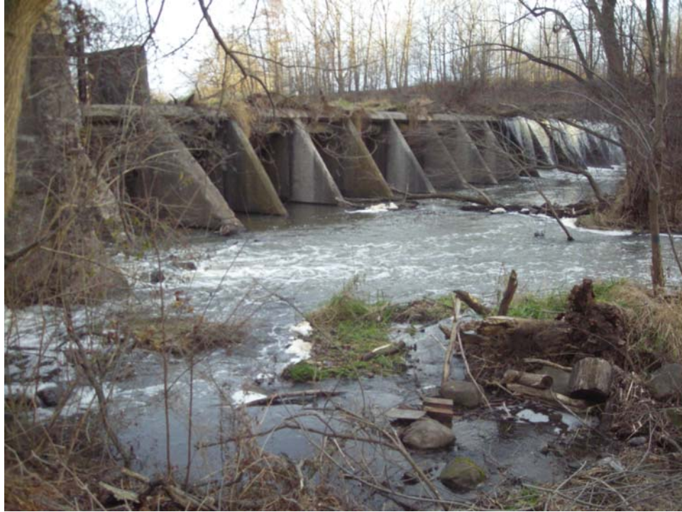
Photo: P74A Direction of view: SW Description: Newfane Dam spillway.
