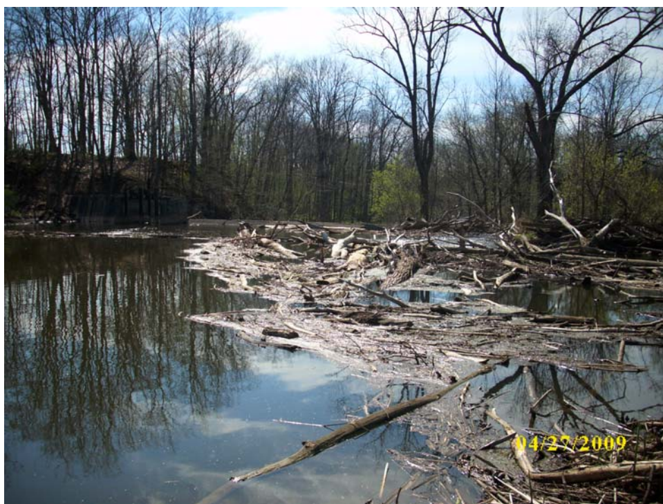
Photo: P80b Direction of view: SW Description: View immediately upstream of Newfane Dam.
