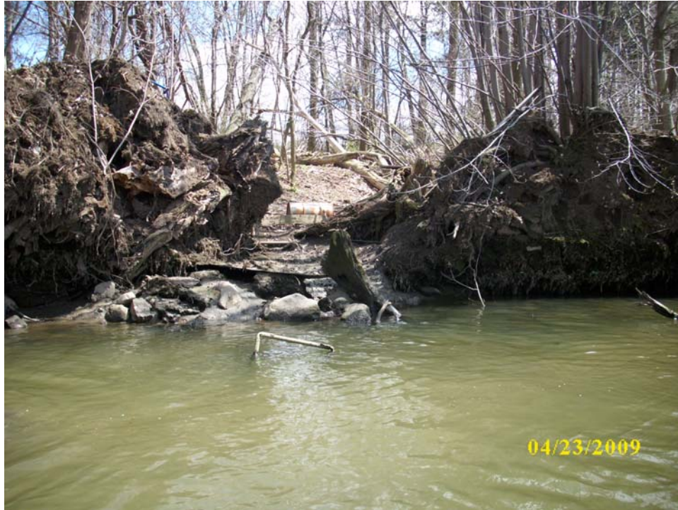
Photo: P42 Direction of view: SE Description: Overland drainage along RDB.
