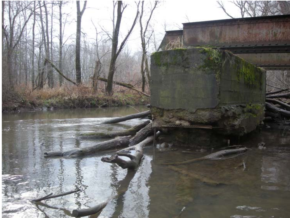
Photo: P24A Direction of view: SE Description: Farm bridge #2 from RDB.
