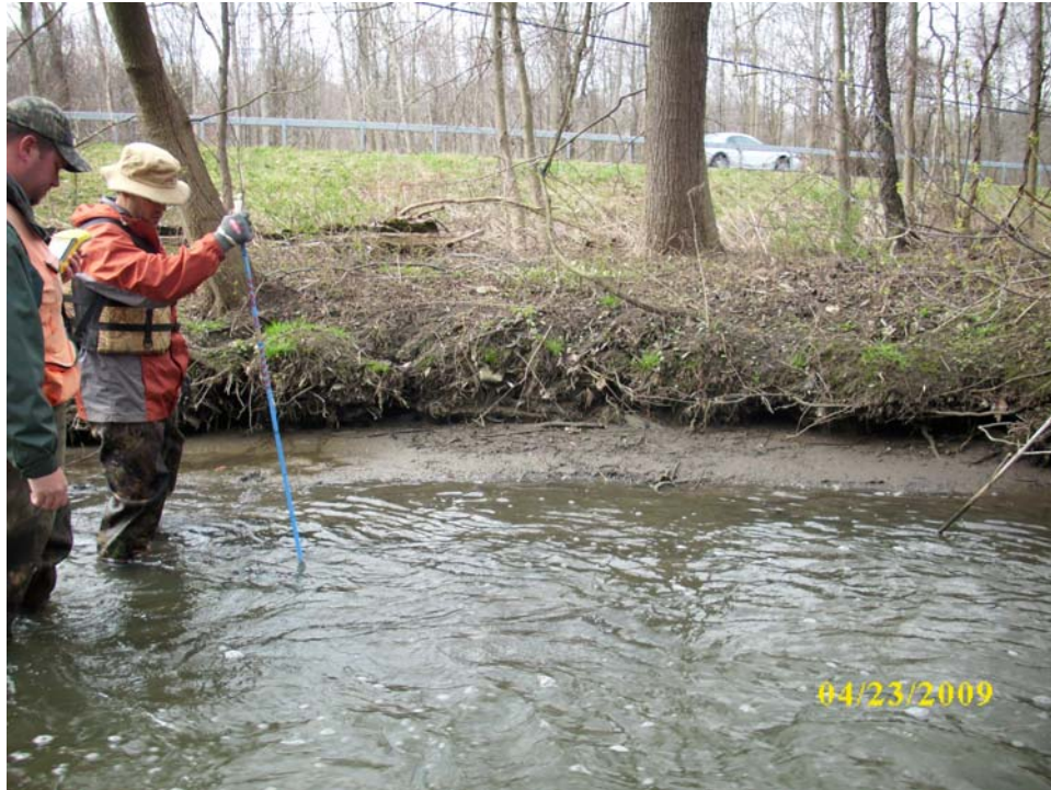
Photo: P23 Direction of view: SW Description: Sediment deposit along LDB.
