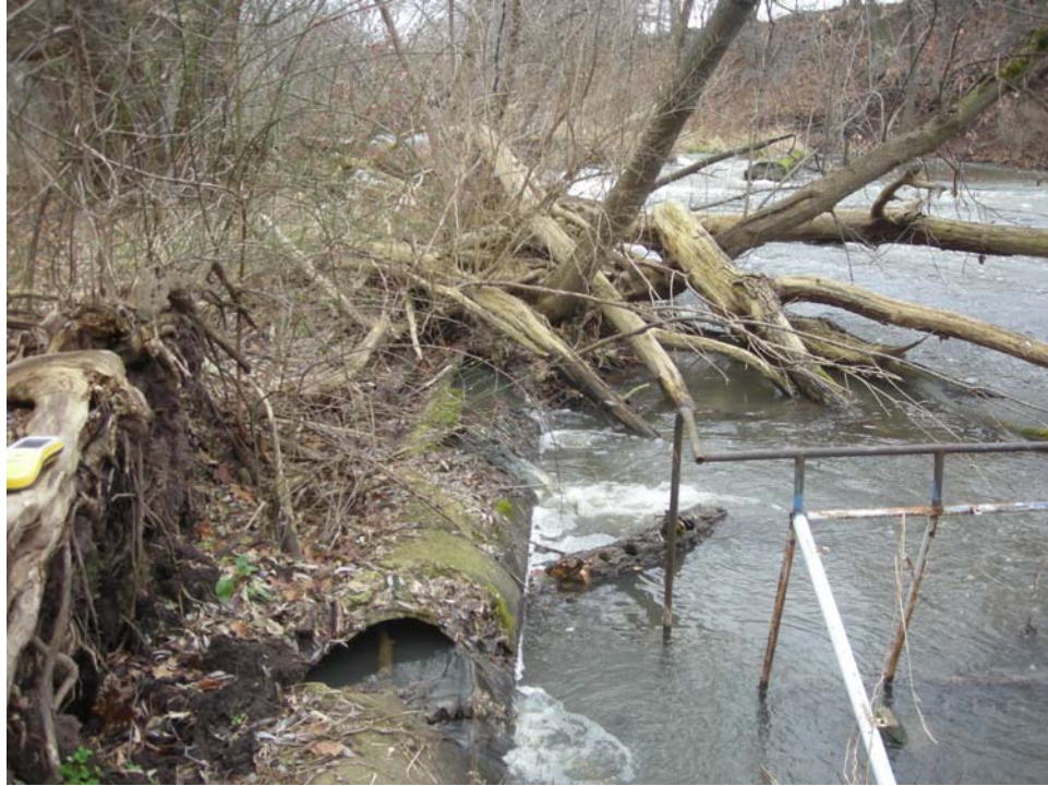
Photo: P54A Direction of view: SW Description: Intake culvert along RDB.
