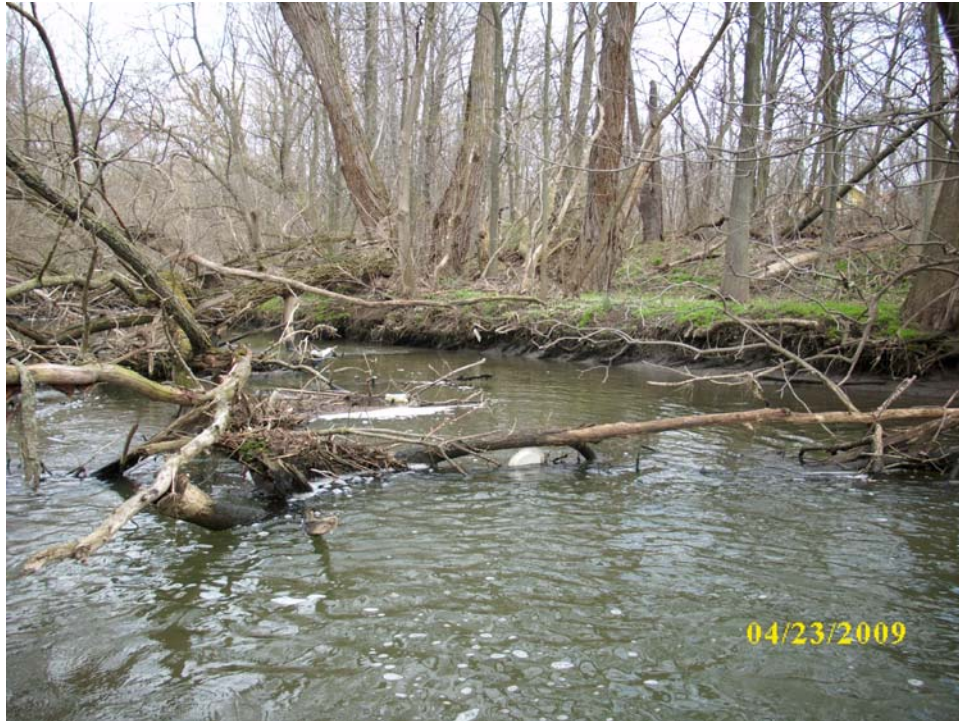
Photo: P25 Direction of view: NE Description: LWD obstruction across creek and terrace along RDB (OBS-020).
