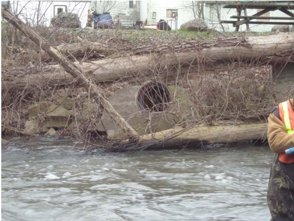
Photo: P57A Direction of view: E Description: Section of concrete culvert on RDB.
