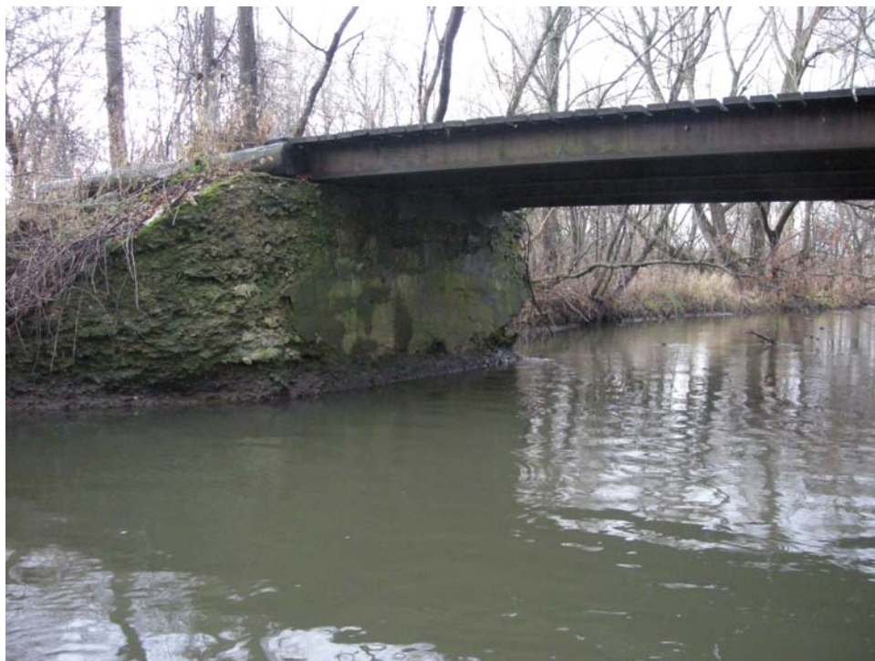
Photo: P22A Direction of view: SE Description: Farm bridge #1 from RDB.
