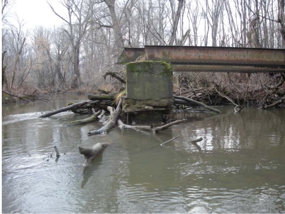
Photo: P26A Direction of view: S Description: Farm bridge #2 from mid-channel.
