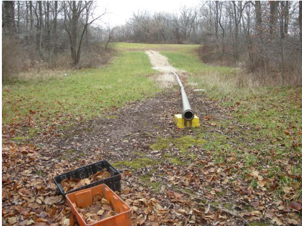
Photo: P61A Direction of view: W Description: Irrigation section along LDB.
