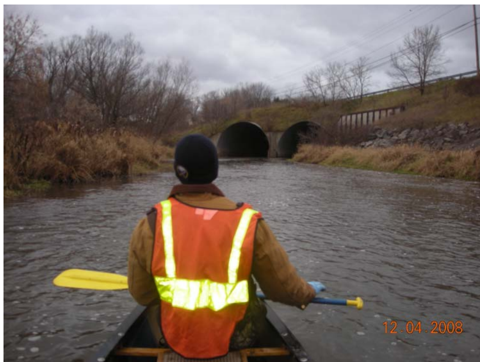
Photo: P72A Direction of view: N Description: Entering the culverts at Ide Road.
