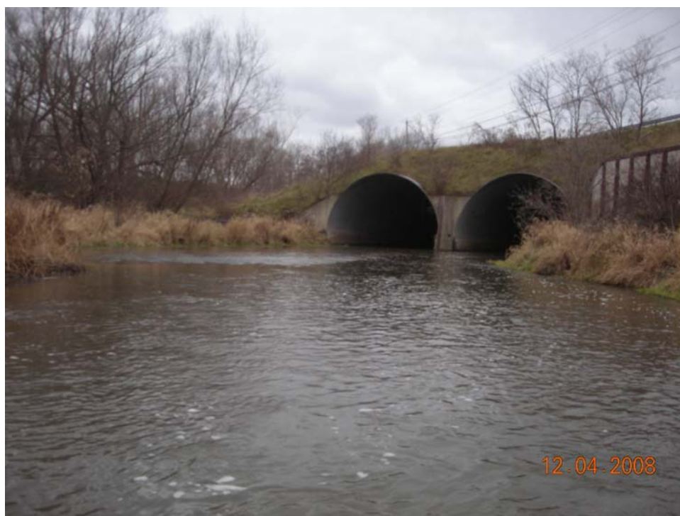
Photo: P73A Direction of view: N Description: View of Ide Road crossing and culverts.
