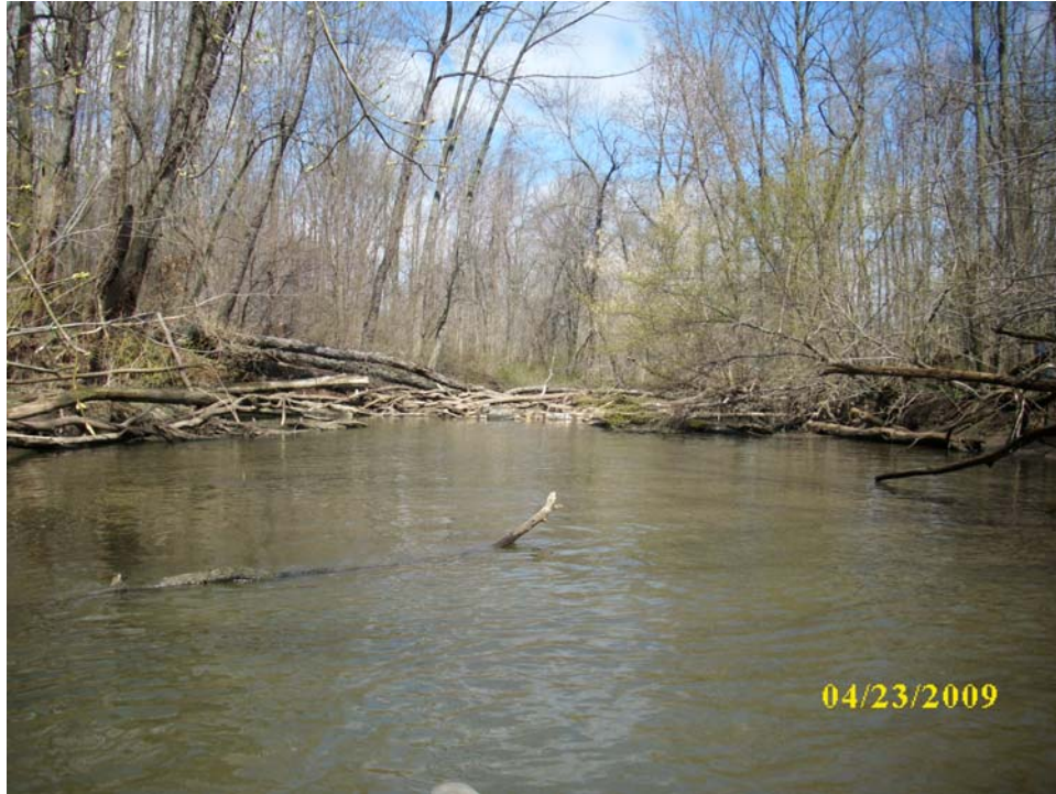
Photo: P36 Direction of view: N Description: LWD obstruction across creek (OBS-025).
