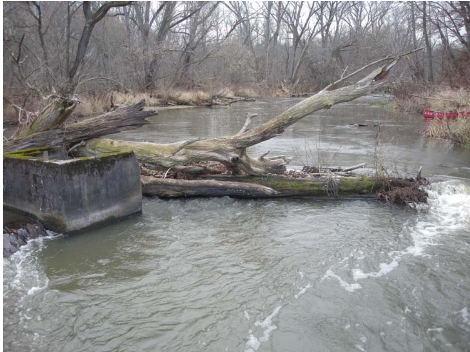
Photo: P53A Direction of view: S Description: Intake culvert in mid-channel.
