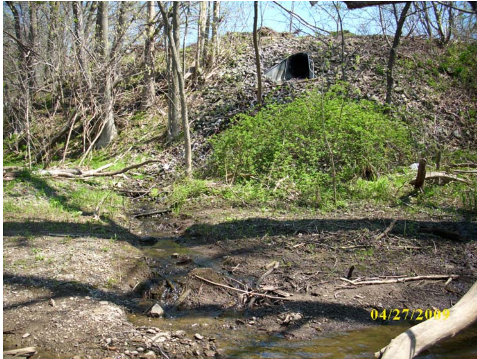
Photo: P73 Direction of view: NE Description: Culvert with run-off flowing to creek (OUT-025).
