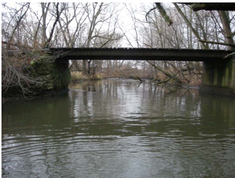
Photo: P23A Direction of view: S Description: Farm bridge #1 from mid-channel.
