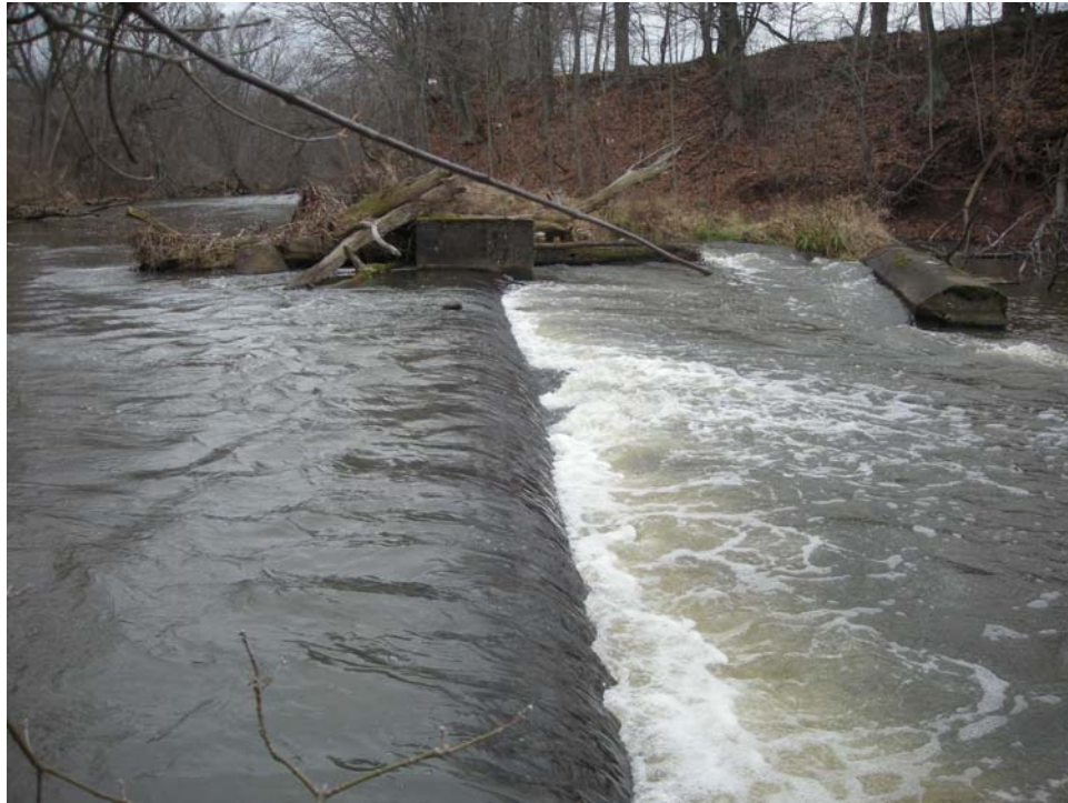
Photo: P55A Direction of view: SW Description: Intake culvert in mid-channel.
