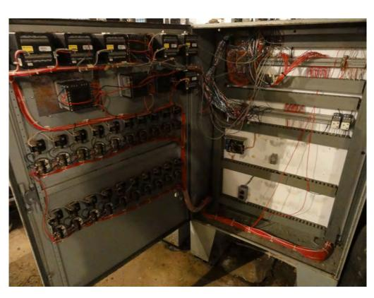
View of interior of GWET system control panel. Note absence of PLC within control panel.
