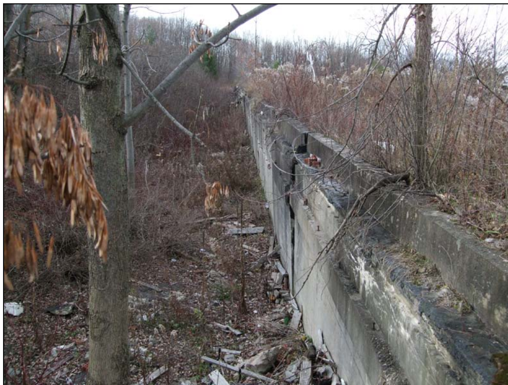
M-4. Known-distance range concrete target butt. Some frames for moving the targets up and down have been removed. Bullets impacted to the left.
