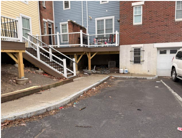
Photo #7 Additional photo from underneath deck
