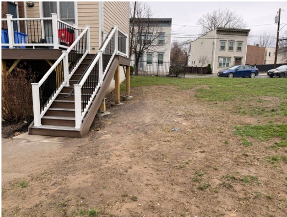
Photo #9 Interior lawn area, showing slight erosion facing Northwest
