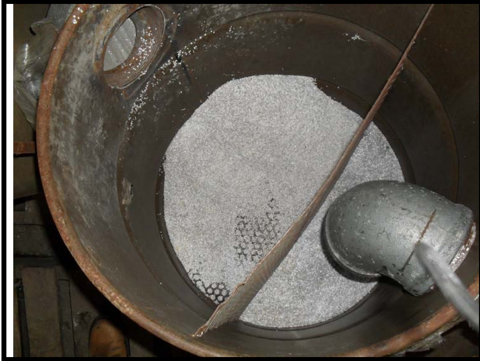
Building 1 Basement, Room 003 - Drum of Unknown Substance.
