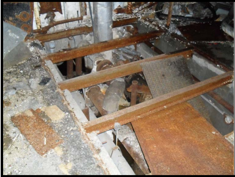
Building 17 Coating Alley – Sump/Pipe Chase.
