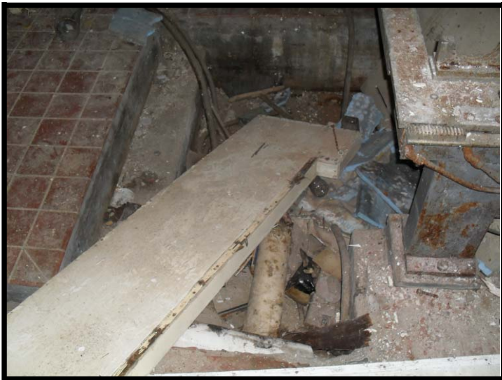
Building 7 Coating Alley – Sump/Pipe Chase.
