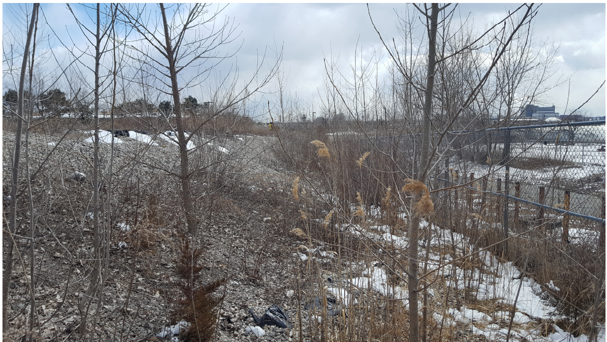
Photograph #6 – Cover material (crushed stone) on west side of Primary Remediation Area, facing south. Barretto Street on right, beyond fence.
