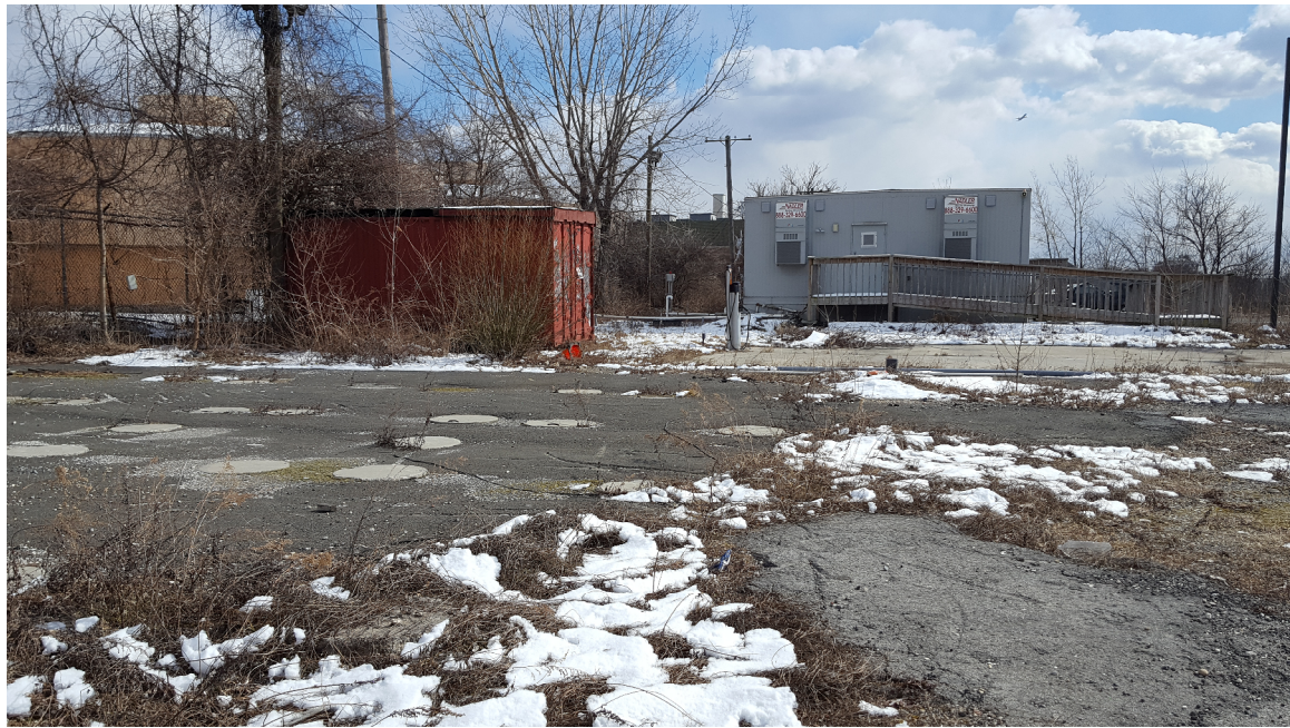
Photograph #18 – Paved area north of construction trailers. Concrete disks appear to be part of foundation for previously existing building.
