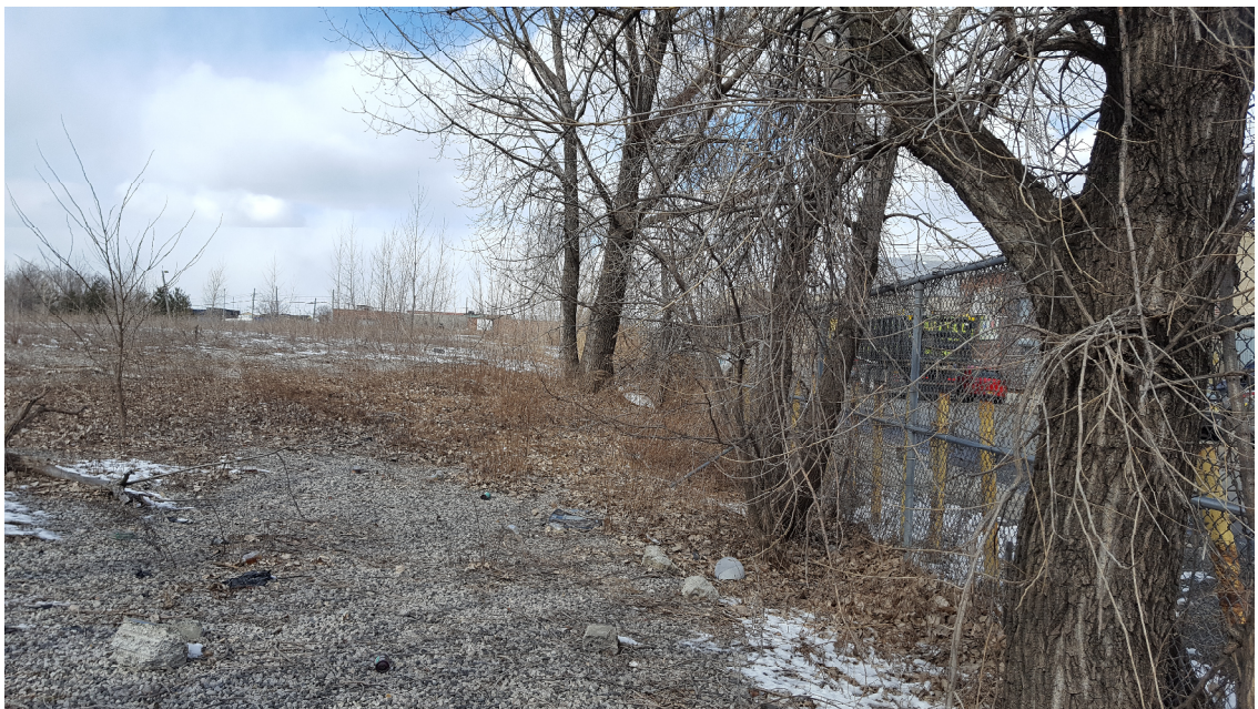
Photograph #8 - Cover material (crushed stone) on east side of Primary Remediation Area, facing north. Manida Street on right, beyond fence.
