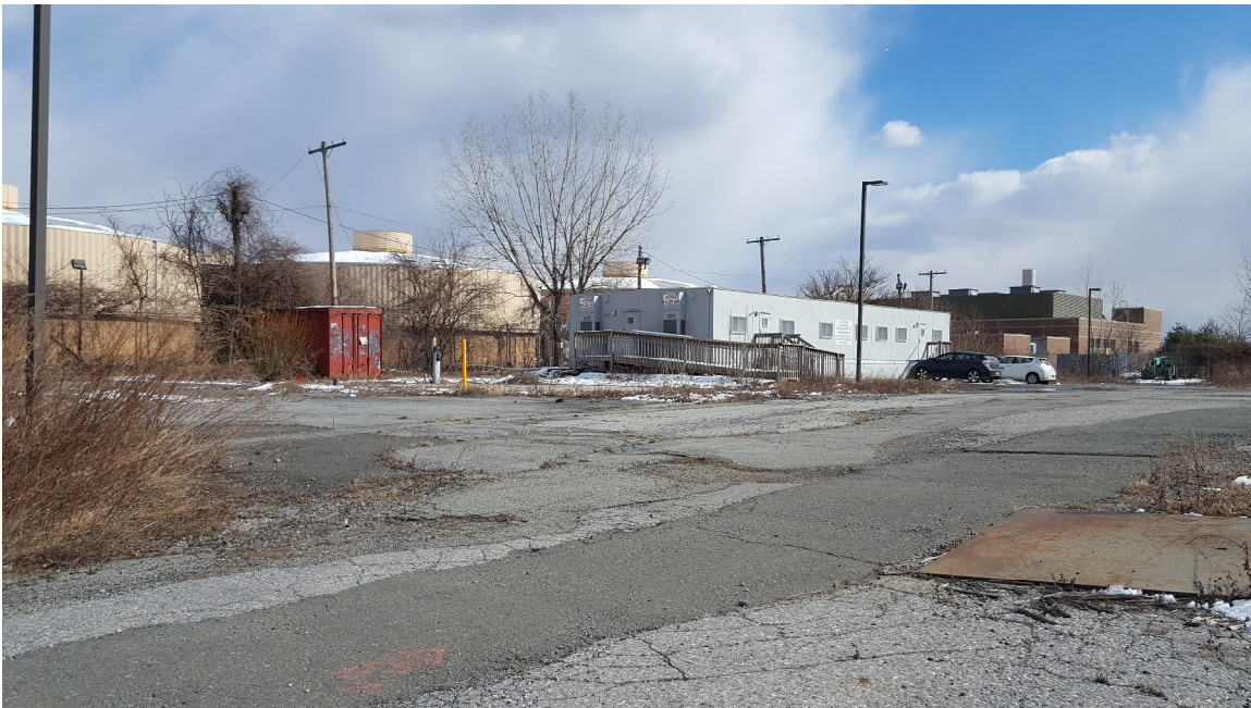
Photograph #14 – View of construction trailers, facing southeast. Sludge thickeners to left, east of offices.
