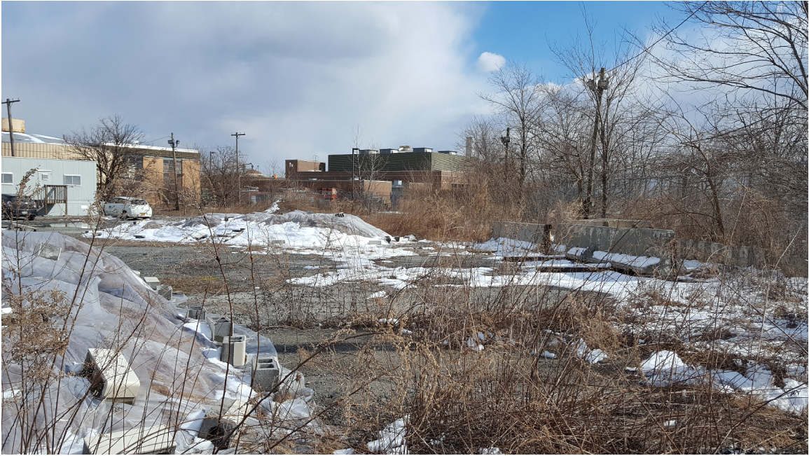
Photograph #15 – Area west of construction trailers, facing south. Two tarped stockpiles of mulch (wood chips). East River to right.
