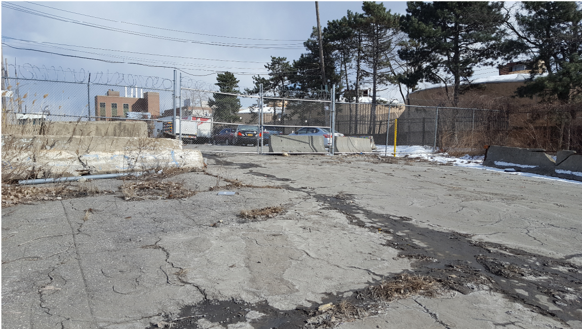
Photograph #11 – View of Site entrance at Ryawa Avenue, facing east. Sludge thickeners to right.
