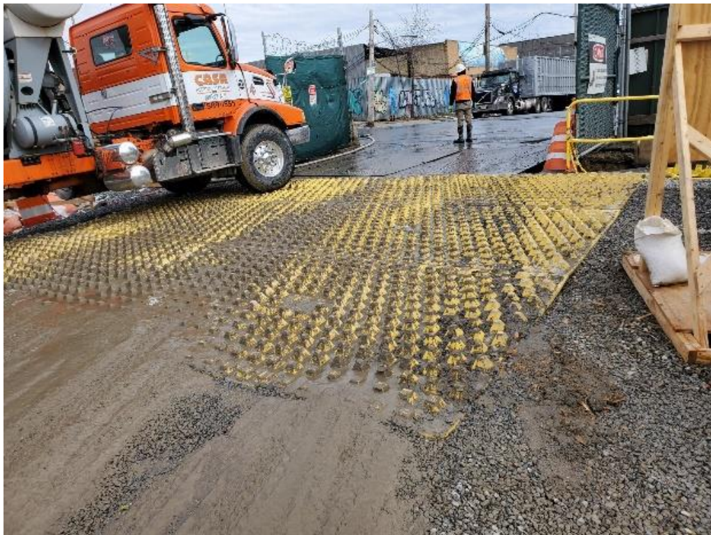
Photo 8 - Site entrance south of 2.5acre BUD area looking east. Rumble pad and washing operation in place.
