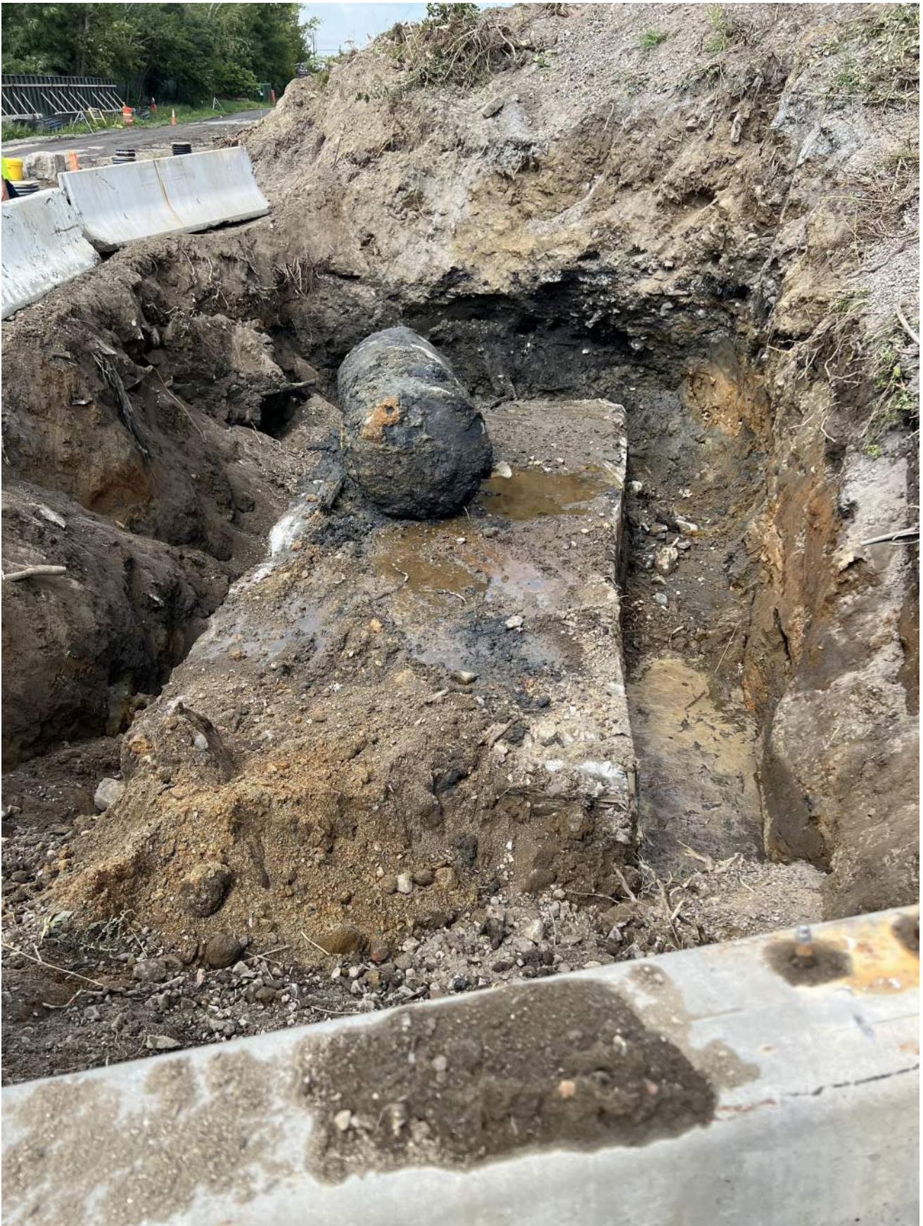
Attachment B Uncovered 550 gallon UST and concrete partially encasing 5 additional 550 gallon USTs.
