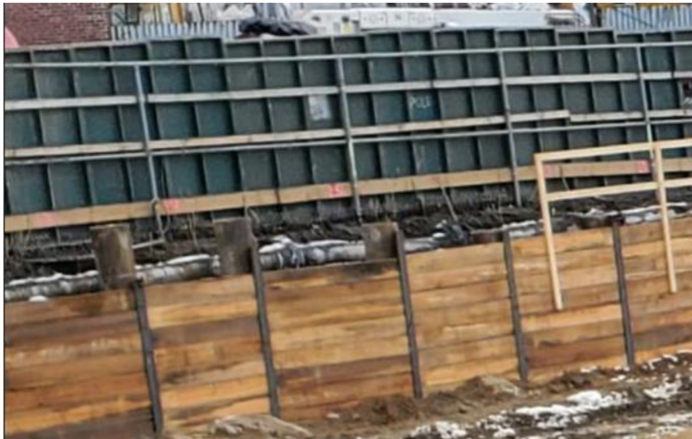
East perimeter fence and lagging
