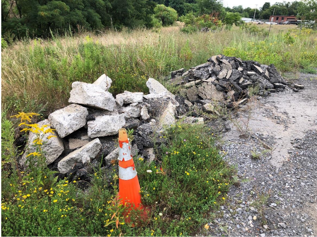
Photograph 1 – Settling of the former foundation north of the existing building
