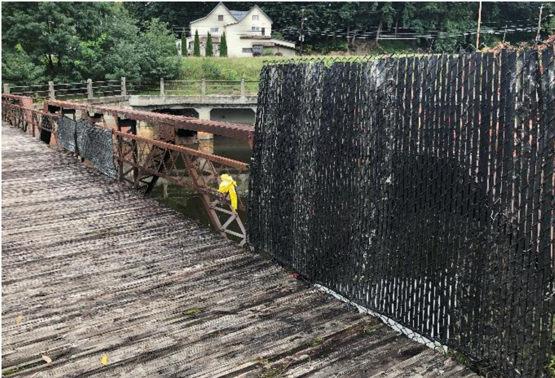
Photograph 4A – Repairs to the missing side rails on the footbridge
