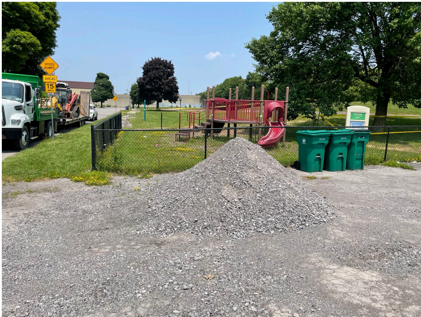
Imported crusher run for future impervious surface work subbase.
