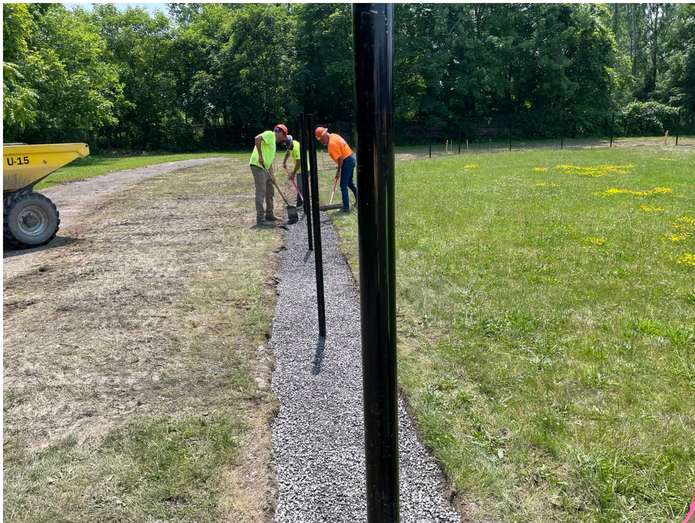
Backfilling fence trench with No.1 stone.
