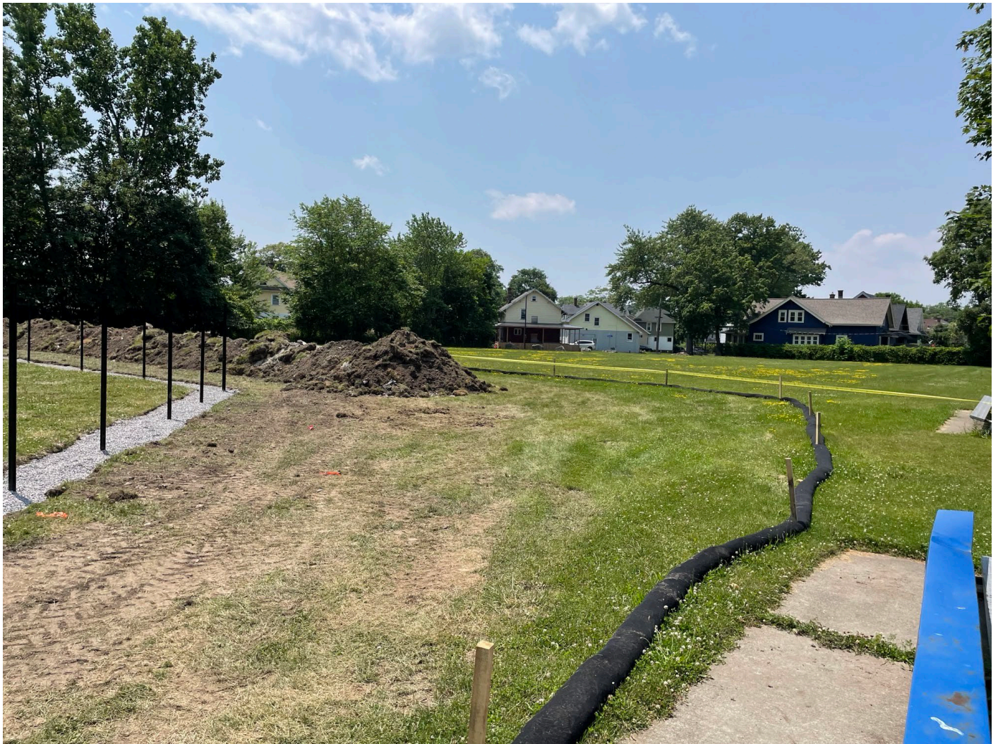
Berm of excavated materials/ perimeter silt sock.
