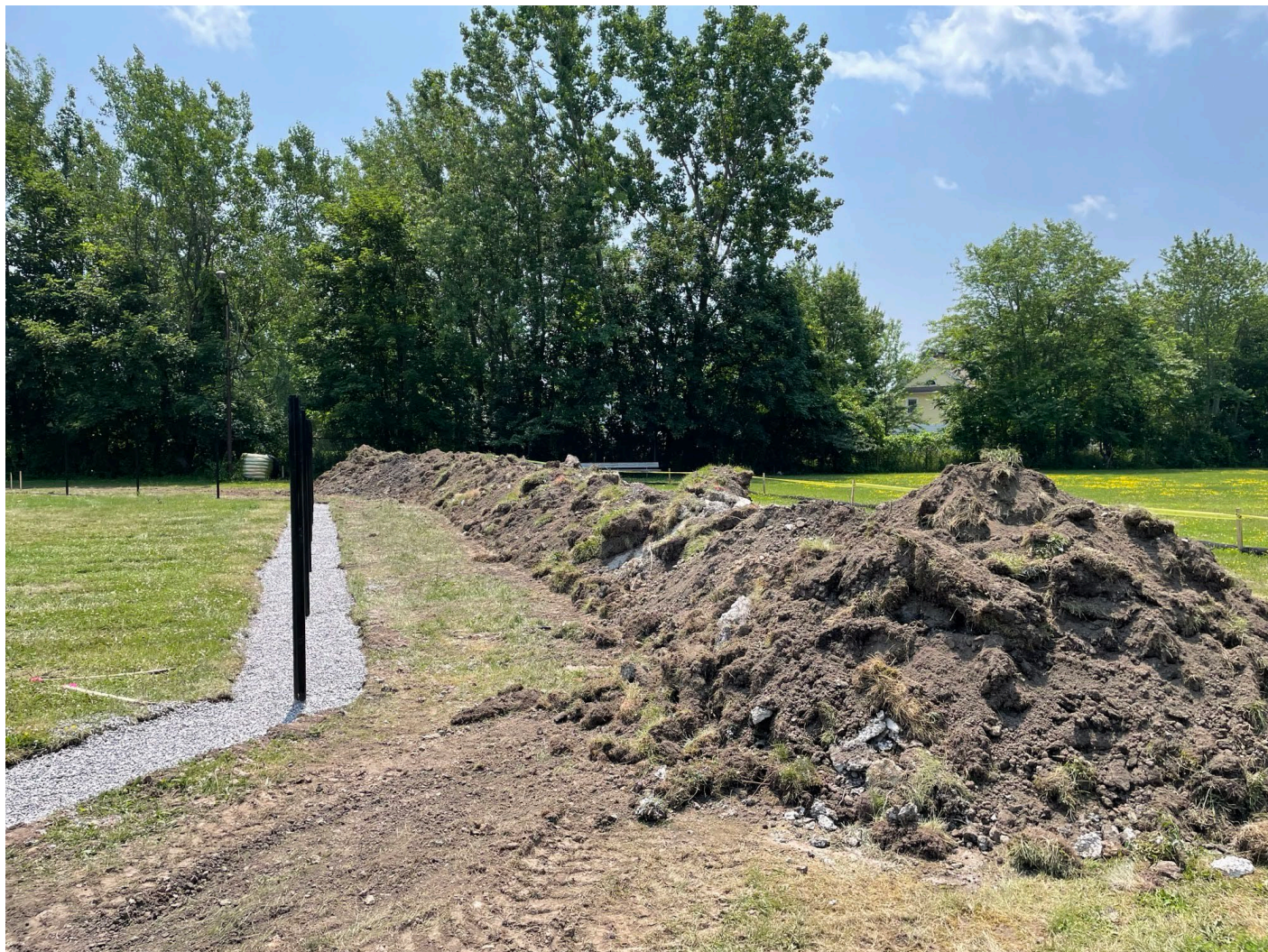
Berm of excavated materials.
