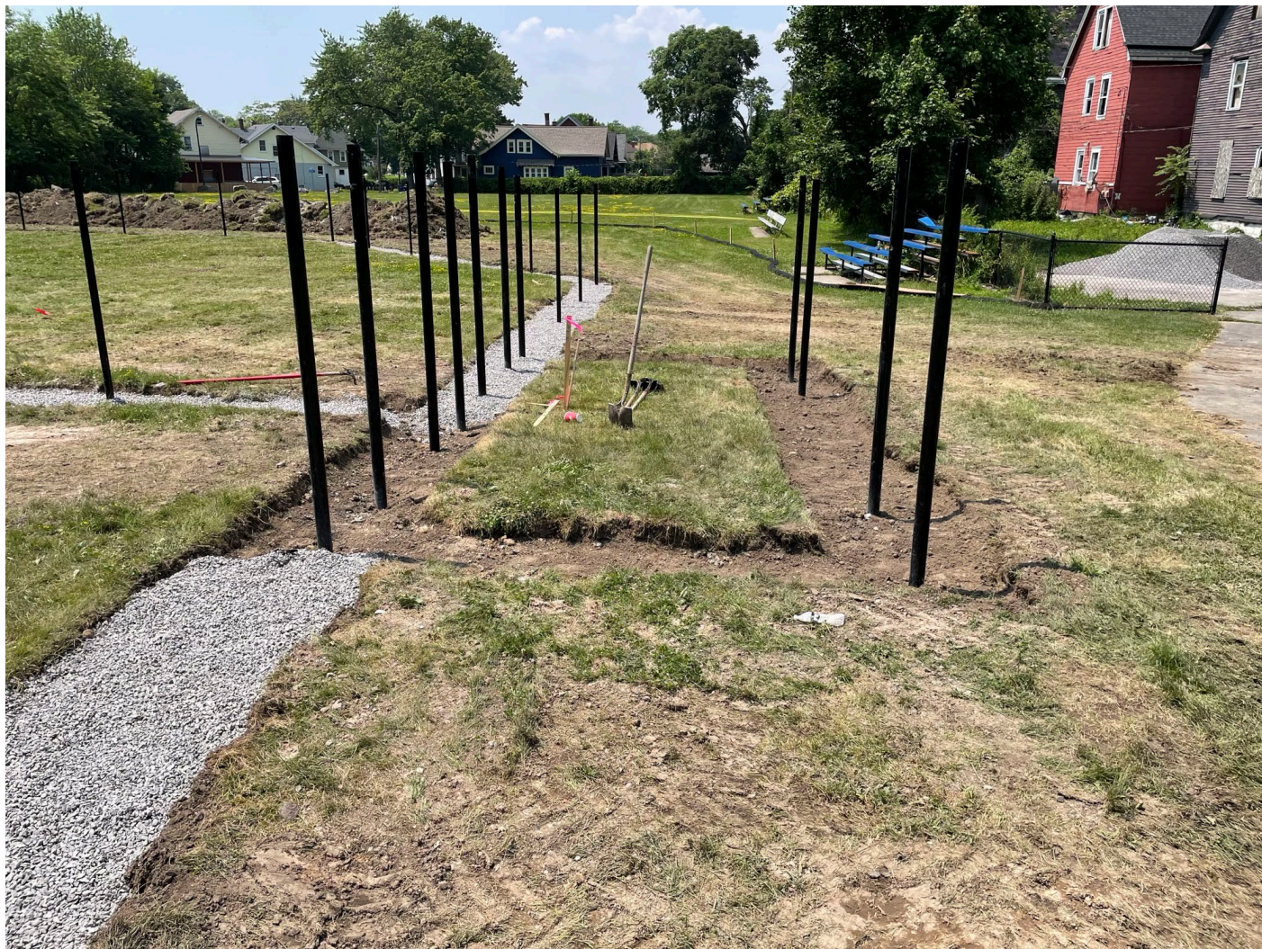
Fence trench/partial backfill.
