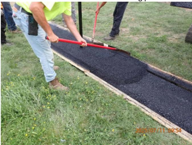
Placing the asphalt for the vegetative control strip.
