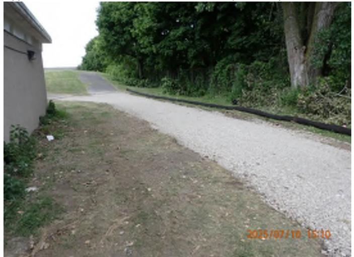
Subbase for the asphalt trail on east side of shelter house.
