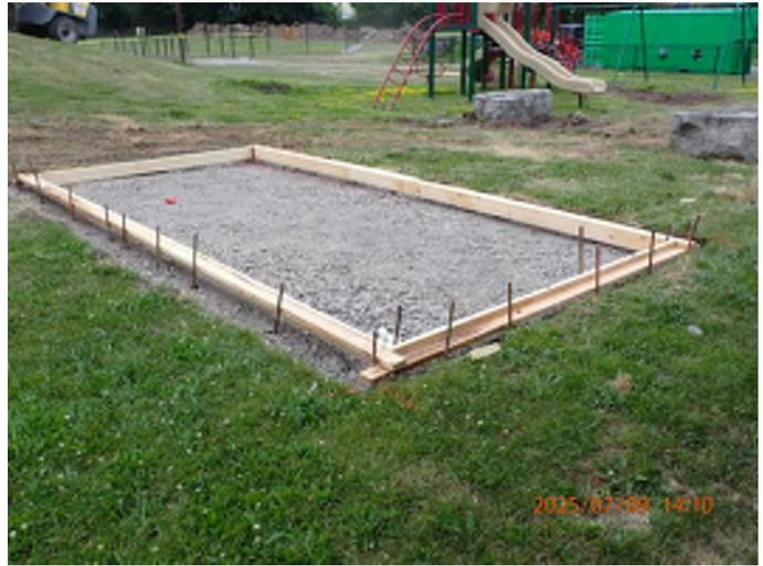
Typ. form work and base for concrete pad for picnic table.
