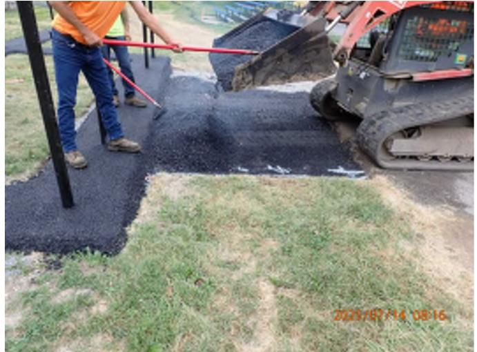
Placement of asphalt on the north side of dog park fence.
