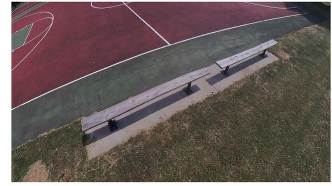
NOTE: REPLACE EXISTING WOODEN PLANK WITH PRESSURE TREATED PLANK OF NOMINAL SIZE TO MAINTAIN EXISTING DIMENSIONS. PROVIDE NEW MOUNTING HARDWARE FOR CONNECTION TO EXISTING METAL POSTS TO REMAIN
