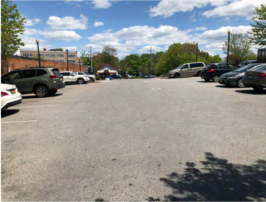
5. Cover system at northernmost portion of property
