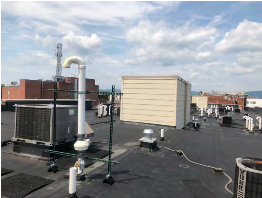
6. One of three discharge points on roof
