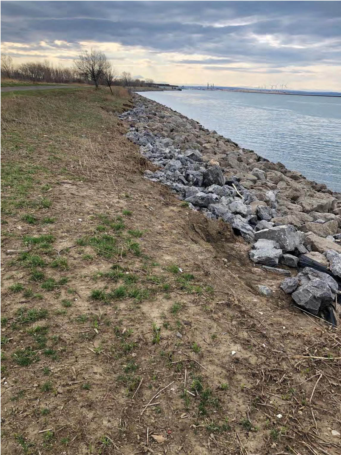
View of medium stone placed behind the armor stone.
