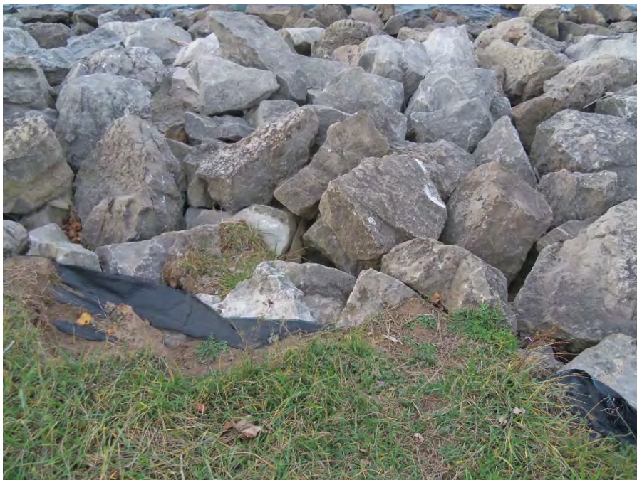
View of exposed geotextile located approximately midway between Bell Slip and north end of Greenbelt.
