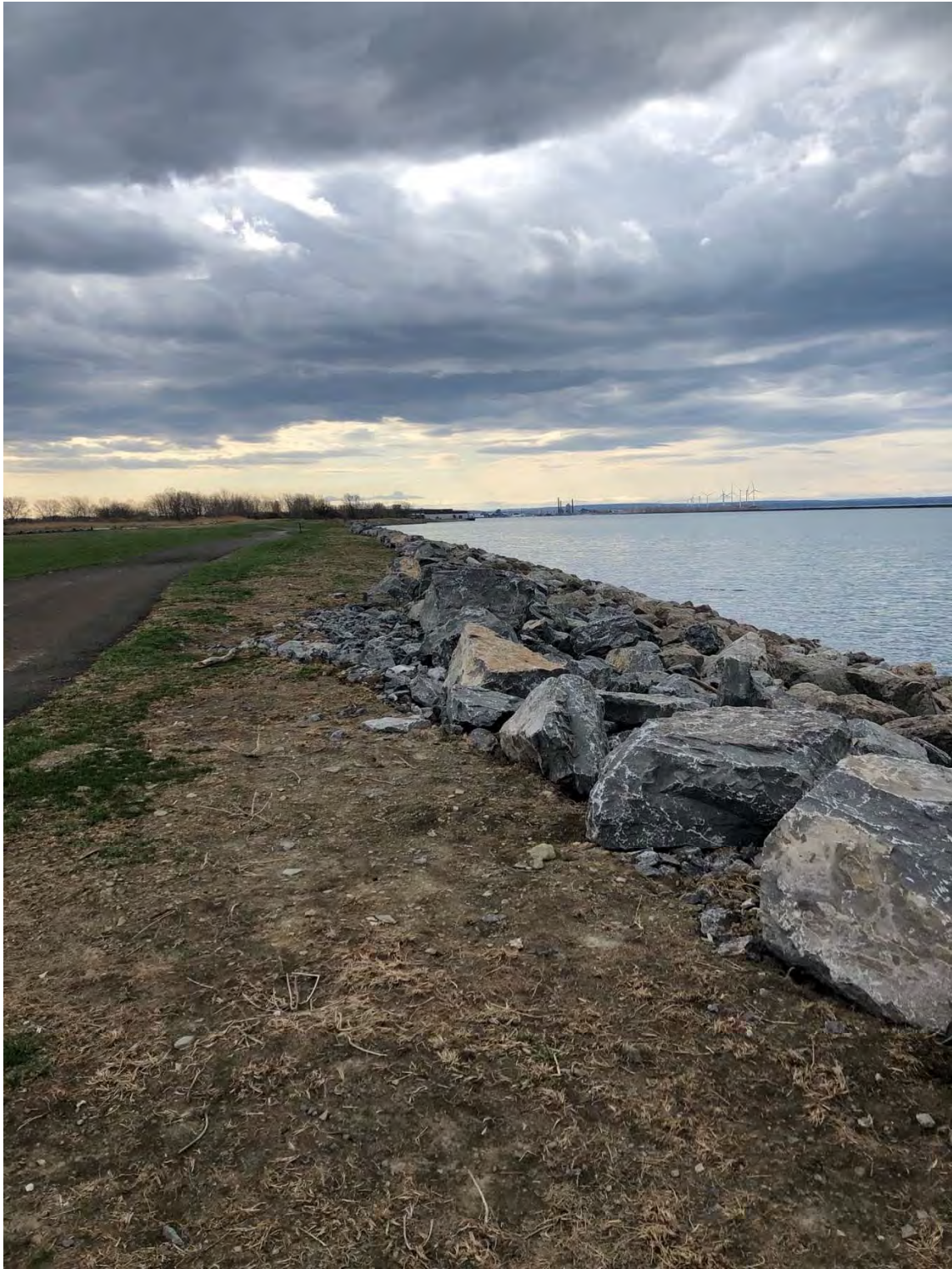
View of new armor stone placed at the top of the bank.
