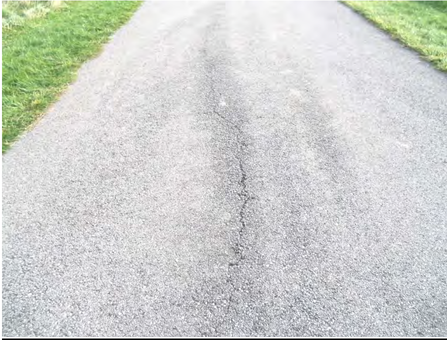
View of crack in asphalt in section of path along the south side of Bell Slip.
