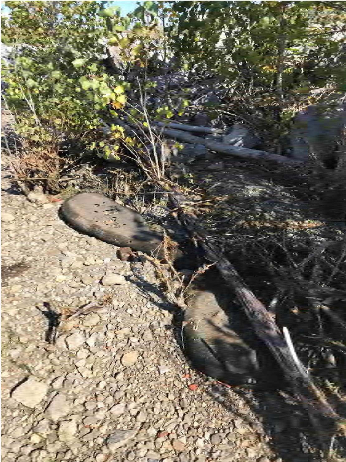
Exposed toe sock and netting along east shoreline of Bell Slip.
