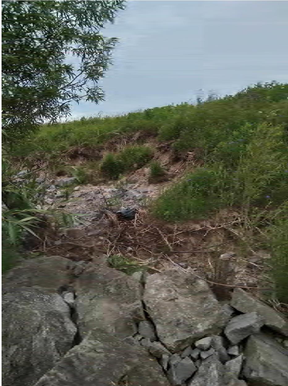
Photo No. 7 – Stump left behind following tree removal by beavers and damage to embankment. North side of Bell Slip.
