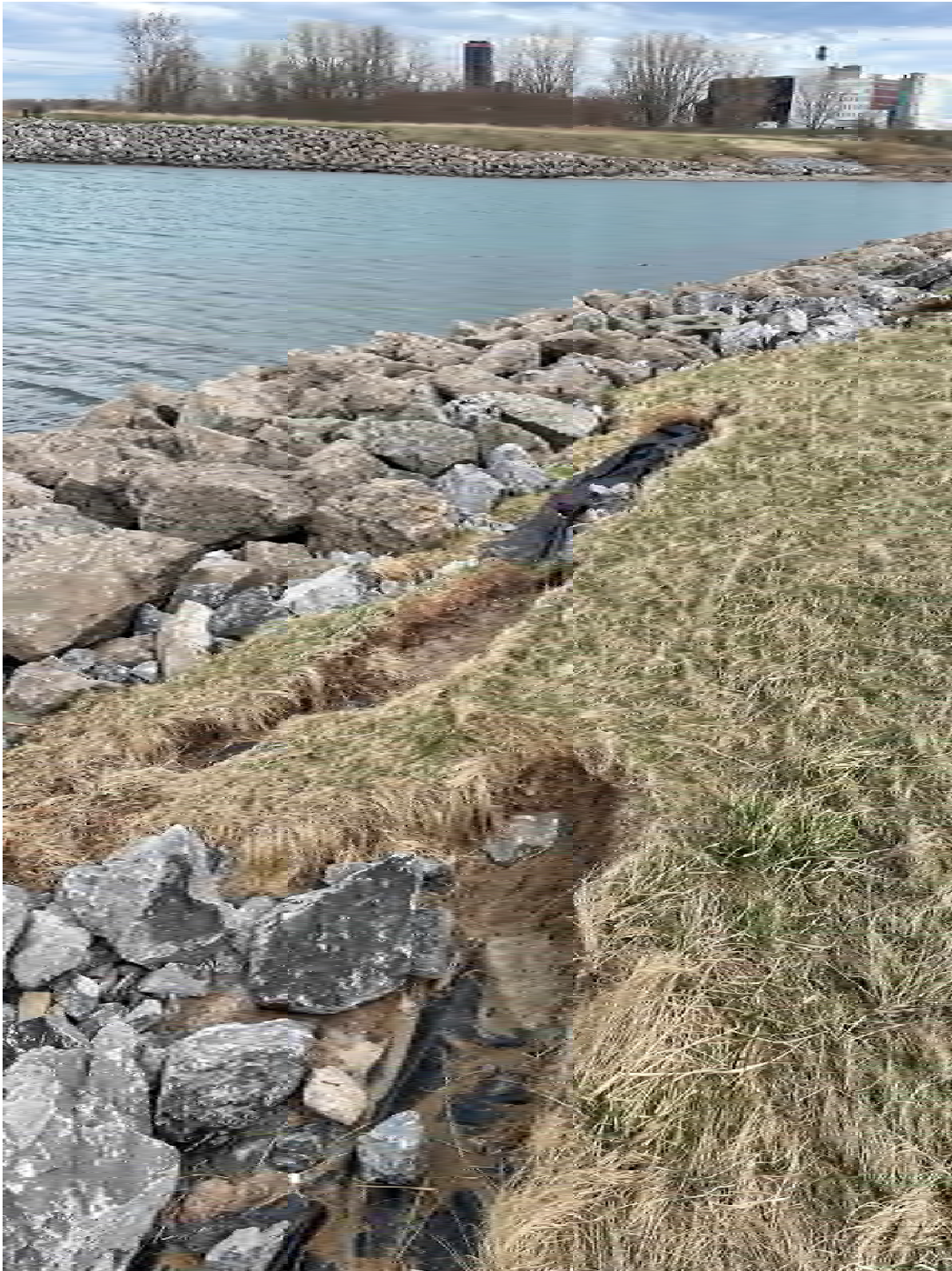
View of bank erosion on South side of Bell Slip, view looking towards the east.
