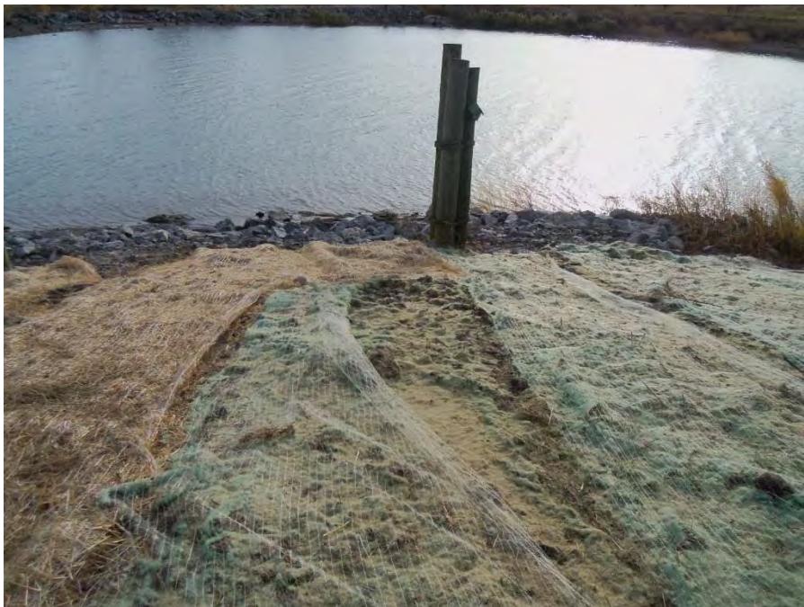
View of new netting installed in 2020 in a portion of the south side of Bell Slip.
