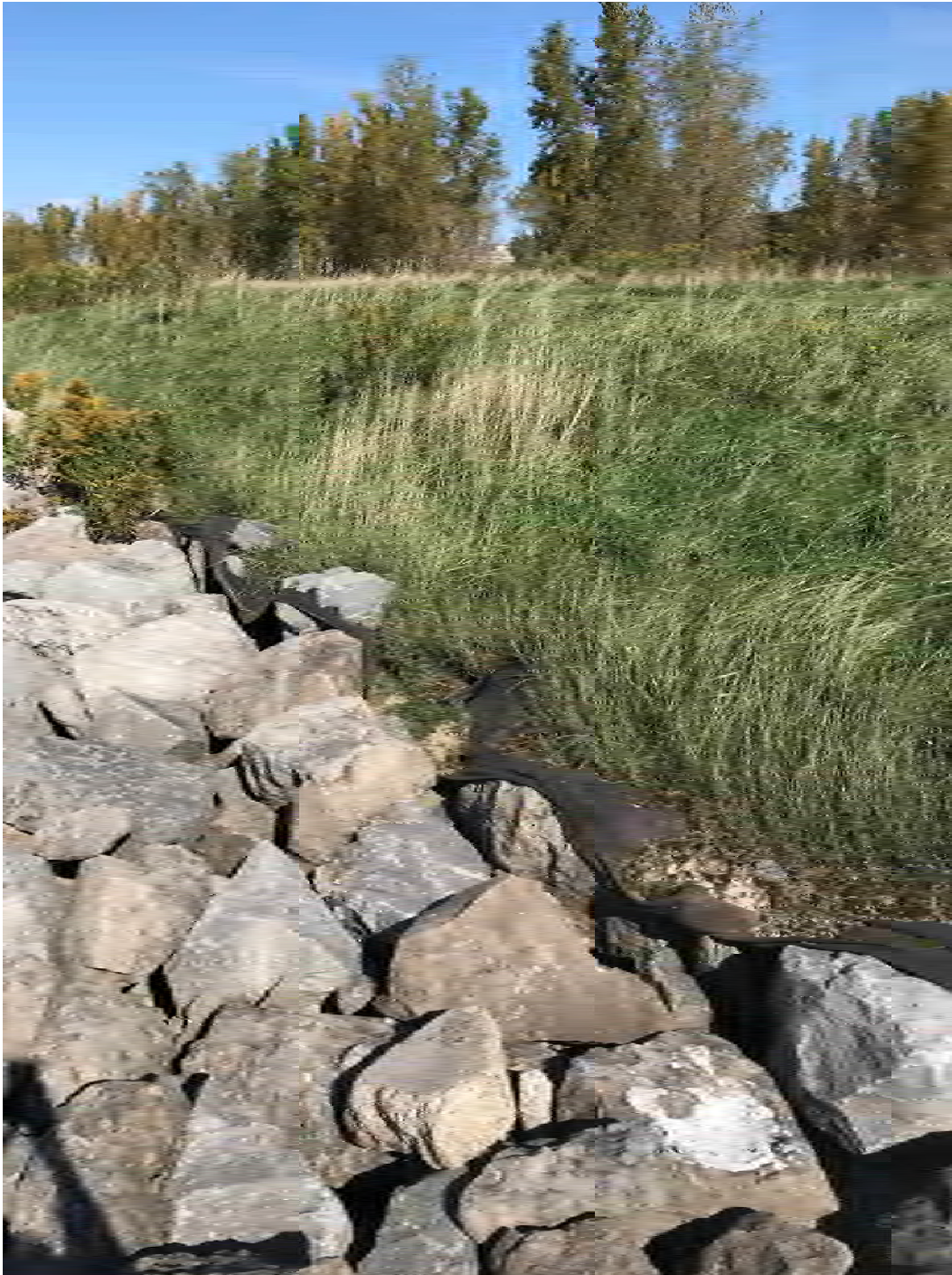
View of exposed geotextile between revetment and soil cover system.
