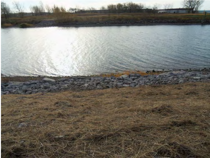
View of new revetment installed in 2020 in a portion of the south side of Bell Slip.
