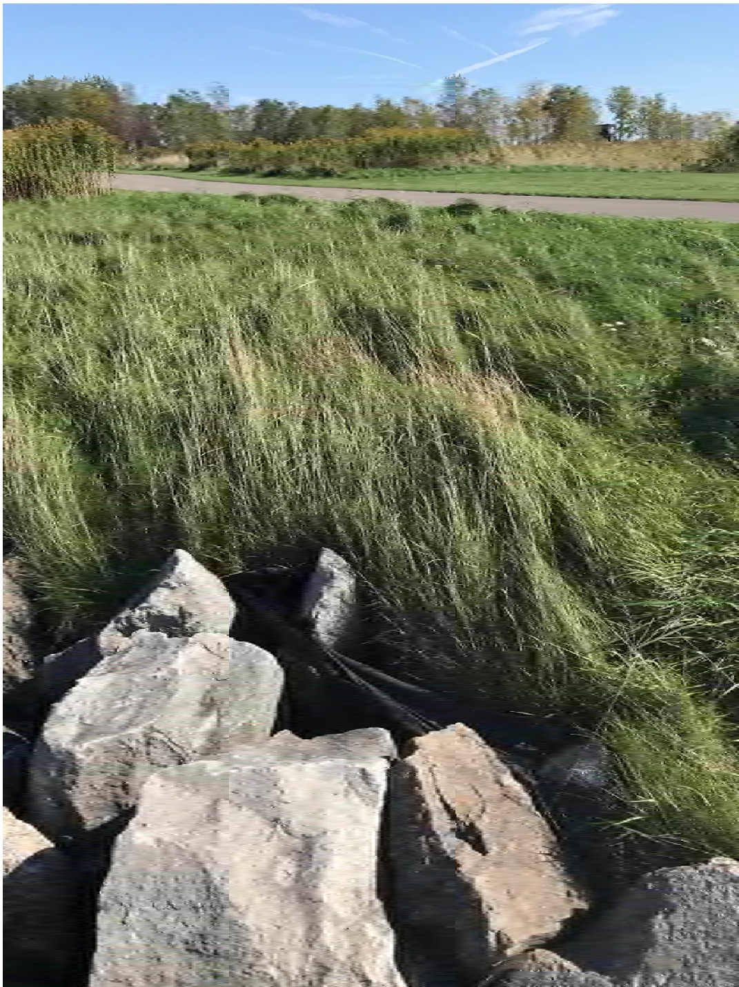
Area of exposed geotextile between revetment and soil cover system, south side of Bell Slip.
