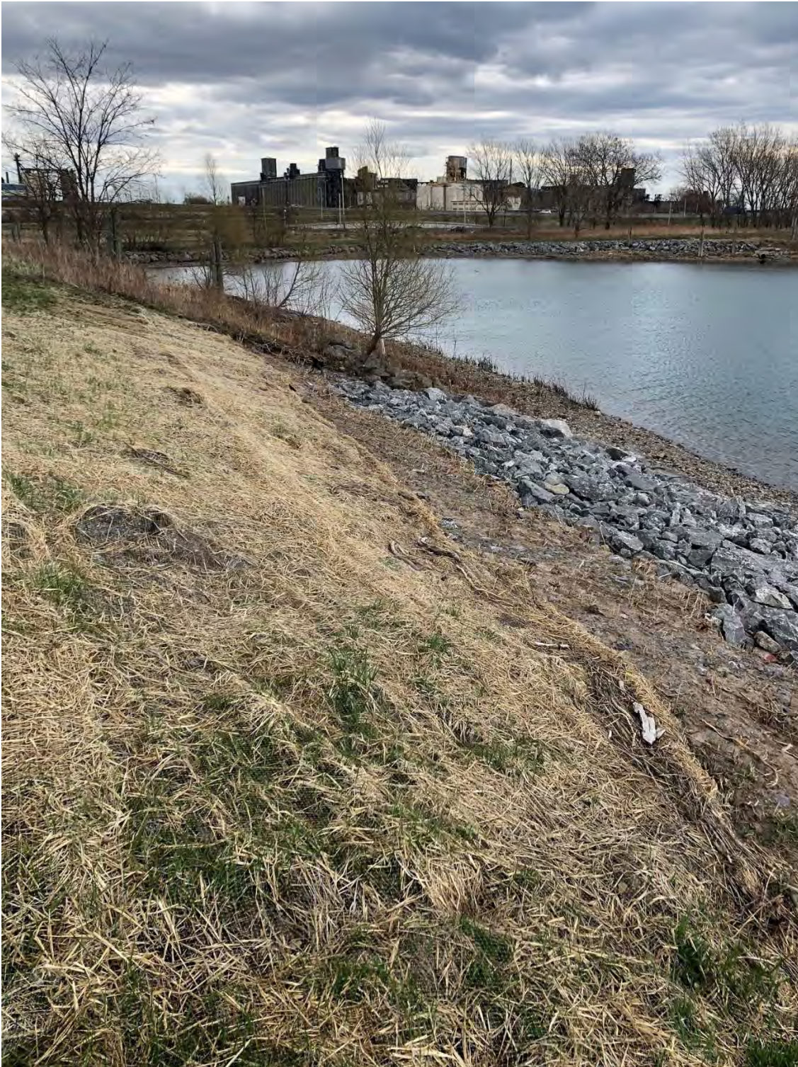
View of erosion control blanket on northern bank slope at Bell Slip.
