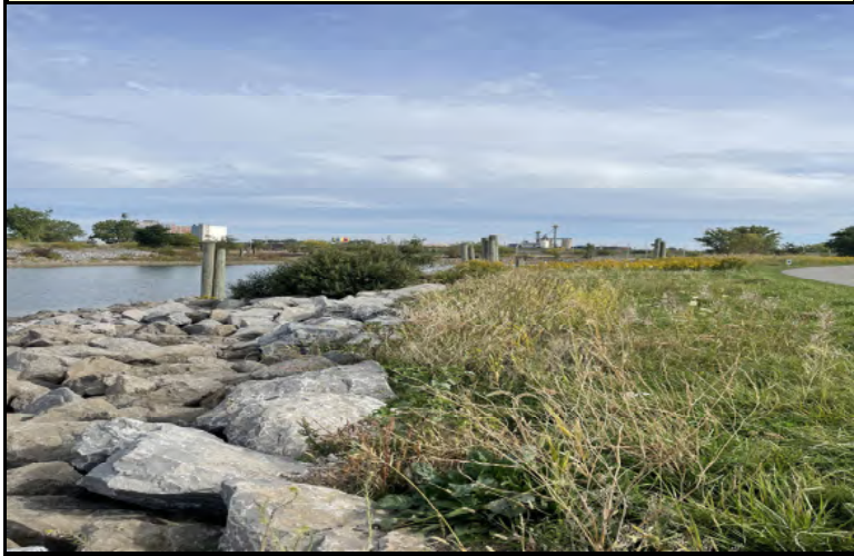
Photo 7: Stabilized shoreline and completed repairs
