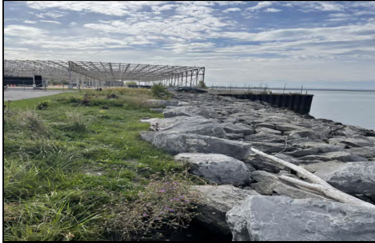
Photo 1: Stabilized shoreline and completed repairs
