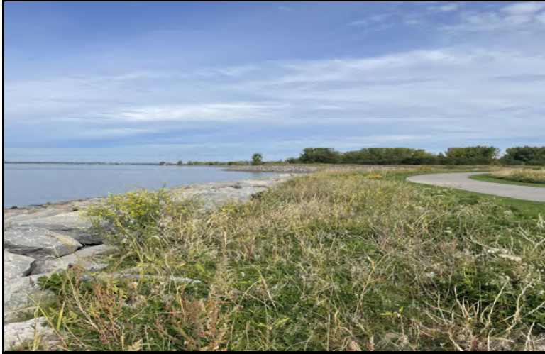
Photo 5: Stabilized shoreline and completed repairs
