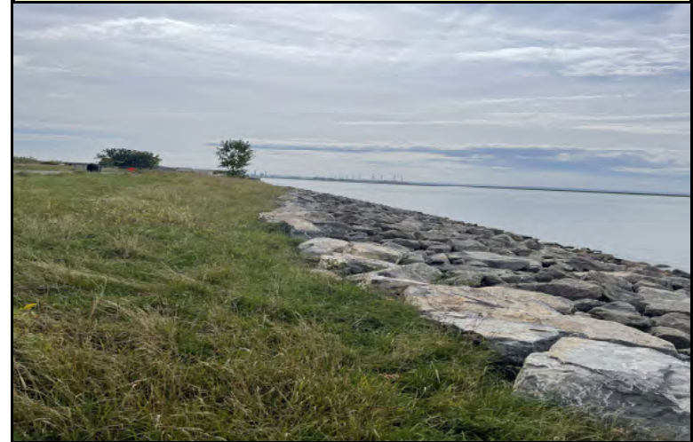
Photo 12: Stabilized shoreline and completed repairs
