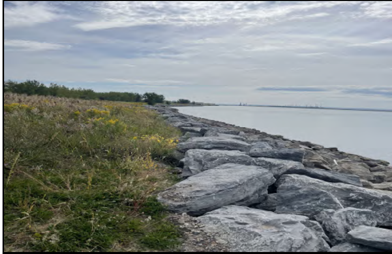
Photo 17: Stabilized shoreline and completed repairs
