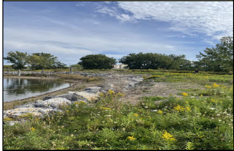
Photo 8: Stabilized shoreline and completed repairs
