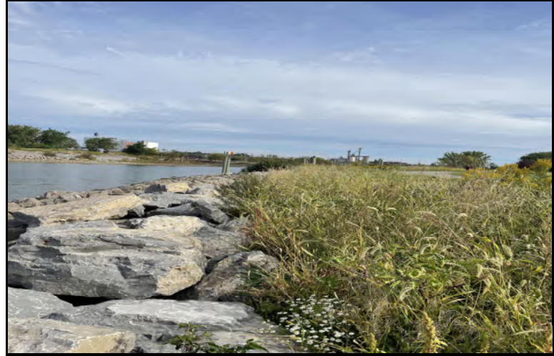
Photo 6: Stabilized shoreline and completed repairs
