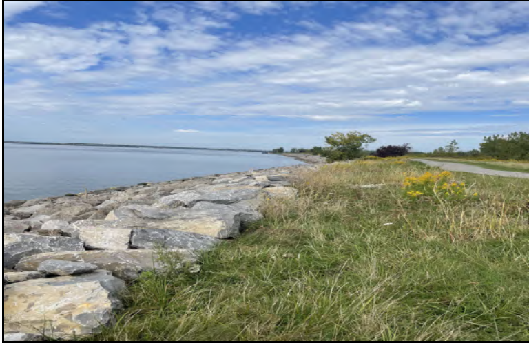
Photo 13: Stabilized shoreline and completed repairs
