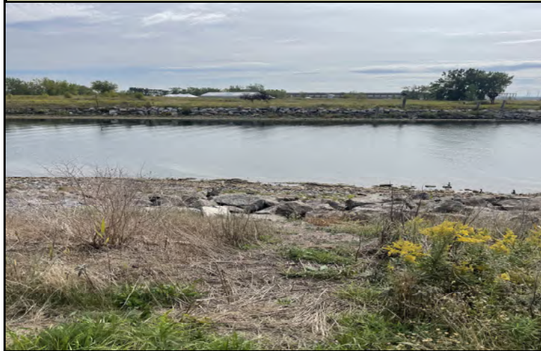
Photo 11: Stabilized shoreline and completed repairs
