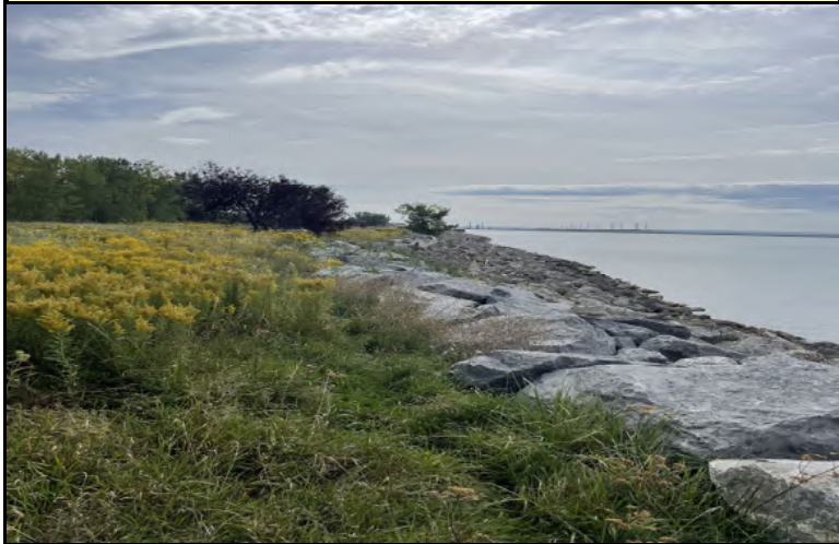
Photo 15: Stabilized shoreline and completed repairs
