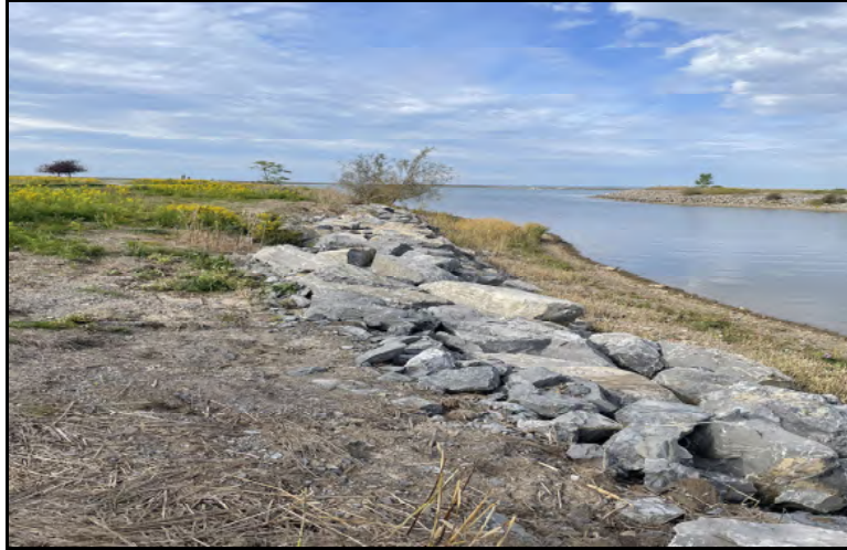
Photo 9: Stabilized shoreline and completed repairs
