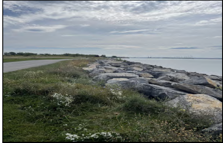
Photo 22: Stabilized shoreline and completed repairs
