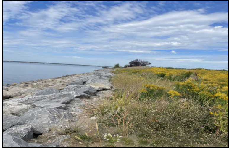
Photo 18: Stabilized shoreline and completed repairs
