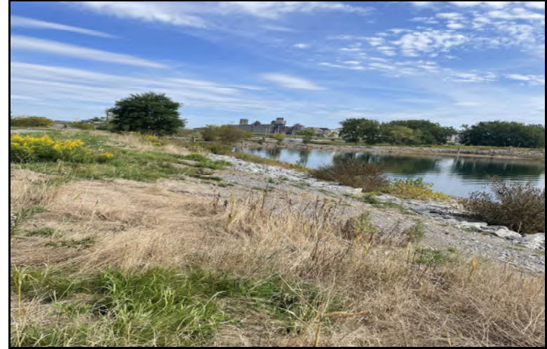
Photo 10: Stabilized shoreline and completed repairs
