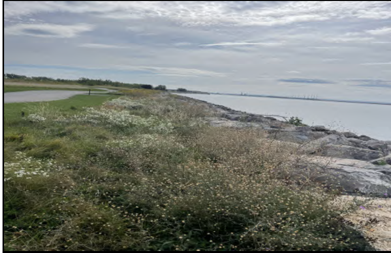
Photo 21: Stabilized shoreline and completed repairs
