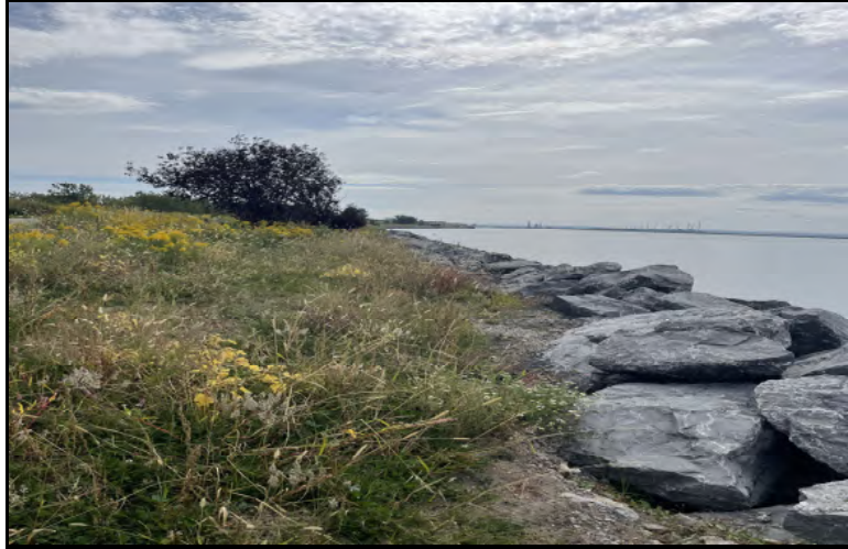
Photo 19: Stabilized shoreline and completed repairs
