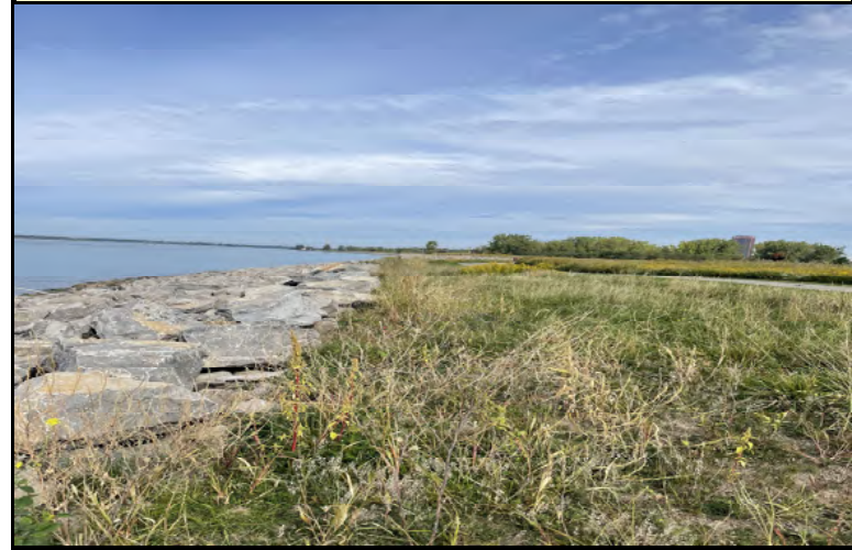
Photo 4: Stabilized shoreline and completed repairs
