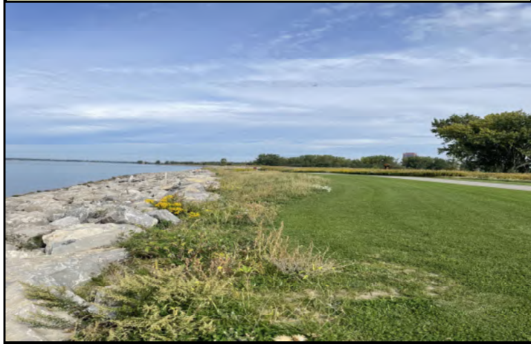
Photo 3: Stabilized shoreline and completed repairs
