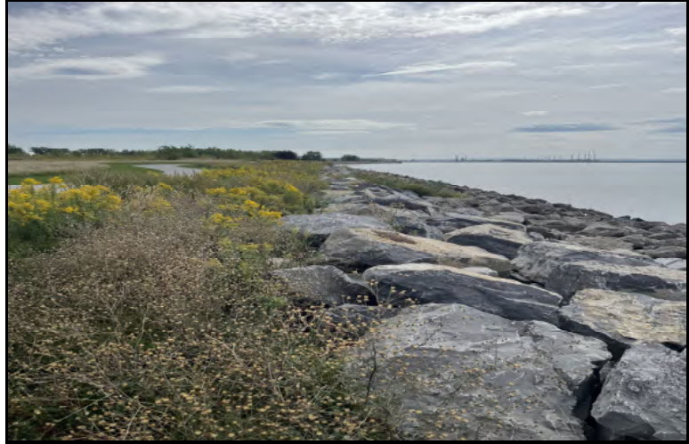
Photo 20: Stabilized shoreline and completed repairs
