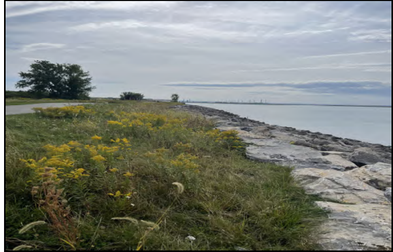
Photo 14: Stabilized shoreline and completed repairs
