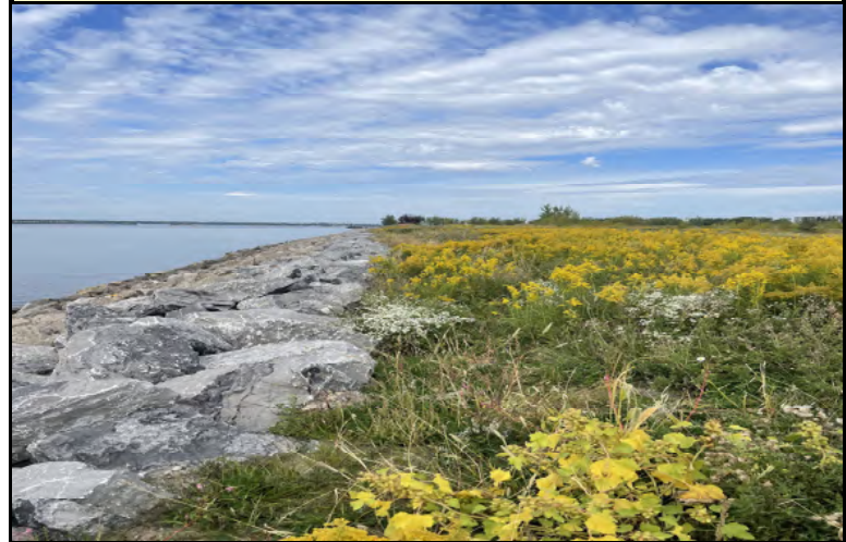
Photo 16: Stabilized shoreline and completed repairs
