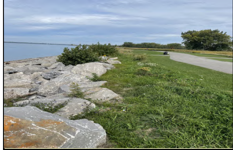
Photo 2: Stabilized shoreline and completed repairs
