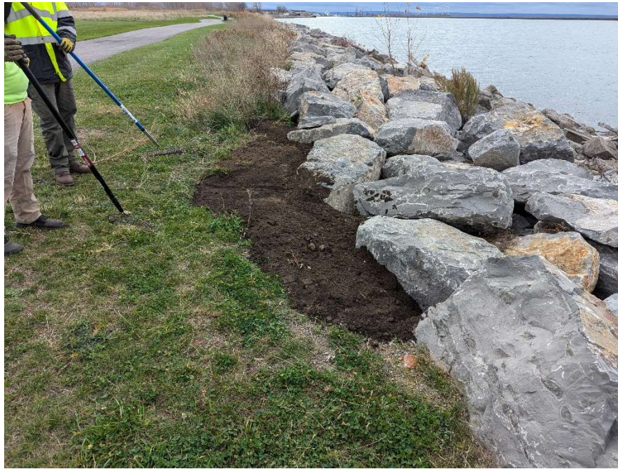
Photograph 3: Fill material spread out in the erosion area
