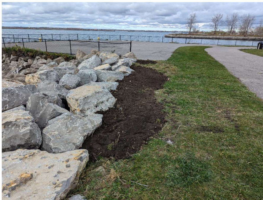
Photograph 2: Fill material placed in erosion area
