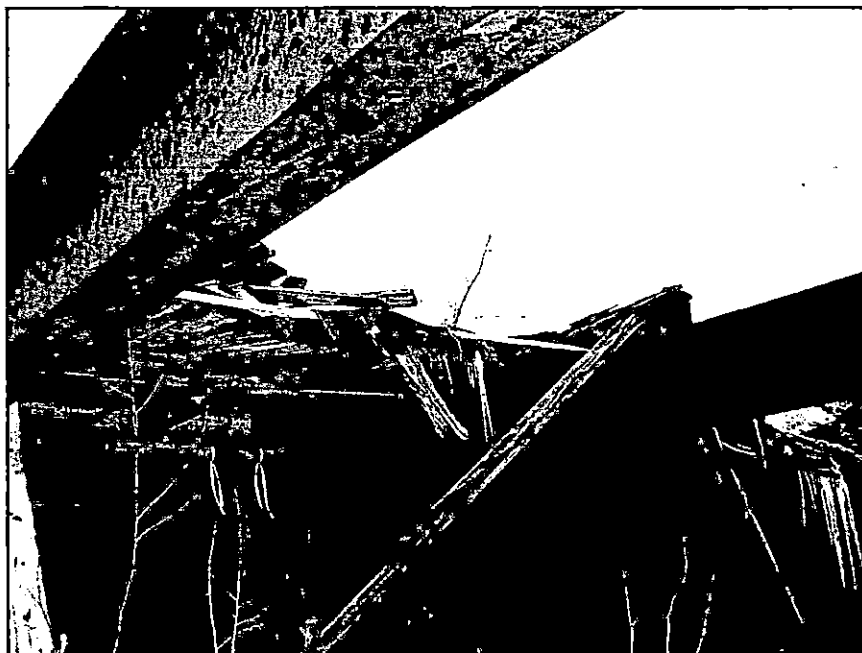
Building A Collapsed Roof Section
