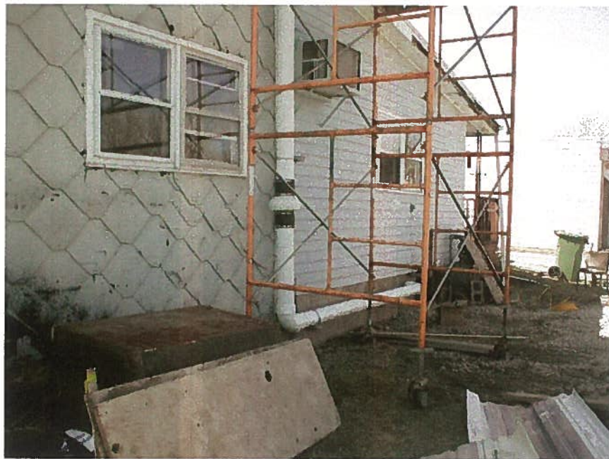
Aboveground exterior SSDS vent piping and in-line fan on north wall of building
