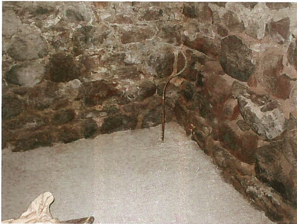
SSDS Vacuum Monitoring Point No. 2 located in eastern portion of basement
