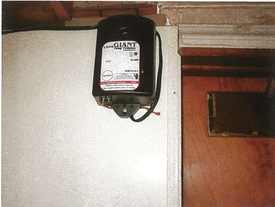
SSDS alarm in first-floor kitchen area
