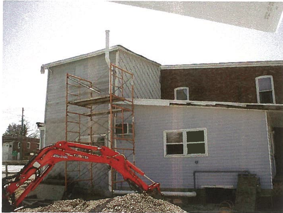
Aboveground exterior SSDS vent piping extending above roofline
