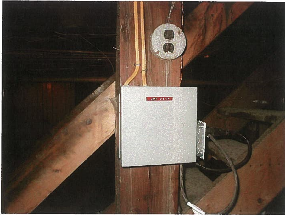
SSDS control box in basement
