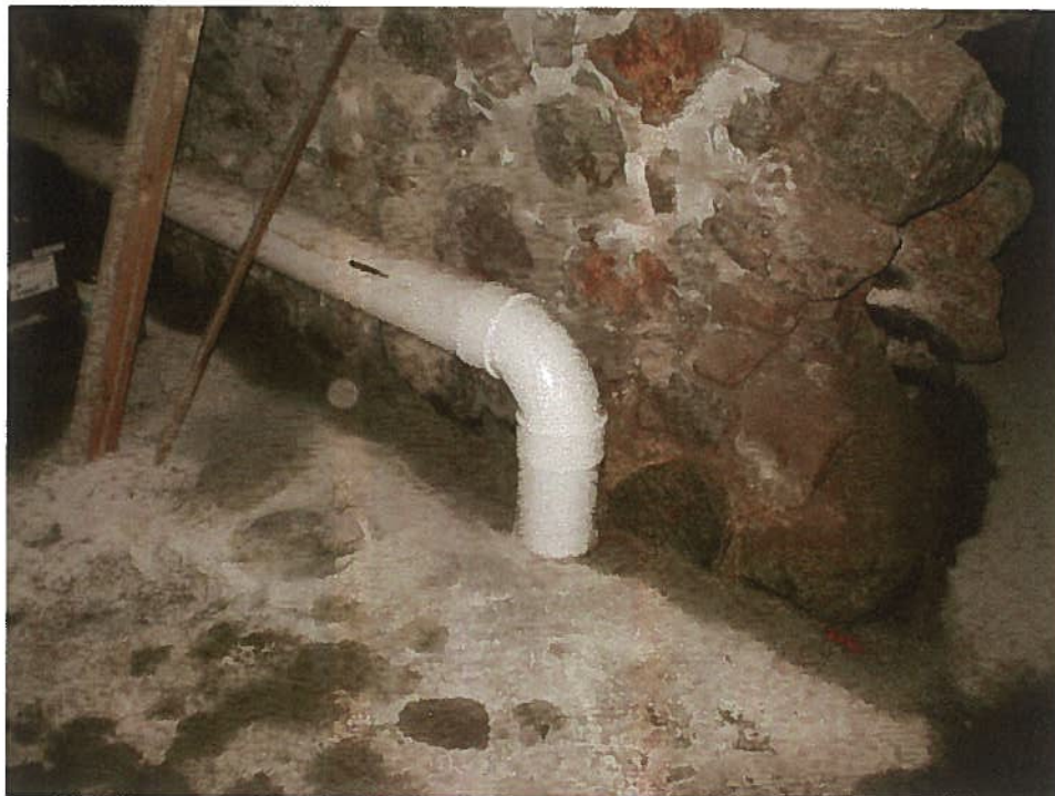
Aboveground SSDS vent piping connected to sub-slab perforated piping
