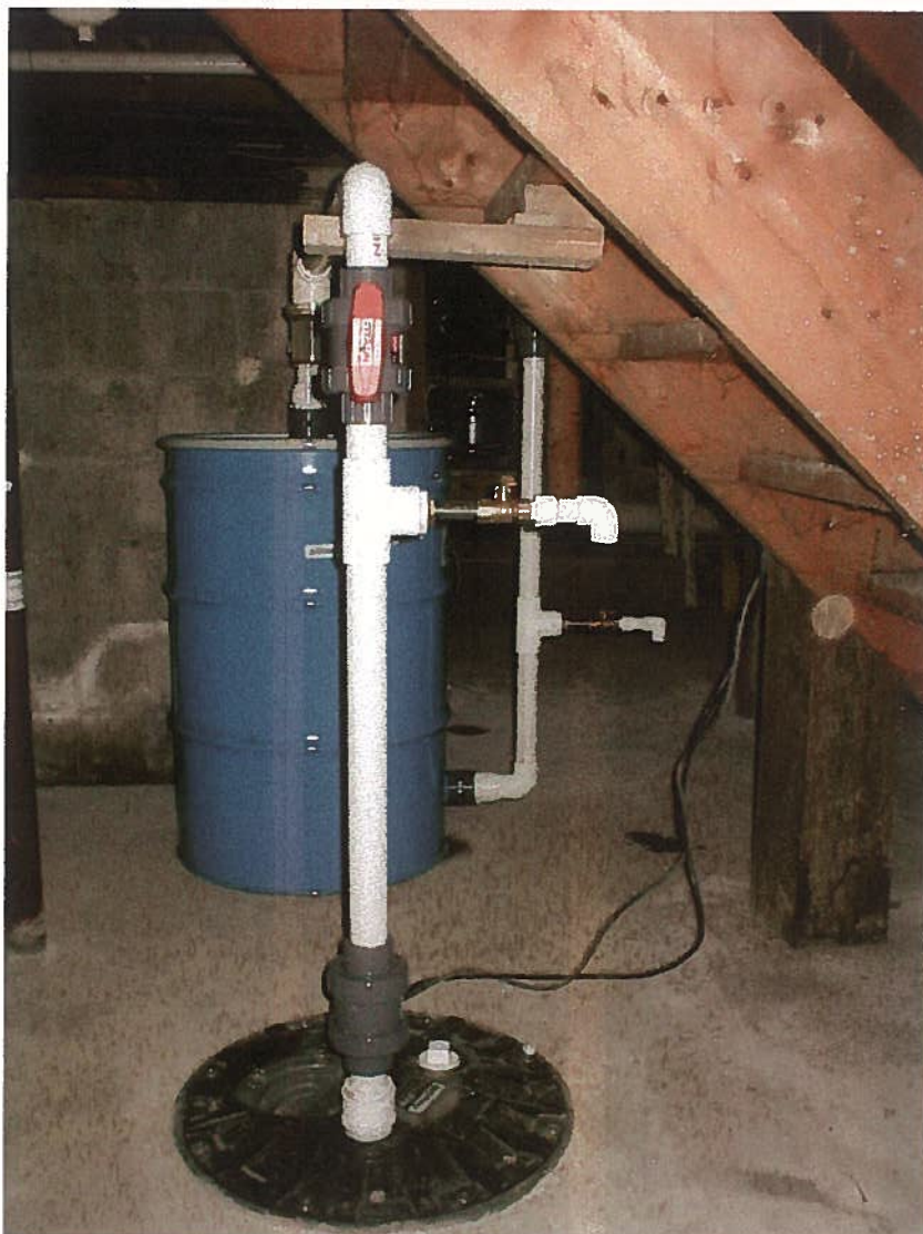
Basement sump with influent and effluent sample ports on each side of carbon filter drum
