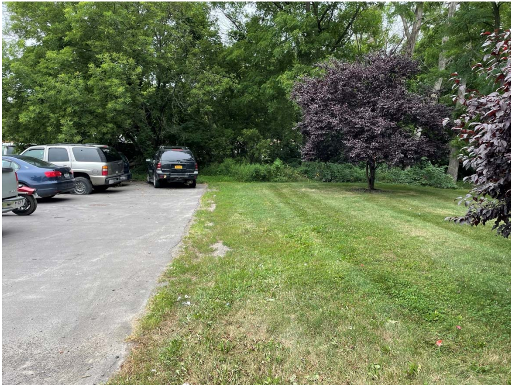
Asphalt pavement and earthen cover system – looking west
