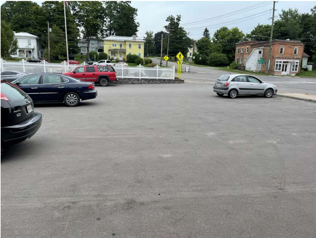
Asphalt pavement cover system – looking east
