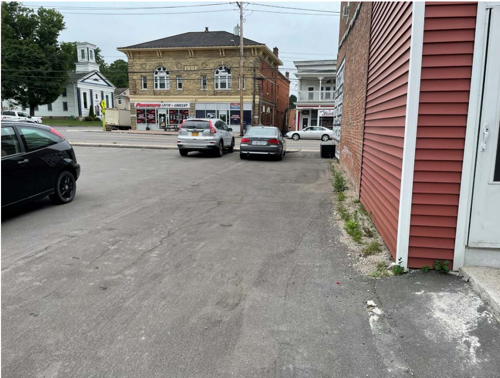
Asphalt pavement cover system – looking south
