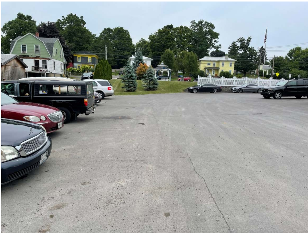
Asphalt pavement cover system – looking east
