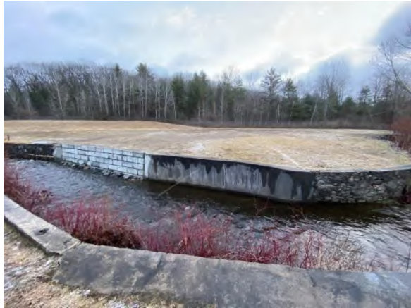
Southern wall repair area (2023) looking east Photographed December 2023
