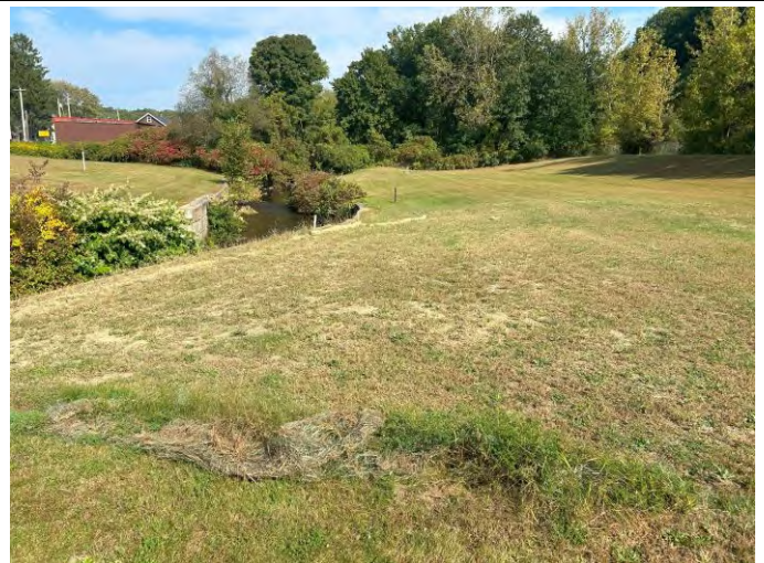
Repaired Site cover east of Cayadutta Creek
