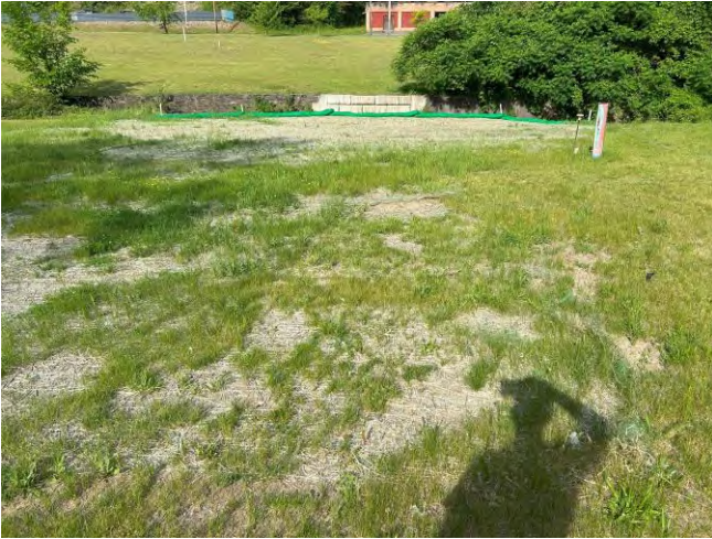
Northern wall repair area, showing erosion control matting and vegetation, looking northwest (Photographed June 2024)
