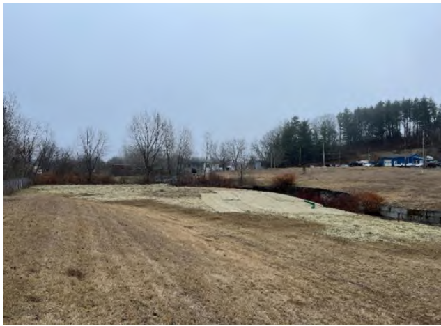
Eastern portion of the Site, looking south-southwest showing erosion control matting and mulch over imported topsoil Photographed December 2023
