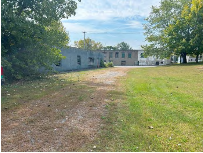
View of crushed stone driveway looking south towards Hill Street
