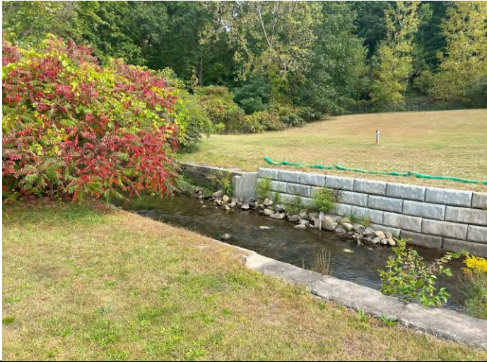
Repaired retaining wall, repaired animal burrows, and intact site cover at northern border of Site
