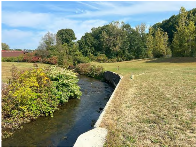
View of eastern retaining wall along Cayadutta Creek and repaired Site cover facing north
