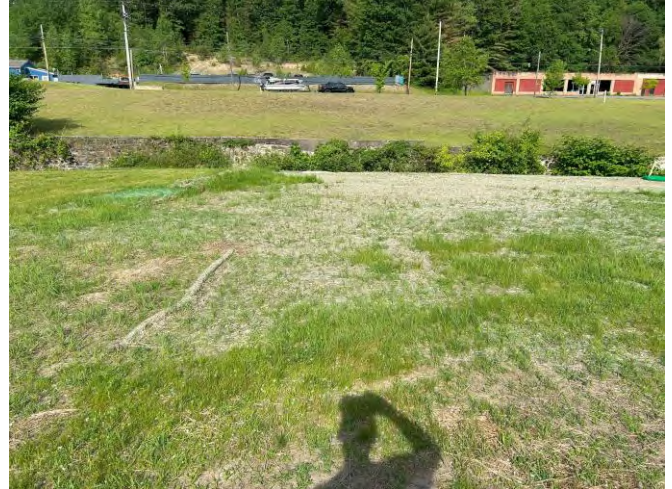
Southern wall repair area, showing erosion control matting and vegetation, looking west (Photographed June 2024)
