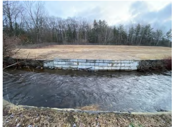
Northern wall repair area (2023 section left, 2019 section right) looking east Photographed December 2023
