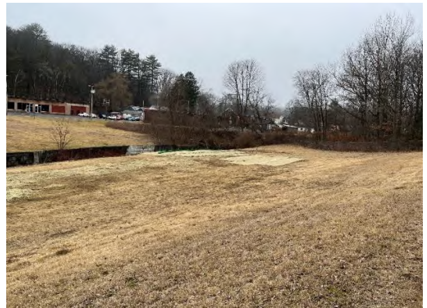
Eastern portion of the Site, looking northwest, showing erosion control matting and mulch over imported topsoil Photographed December 2023
