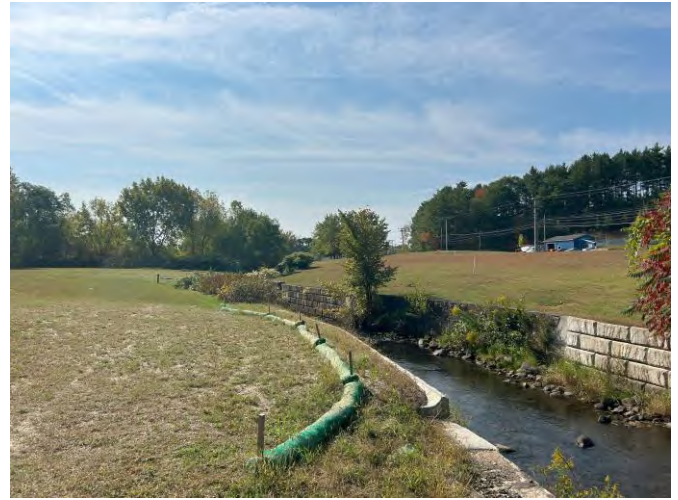
View of repaired Site cover facing southwest
