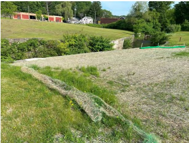
Southern wall repair area, erosion control matting and vegetation, looking north west (Photographed June 2024)
