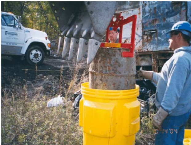
Overpack of the Excavated Drum
