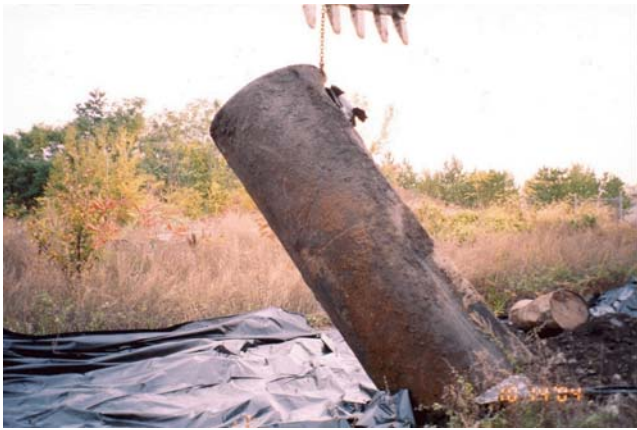
Excavation of the Buried Tank
