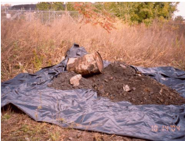
Temporary Staging of Contaminated Soil
