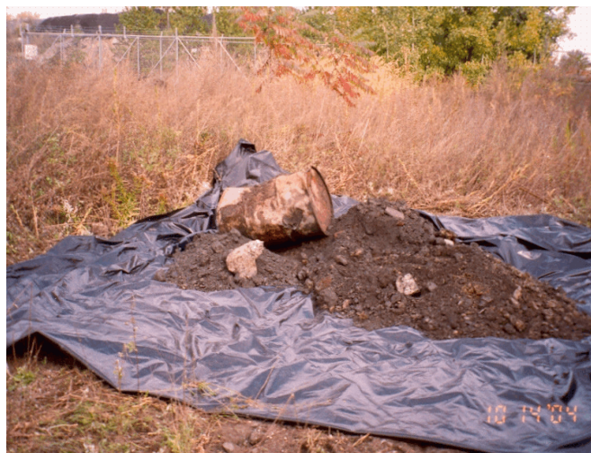
Temporary Staging of Contaminated Soil
