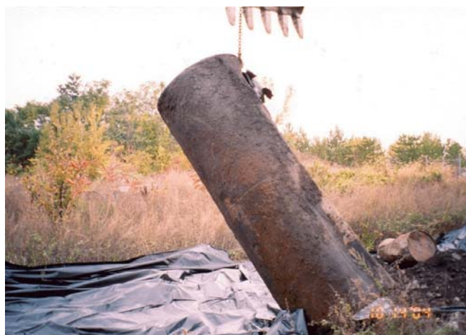
Excavation of the Buried Tank
