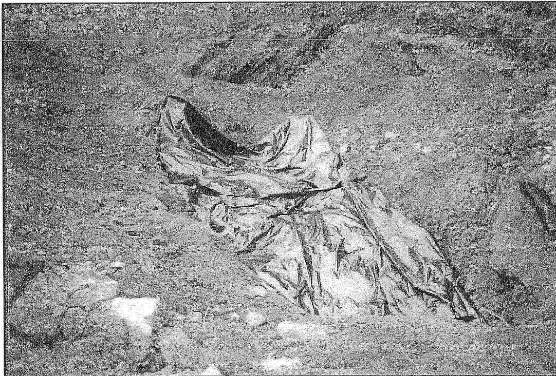
Black Poly Placed in Excavation Above Contaminated Soil
