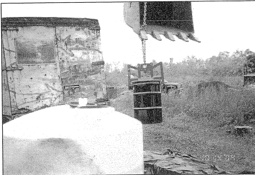
Drum Removed From Excavation to Holding Area
