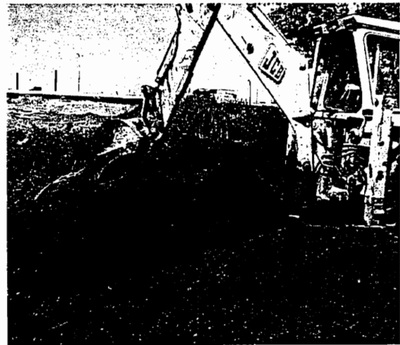
Figure 5: This is sample, US-FA-02 which is located on the canal side of the flu ash pile.
