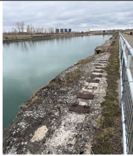
33. South side looking east at top of canal wall
