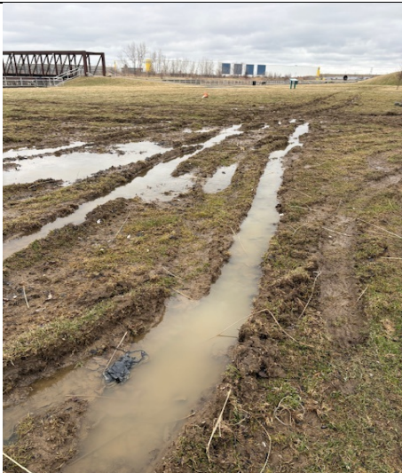
24. South side looking northeast at rutting
