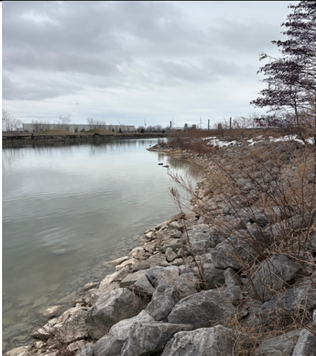
3. North side looking southwest at rock wall
