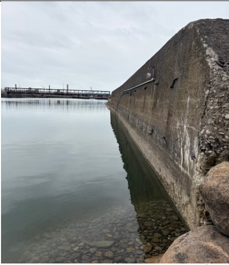
7. North side looking west at side of canal wall
