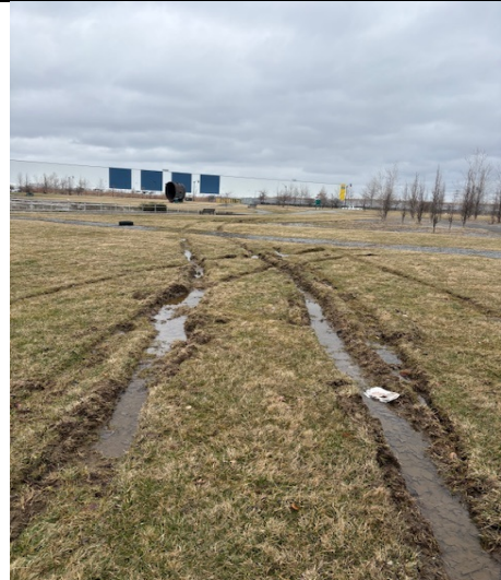
35. South side looking northeast at end of canal rutting
