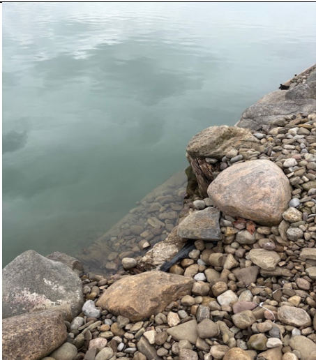
5. North side looking at beginning of canal wall
