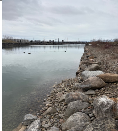
4. North side looking west at beginning of canal wall
