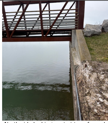
8. North side looking east at top of canal wall and bridge
