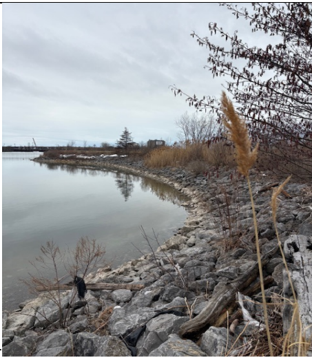
1. North side looking west at rock wall
