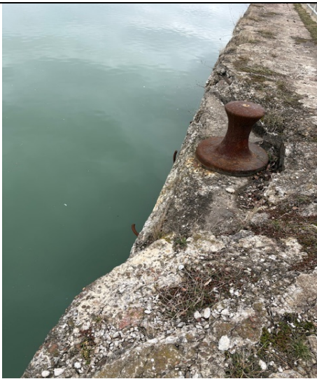
14. South side looking east at top of canal wall
