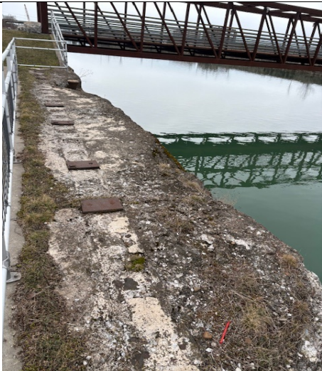
30. South side looking west at canal wall
