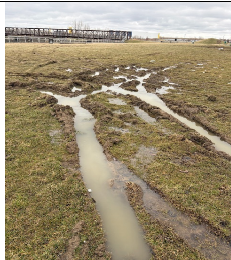
19. South side looking northeast at rutting
