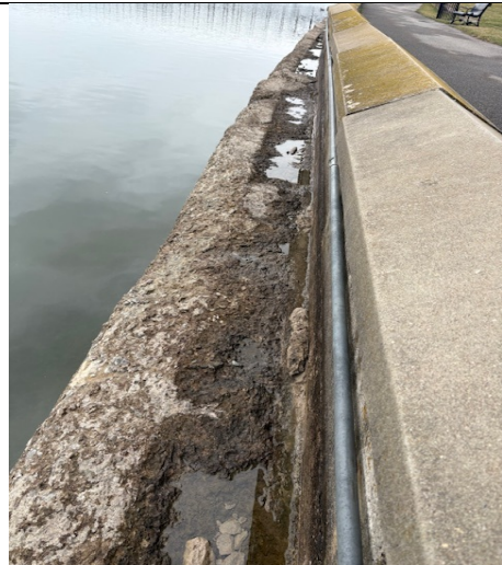
6. North side looking east at top of canal wall
