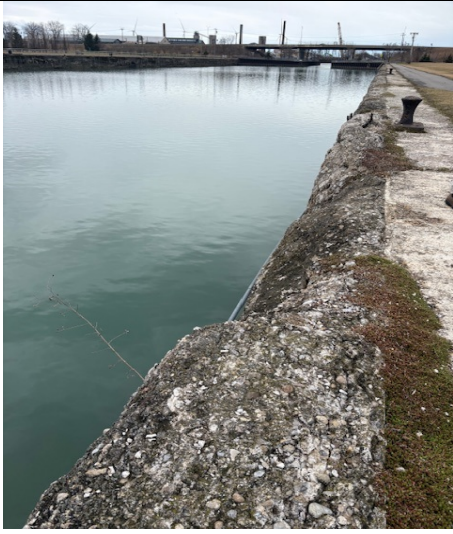
13. North side looking west at top of canal wall
