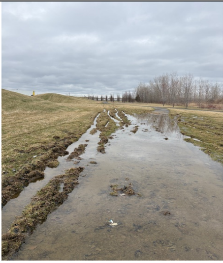
32. South side looking east at rutting
