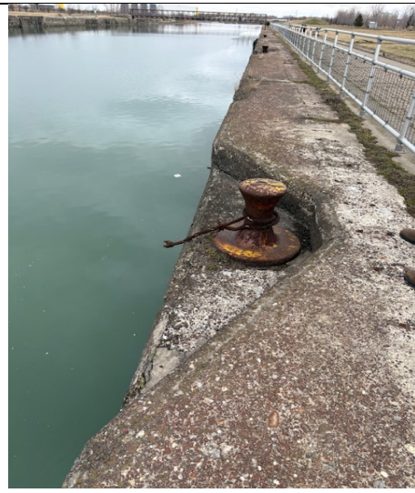
15. South side looking east at top of canal wall
