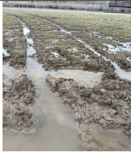
27. South side looking north at rutting
