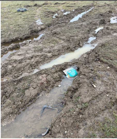
26. South side looking at significant rutting
