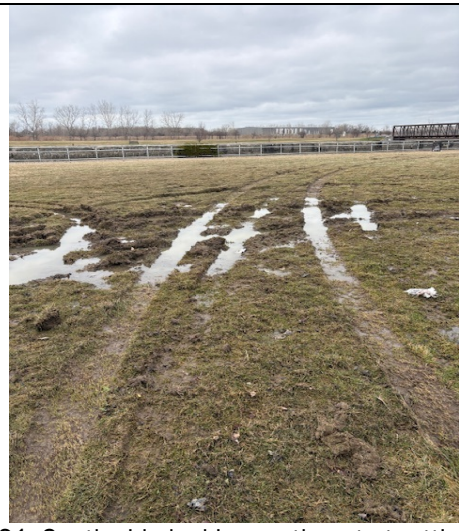
21. South side looking northeast at rutting
