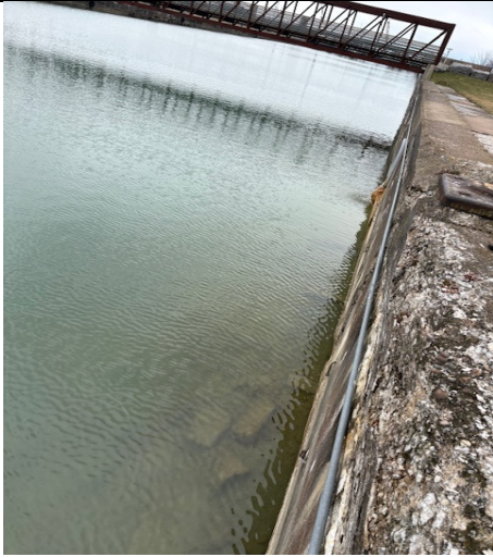
9. North side looking east at top of canal wall
