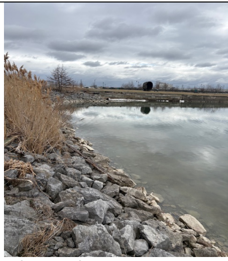
2. North Side looking east at rock wall
