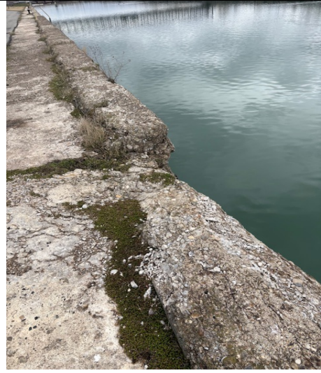
14. North side looking east at top of canal wall
