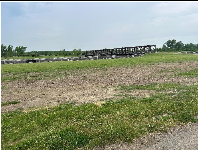
Southside repairs facing northeast
