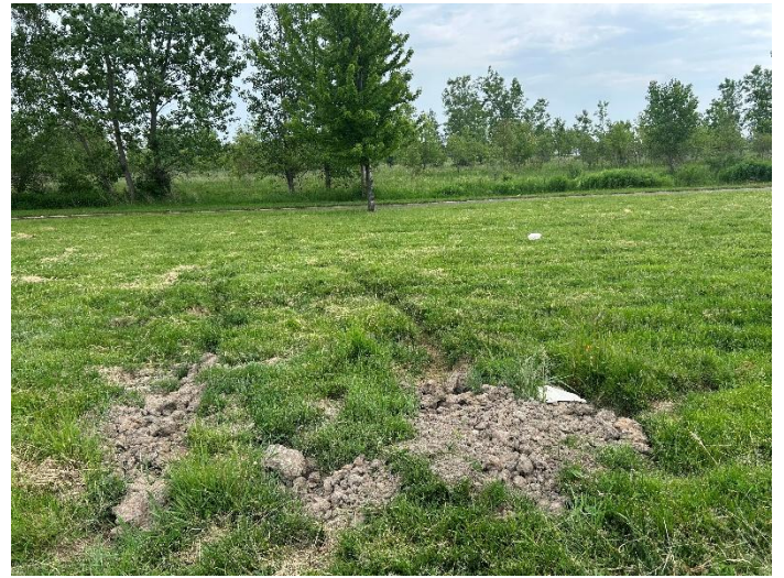
Southside repairs facing south off trail
