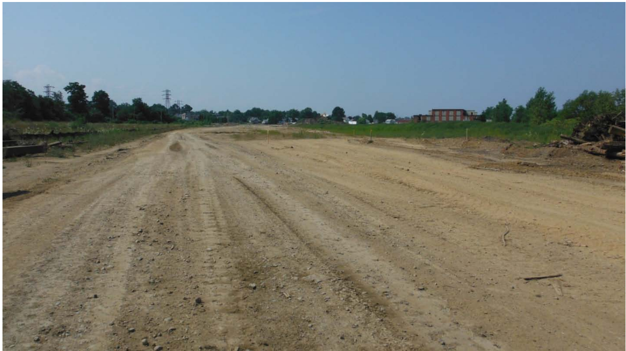
Photograph 4: Eastern portion of the site facing west
