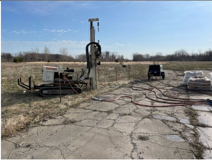
Typical injection set up around EX-MW-11R
