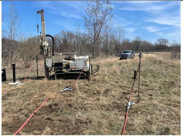
Typical injection set up around MW-07R
