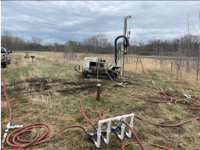
Typical injection set up around MW-07R
