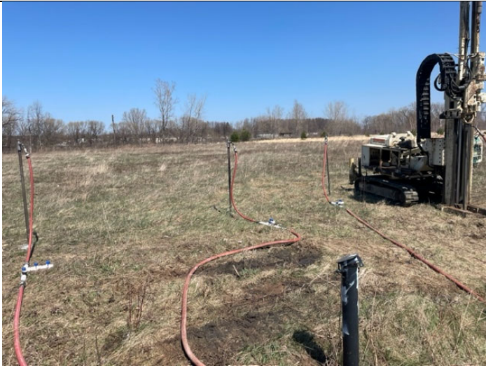
Typical injection set up around EX-MW-11R
