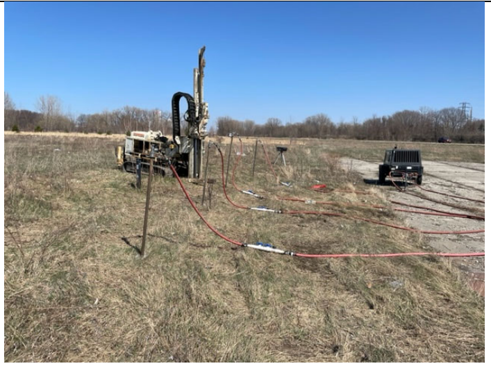
Typical injection set up around EX-MW-11R
