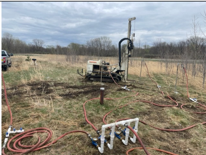
Typical injection set up around MW-07R
