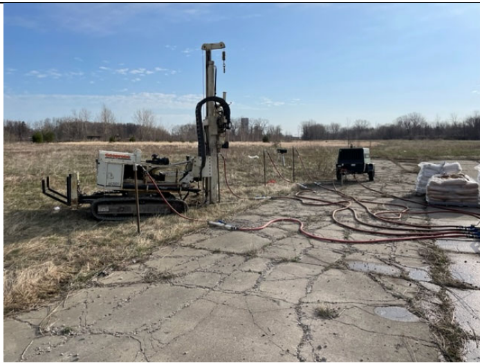
Typical injection set up around EX-MW-11R
