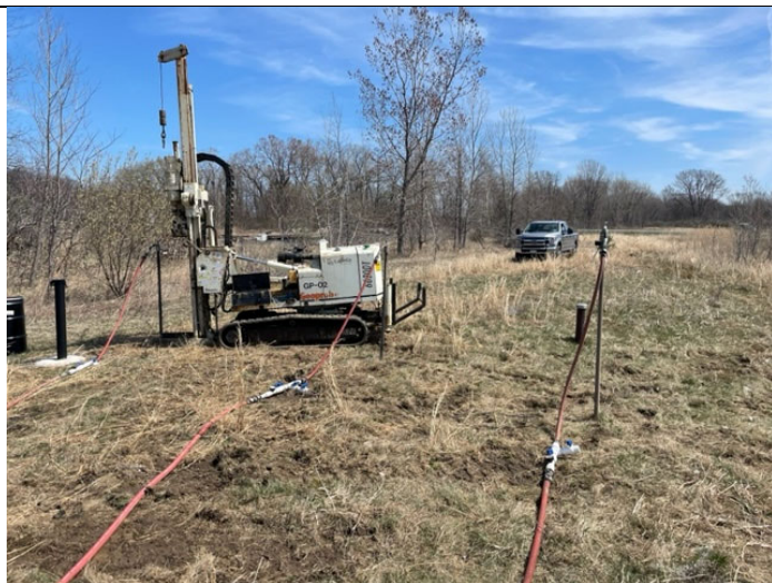
Typical injection set up around MW-07R
