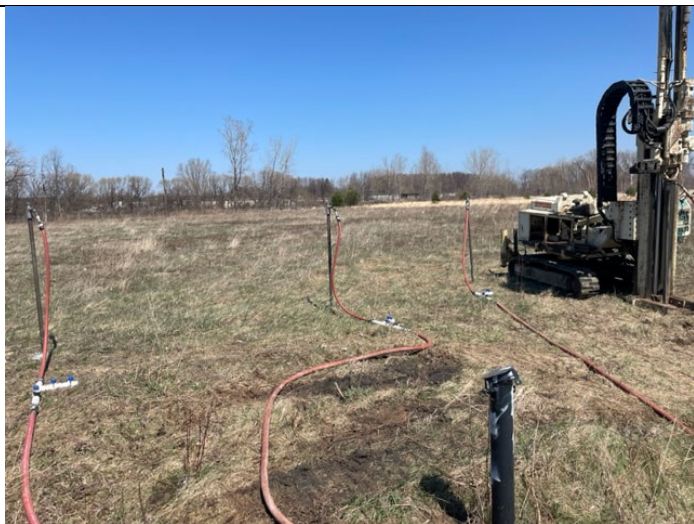
Typical injection set up around EX-MW-11R
