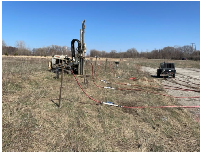
Typical injection set up around EX-MW-11R
