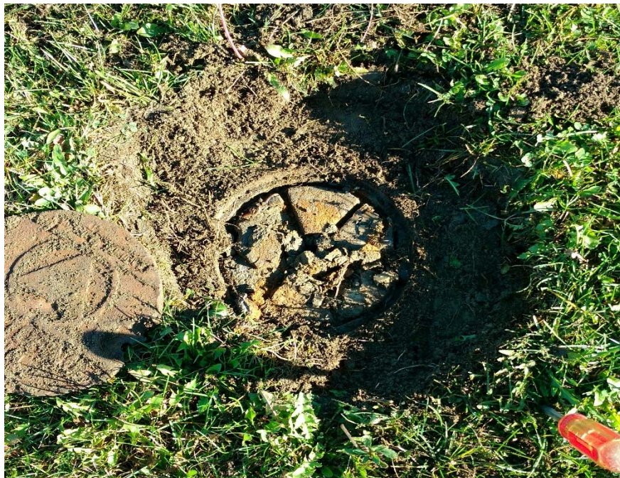
Monitoring Well MW-5 lid.
