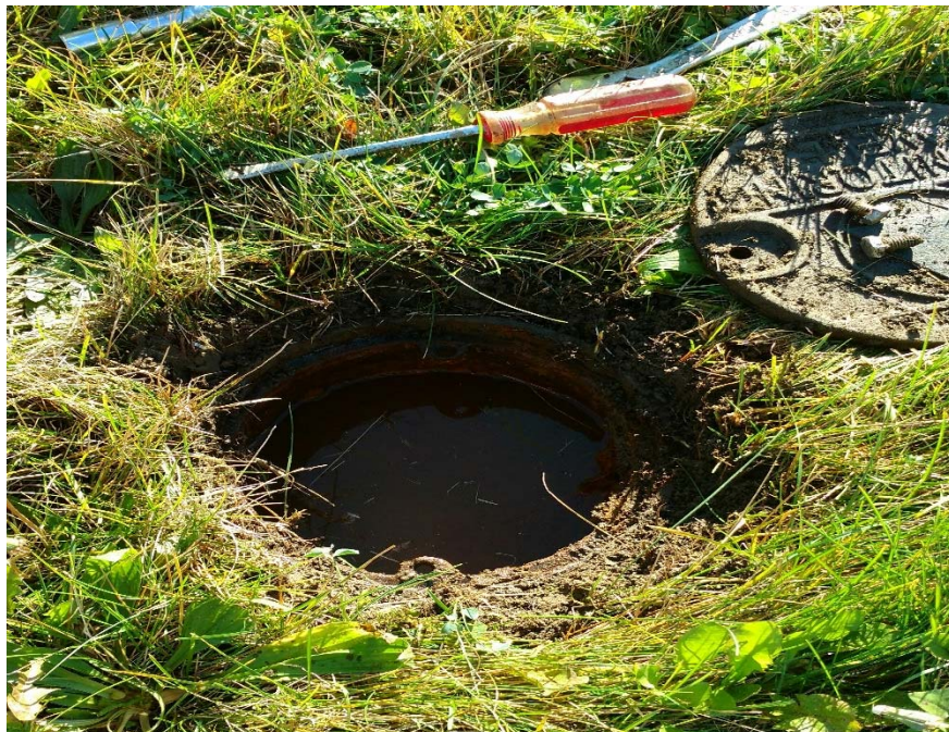
Monitoring Well MW-8 (water in curb box).
