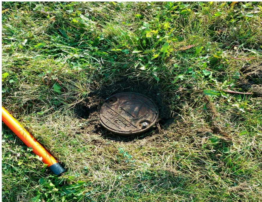
Monitoring Well MW-3.
