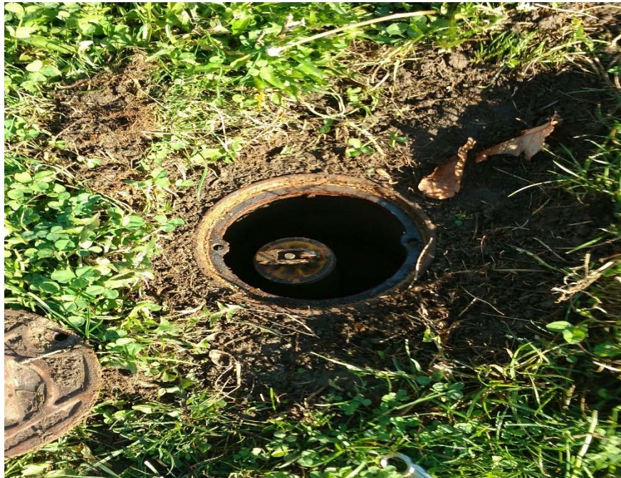
Monitoring Well MW-7.
