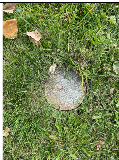
View of water interceptor trench lid
