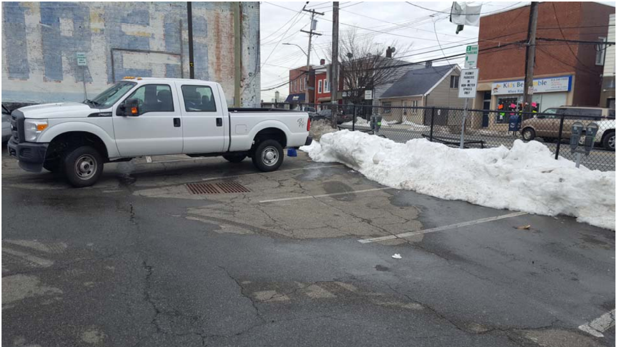
PHOTO 5: ASPHALT CAP (LOOKING WEST)
