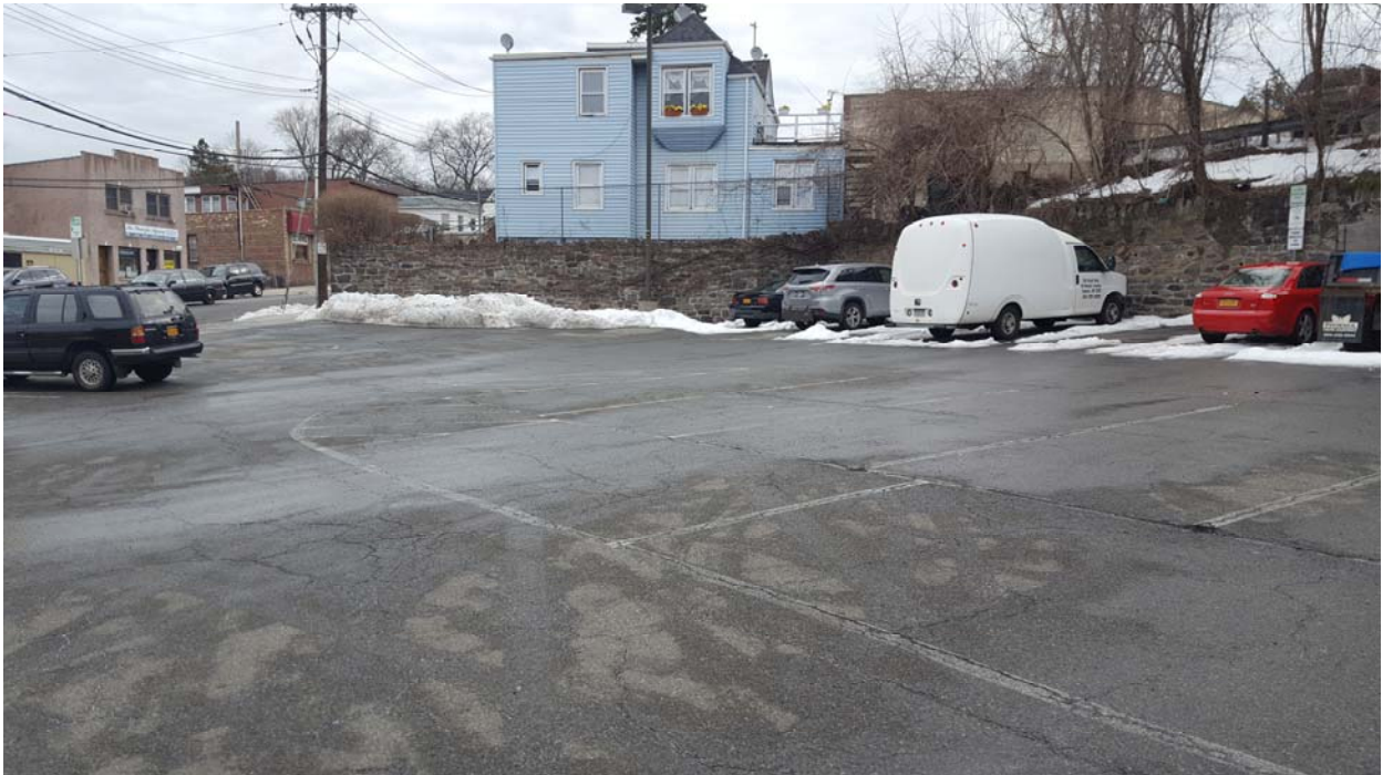
PHOTO 3: ASPHALT CAP (LOOKING EAST)
