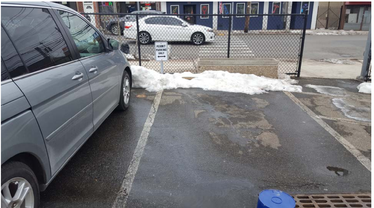
PHOTO 6: ASPHALT CAP (LOOKING WEST)
