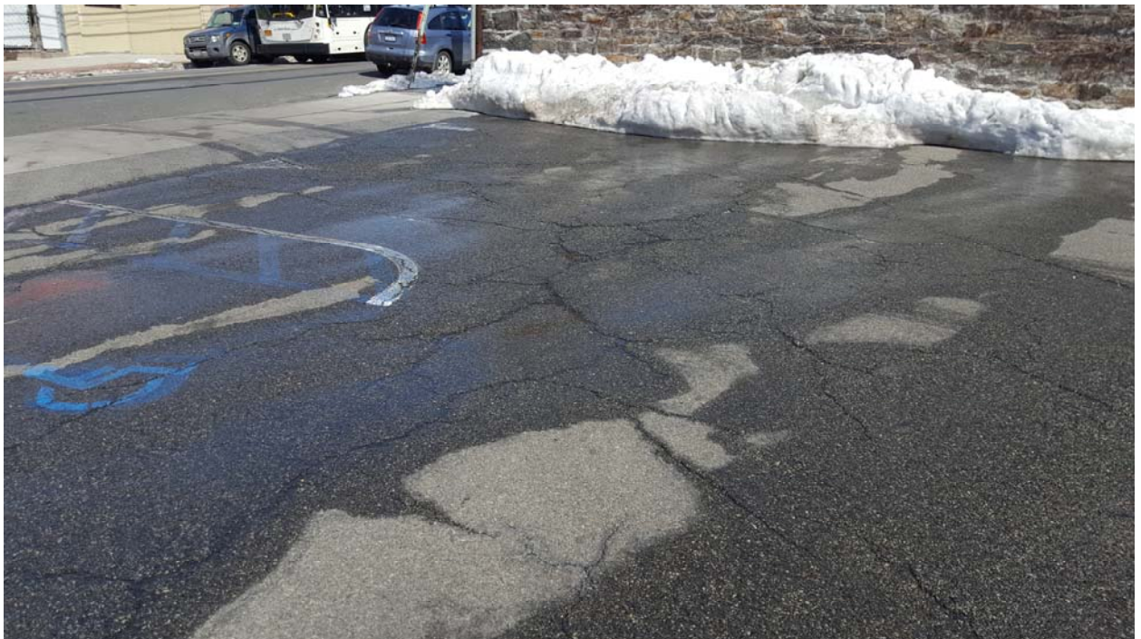
PHOTO 2: ASPHALT CAP (LOOKING NORTHEAST)
