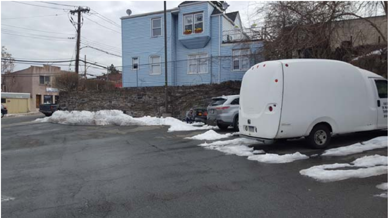
PHOTO 1: ASPHALT CAP (LOOKING NORTHEAST)
