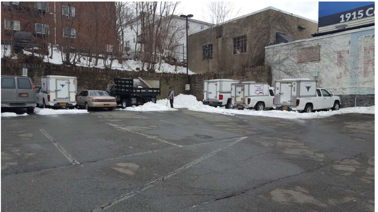
PHOTO 4: ASPHALT CAP (LOOKING SOUTHEAST)
